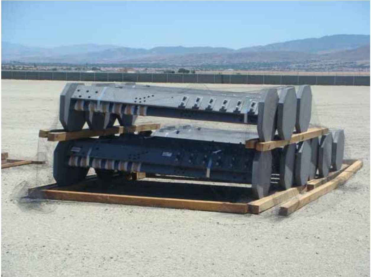
Figure 3: Bird-deterrent netting at Yard 28 used to discourage bird nesting in materials and equipment.
