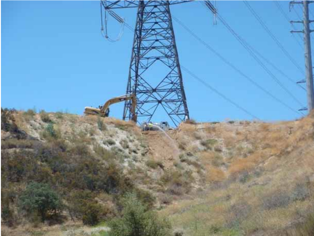
Figure 1: Erosion repairs underway at Tower 9 in Santa Clarita.
