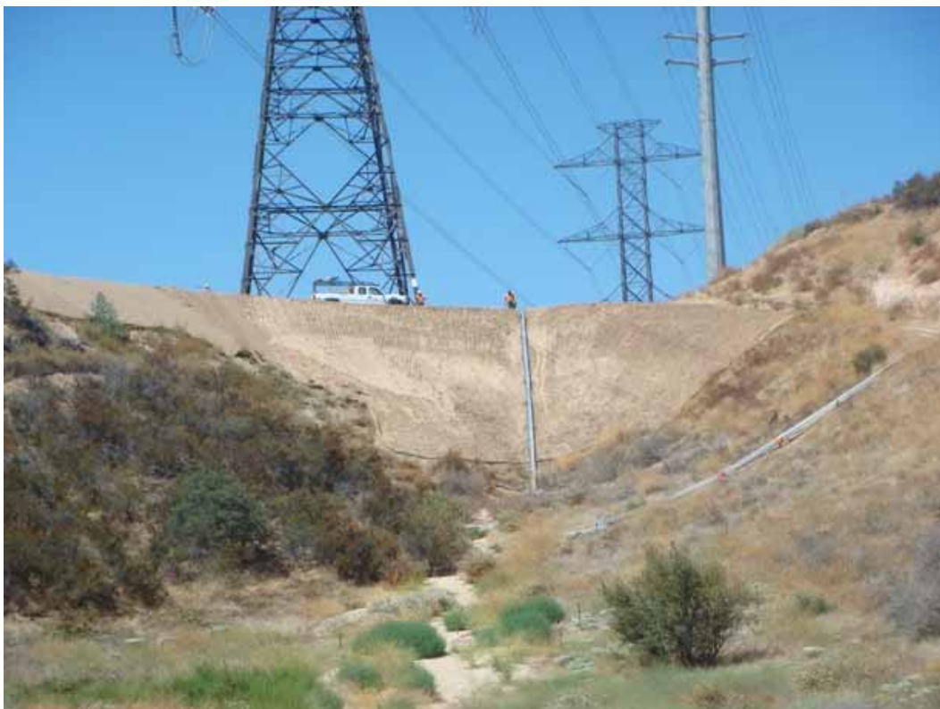
Figure 2: Completed erosion repairs at Tower 9 in Santa Clarita.
