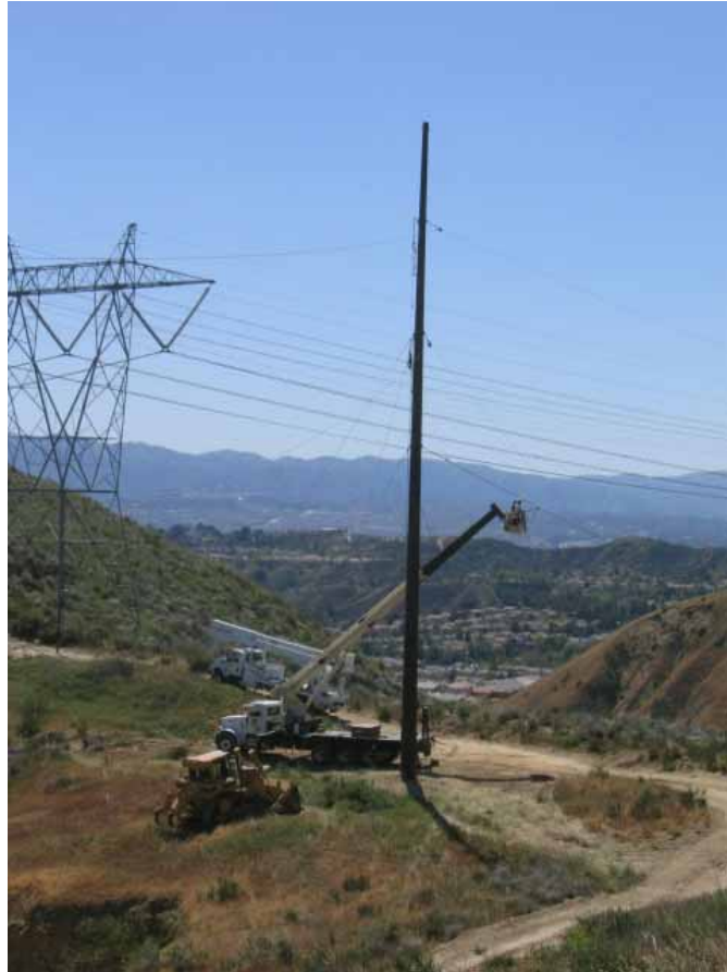
Figure 1: The installation of conductor wire between Shoofly poles 13-17 was completed using a helicopter. Once the sockline pulling cable was installed into each phase, the conductor wire was pulled back through the section and clipped in to each phase of the Shoofly pole.
