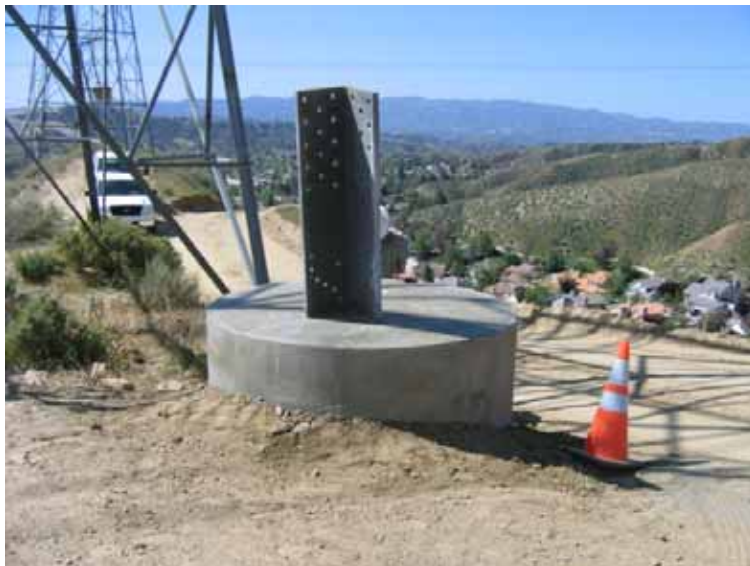
Figure 2: At 500 kV tower 25, crews completed drilling the foundations and pouring concrete.
