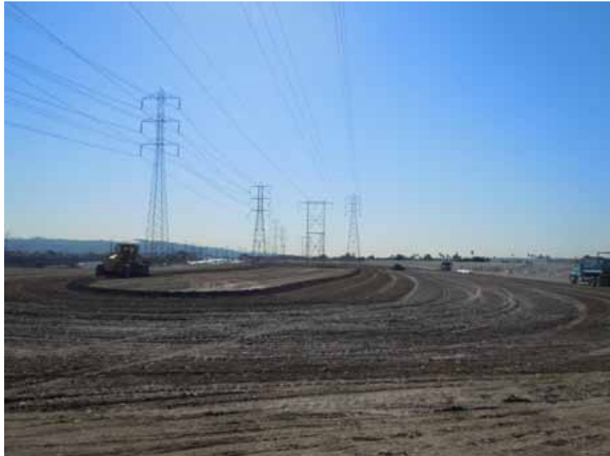
Figure 4: A DCX crew prepares Strawberry Field Contractor Yard in the City of Irwindale.
