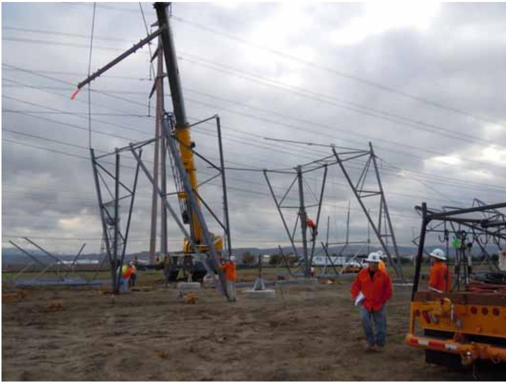
Figure 5: A Wilson crew assembles new Tower M0-T3, Segment 8, Phase 2.
