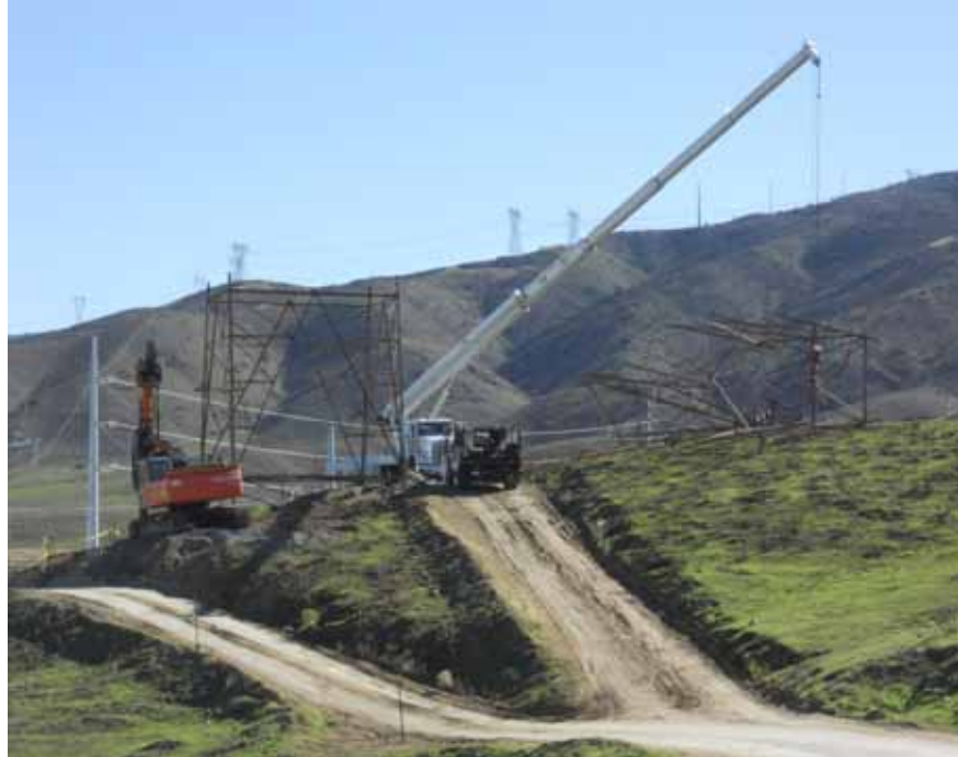
Figure 1: Wreck-out of existing 220 kV tower near new Tower 37 on Segment 5.
