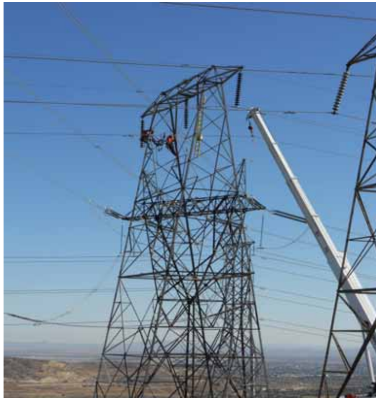
Figure 2: H&M wire crew unclipping wire and installing travelers on existing 220 kV tower on Segment 5.
