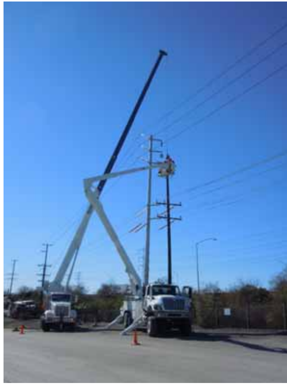
Figure 3: A Wilson crew sets a lightweight steel pole on the Rio Hondo–Amador-Jose-Mesa 66 kV line in the City of Irwindale.
