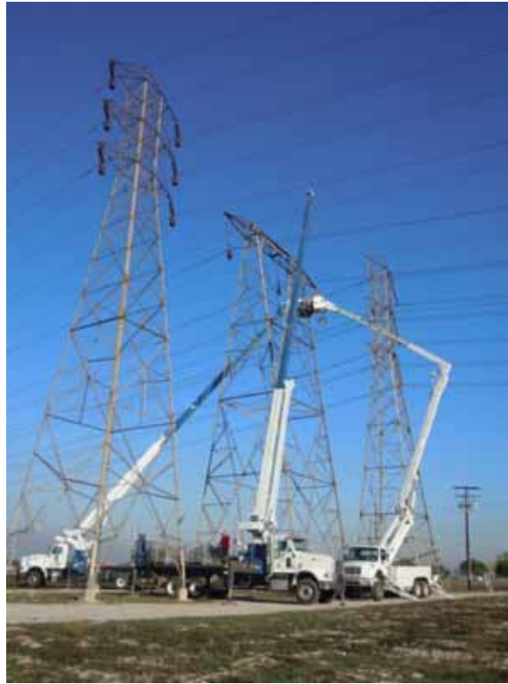
Figure 5: A Wilson crew removes wire from wreck-out towers, Segment 7.
