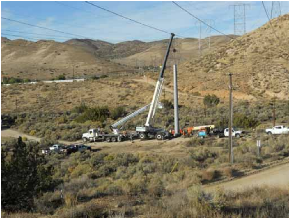
Figure 2: H&M crew installing TSP 5 outside the Vincent Substation, Segment 5.
