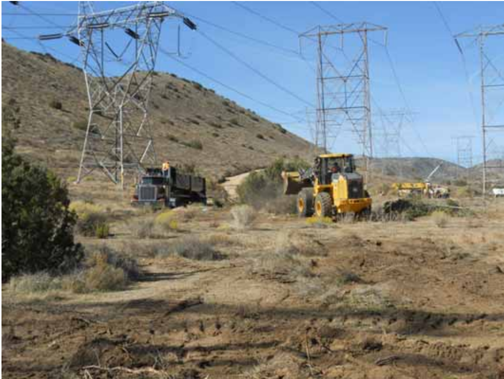
Figure 3: H&H Grading conducting juniper tree removal near Towers 63, Segment 5.
