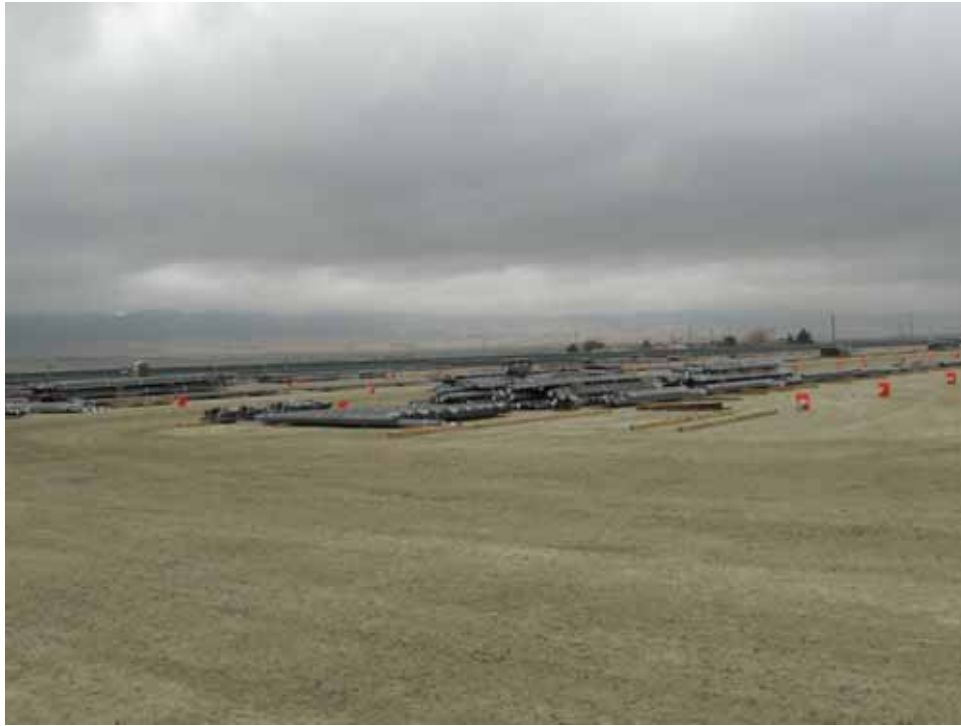
Figure 1: Materials stored in Material Yard 28, Segments 4, 5 & 10.
