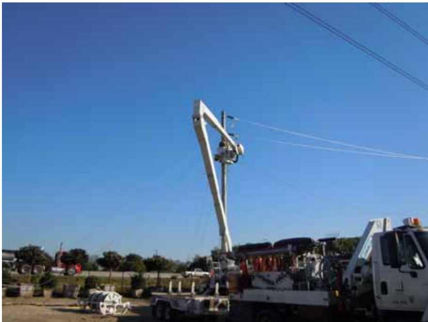
Figure 4: An SCE crew strings wire on the Rio Hondo–Amador-Jose-Mesa 66 kV line in the City of El Monte.
