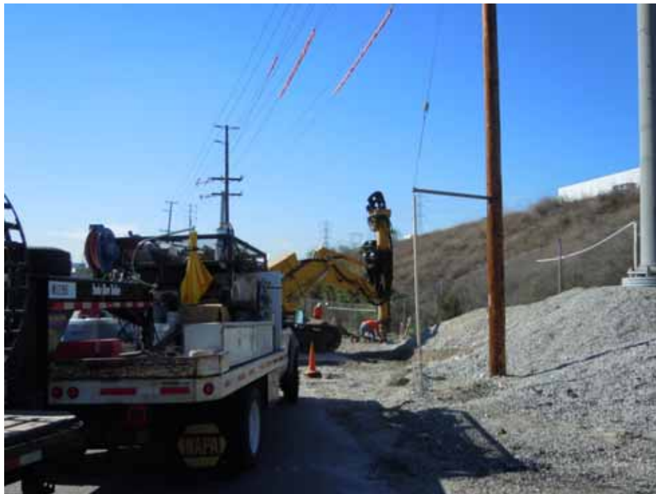
Figure 3: A Wilson crew drills a hole for a riser pole foundation, Segment 7 66 kV.
