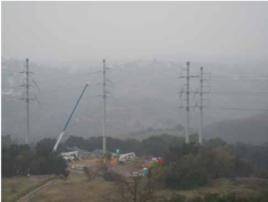
Figure 5: A Wilson crew assembles Tower M57-T3 in Tonner Canyon, Segment 8, Phase 1.
