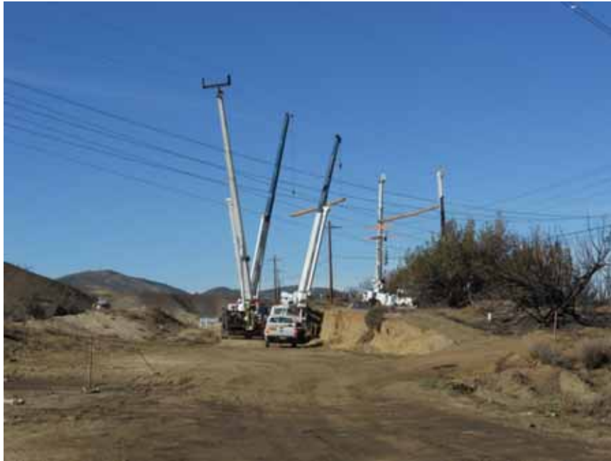
Figure 1: Boom trucks parked in guard pole sites for wire removal across Elizabeth Lake Road, Segment 5.
