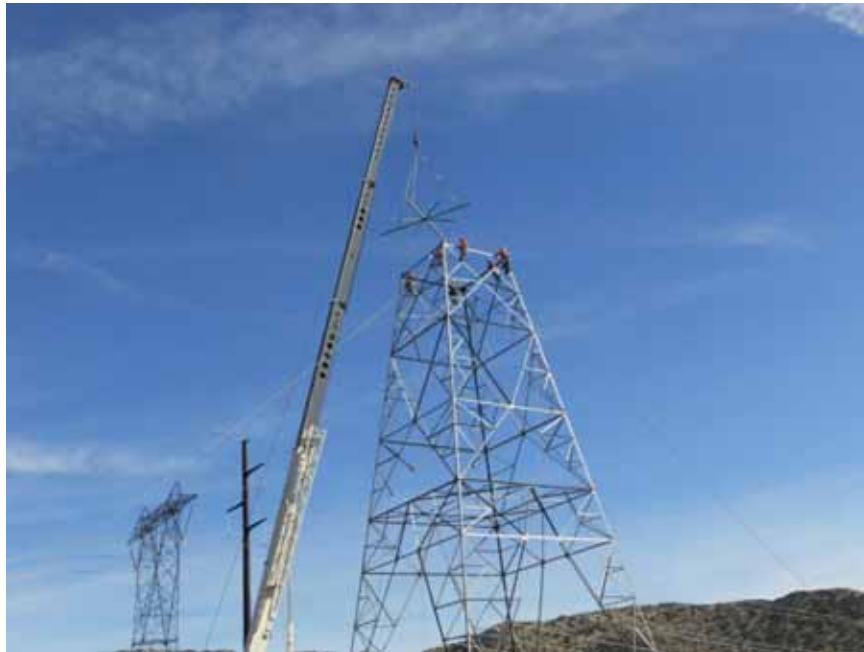
Figure 2: Assembly of new 500 kV Tower 57A, Segment 5.
