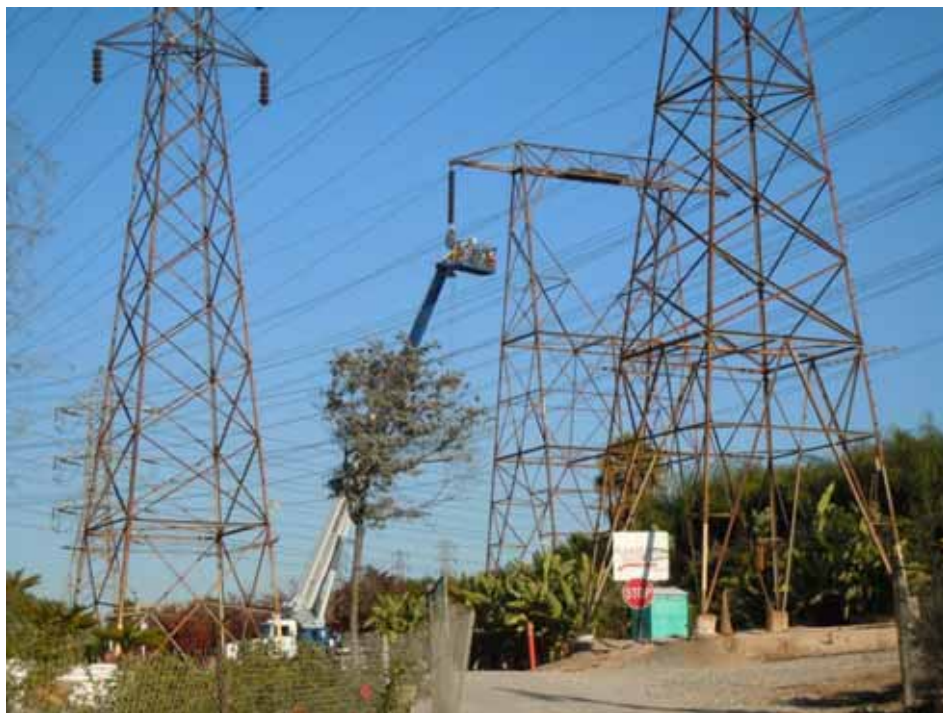
Figure 4: A Wilson crew removes wire, City of Montebello Hills, Segment 7.
