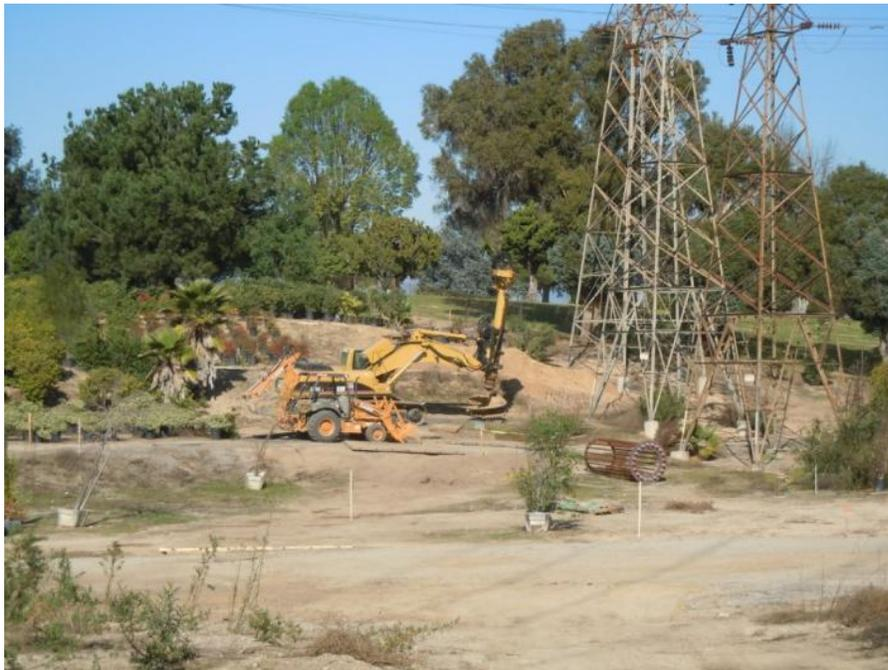
**Figure 4:** Crews drill a foundation for a TSP, Segment 7 66 kV near the Mesa Substation.
