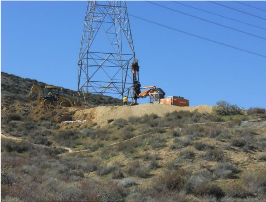
**Figure 1:** Woodward Brothers drilling foundation for Tower 17, Segment 5.
