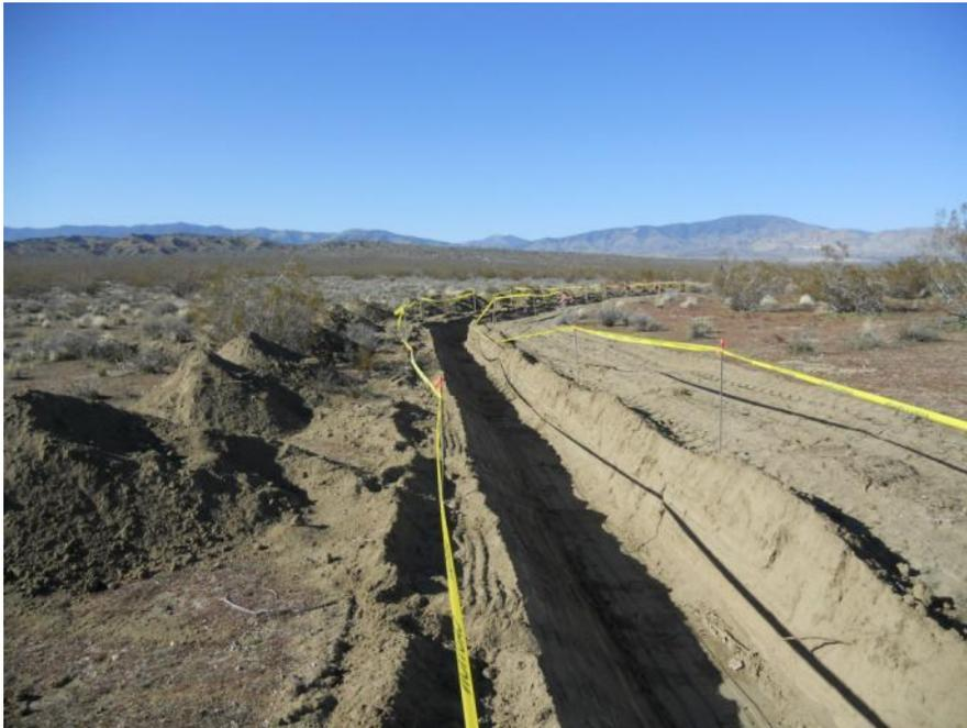
**Figure 2:** Tortoise fence trench along perimeter of Whirlwind Substation, Segment 9.
