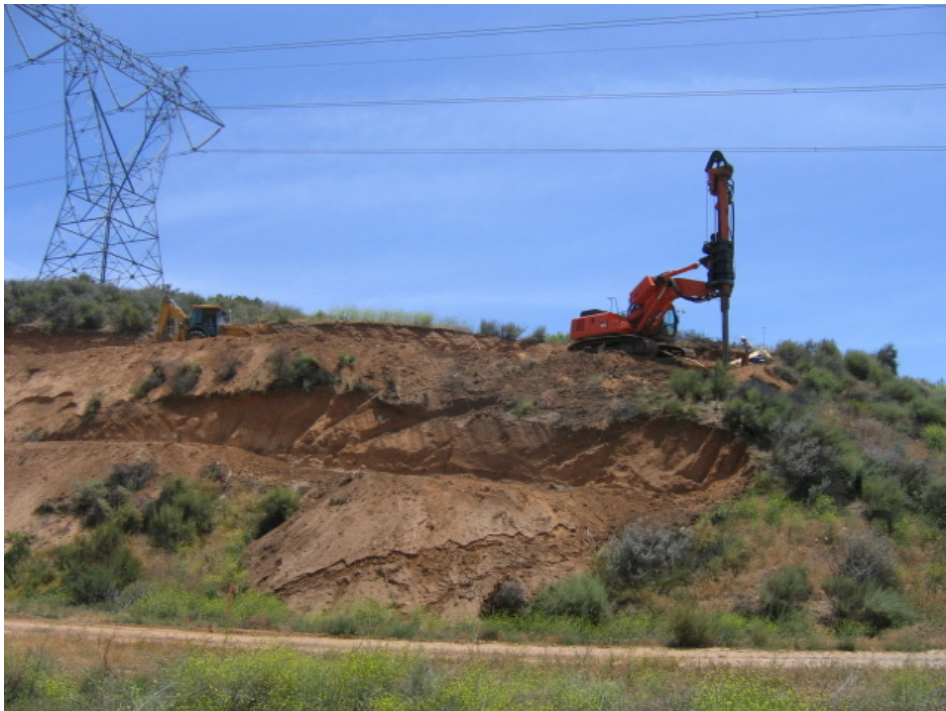
Figure 2: An auger truck excavating foundation footings at NC 3 after road building to the tower site took place.
