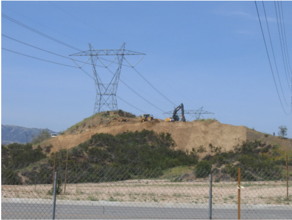
Figure 1: New tower pad construction at NC 4. Once the pad is constructed, the auger truck will be mobilized to drill the new tower foundations.
