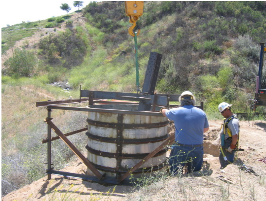
Figure 3: At NC 2, foundations were poured and steel anchors put in place to support the construction of the lattice towers.
