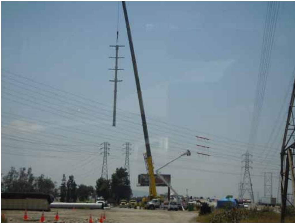
Figure 5: SCE crews set a riser pole on the underground Rio Hondo–Amador-Jose-Mesa line, Segment 7, 66 kV.
