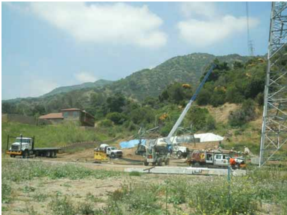
Figure 6: Crews assemble arms at Tower M27-T4, Segment 7 in Duarte.
