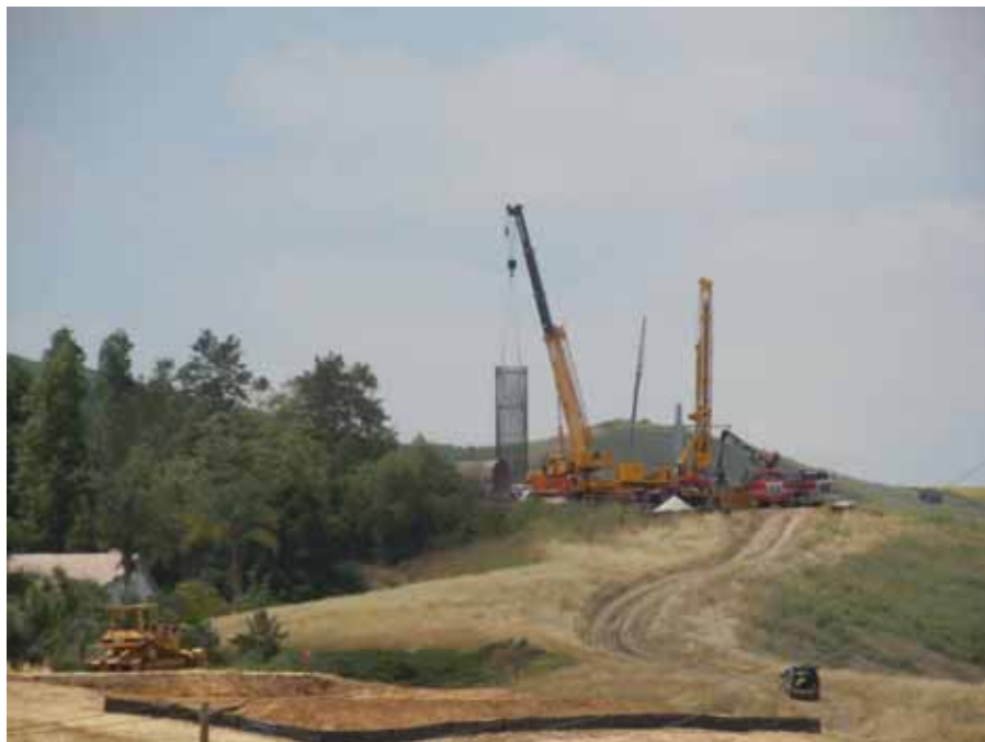
Figure 8: A Tri-State crew sets a rebar cage, Segment 8, Phase 1.
