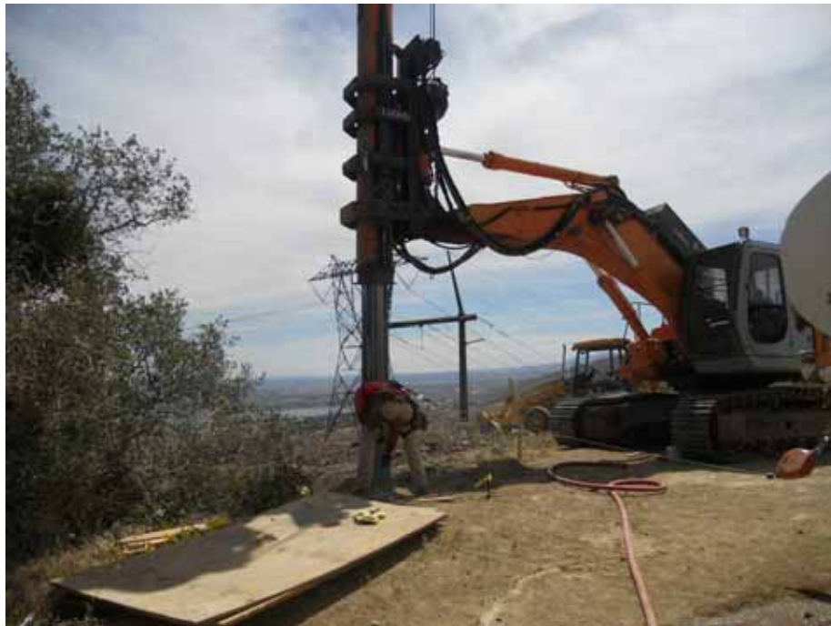
Figure 2: Woodward Brothers drilling foundations at Tower 49, Segment 5.
