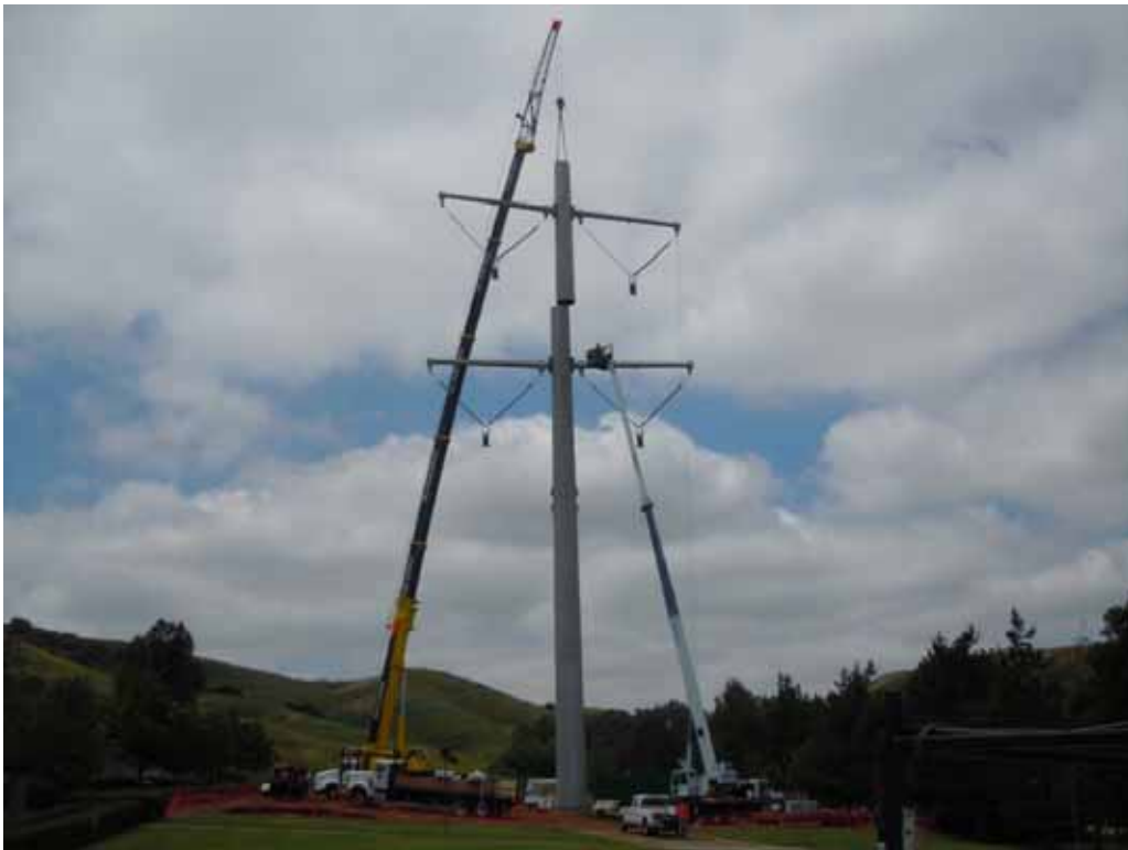
Figure 7: Crews set the mid-section of a tubular steel pole at Tower M61-T2, Segment 8, Phase 1 in Chino Hills.
