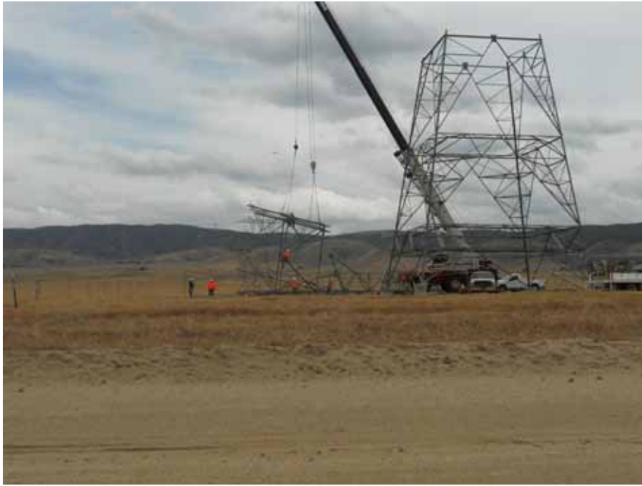
Figure 1: H&M steel crew assembling Tower 46, Segment 4.
