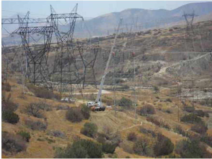
Figure 3: H&M wrecking-out 220 kV tower north of Elizabeth Lake Road, Segment 5.
