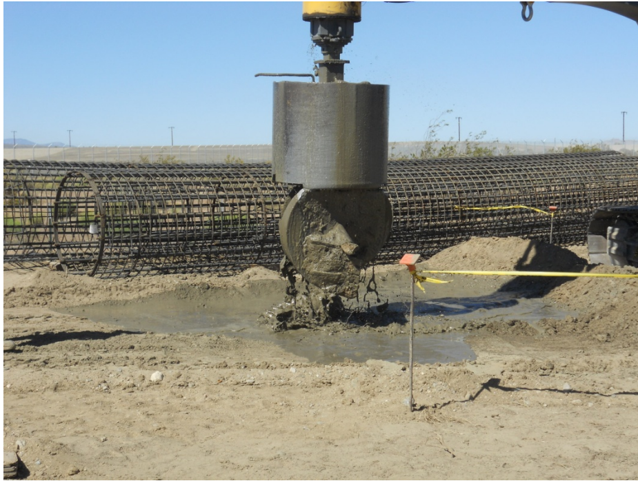
Figure 1: Drilling operation at Tower M74-T1X with the disposal of polymer, soil, and water mixture onsite, Segment 4.
