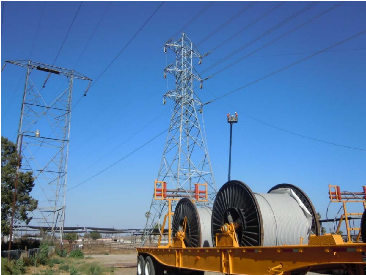
Figure 8: Crews string wire, Segment 8 Phase 2.
