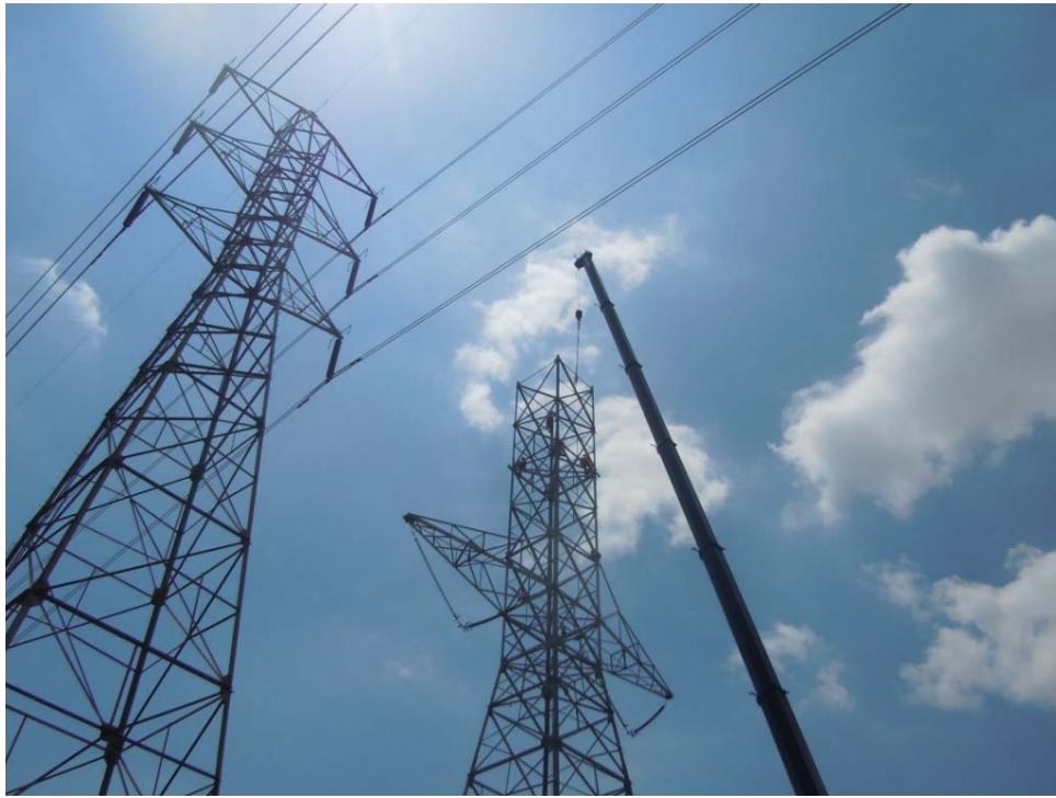
Figure 5: A Wilson crew assembles a tower, Segment 7
