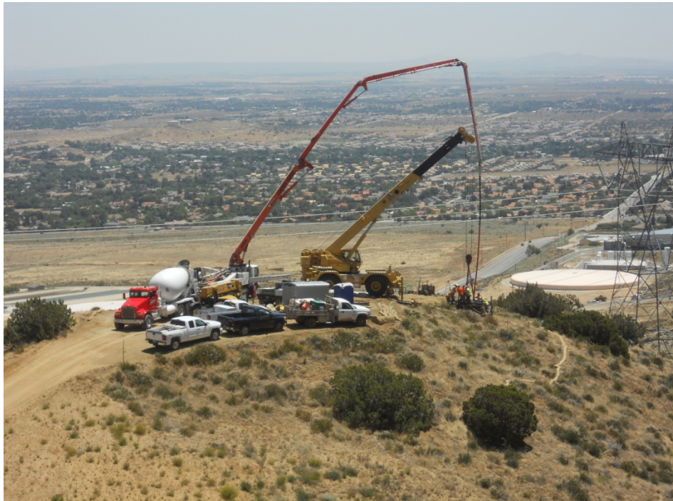
Figure 2: Woodward Brothers pouring concrete at Tower 18, Segment 5.
