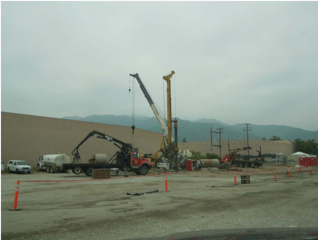
Figure 6: A Tri-State crew drills a foundation, Segment 7
