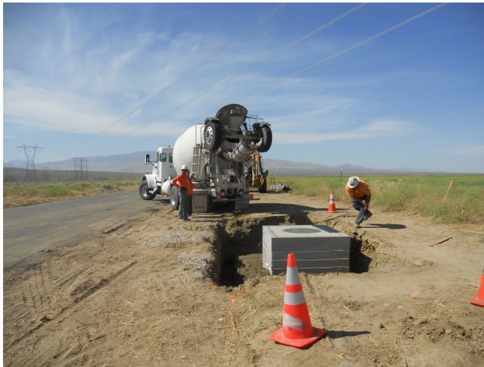
Figure 4: Tidwell pouring slurry around manhole on the east side of 170 th Street, Segment 10 Telecom.
