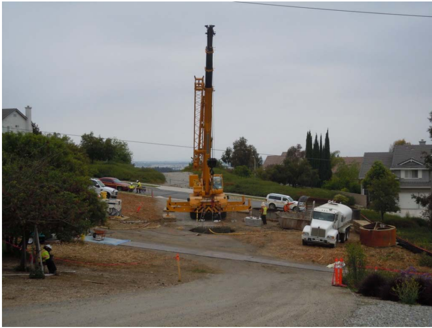
Figure 7: Crews drill a foundation for a TSP, Segment 8 Phase 1.
