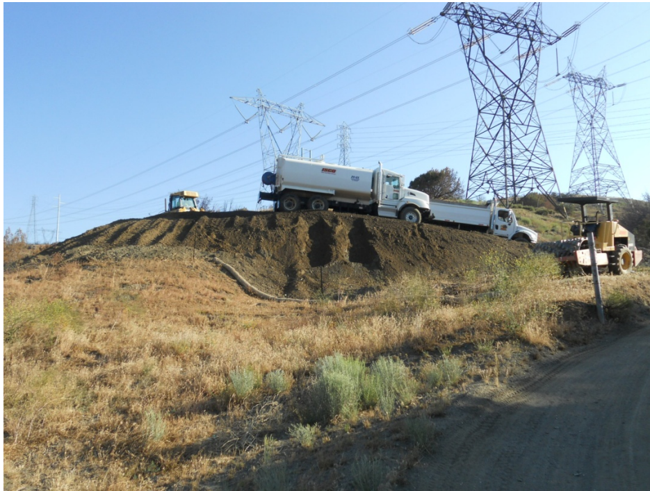
Figure 3: H&H Grading working on crane pad site at Tower 28A, Segment 5.
