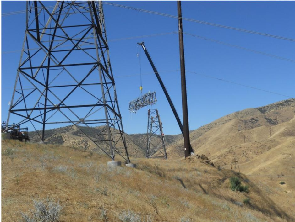
**Figure 1:** H&M steel crew erecting Tower 46, Segment 5.
