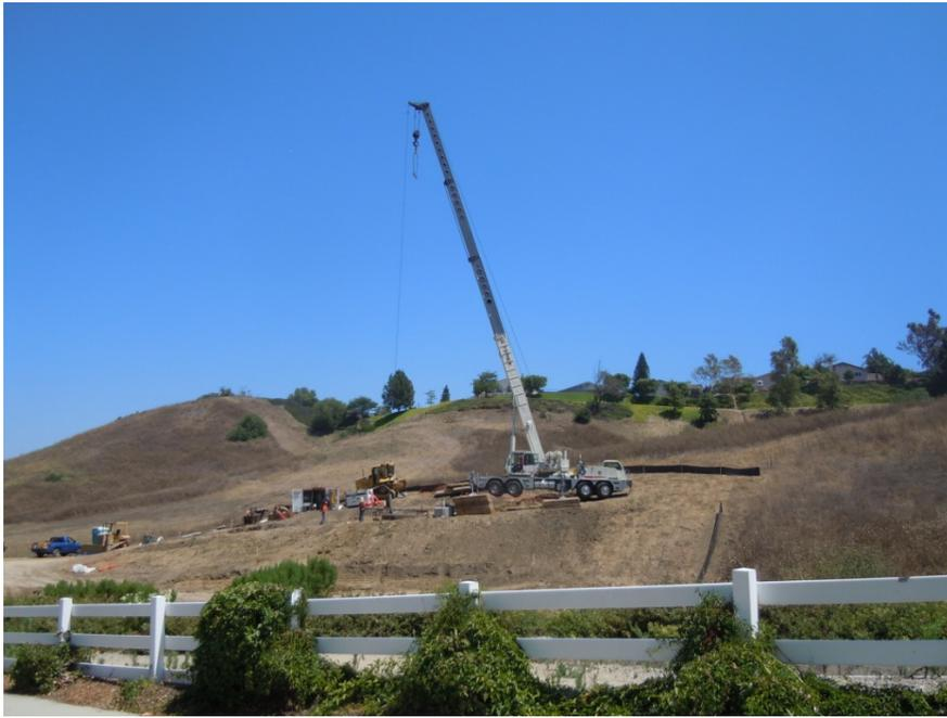
**Figure 5:** Tri-State drills a foundation for an LST in Chino Hills, Segment 8, Phase 1.
