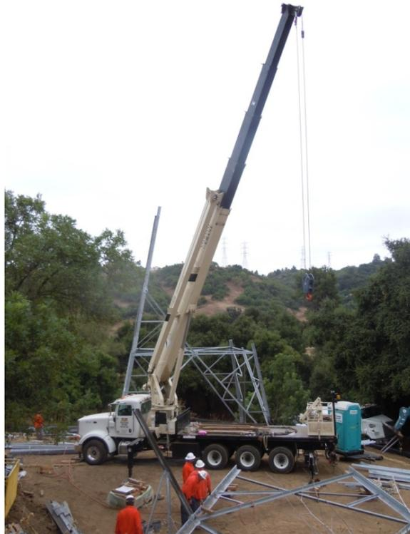
**Figure 6:** Crews assemble a tower within the PHLNHA, Segment 8, Phase 4.
