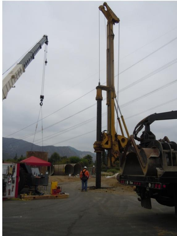
**Figure 4:** A Tri-State crew drills a foundation for a lattice steel tower (LST) in the City of Duarte, Segment 7.
