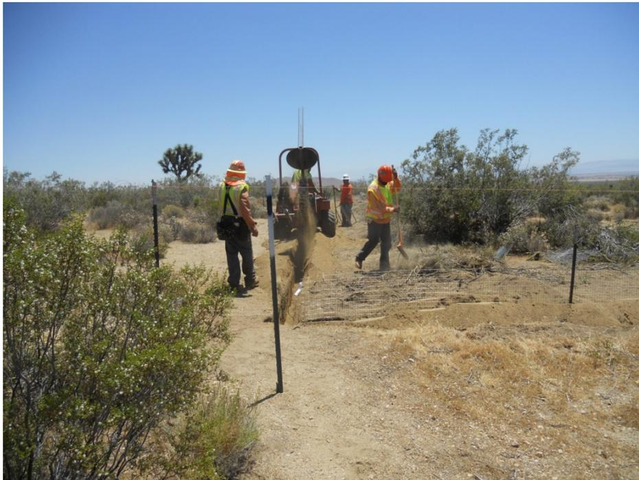
**Figure 2:** Moore Fence crew installing permanent tortoise fencing at Tower 52, Segment 10.
