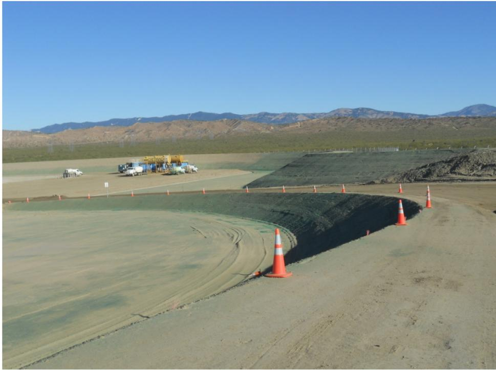
**Figure 3:** Tackifier (used for dust suppression) applied to channel berm inside Whirlwind Substation, Segment 9.
