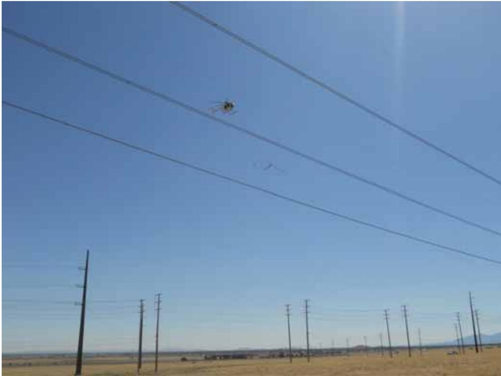
**Figure 3:** Helicopter flying the sockline that is attached to a needle which threads it through the travelers on the towers, Segment 5.
