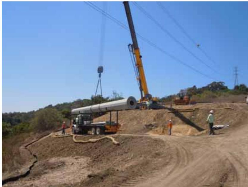
**Figure 8:** A Wilson crew sets an emergency steel pole, Segment 8, Phase 4.
