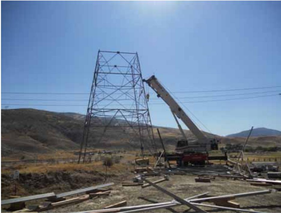
**Figure 1:** H&M steel crew assembling Tower 29, Segment 5.
