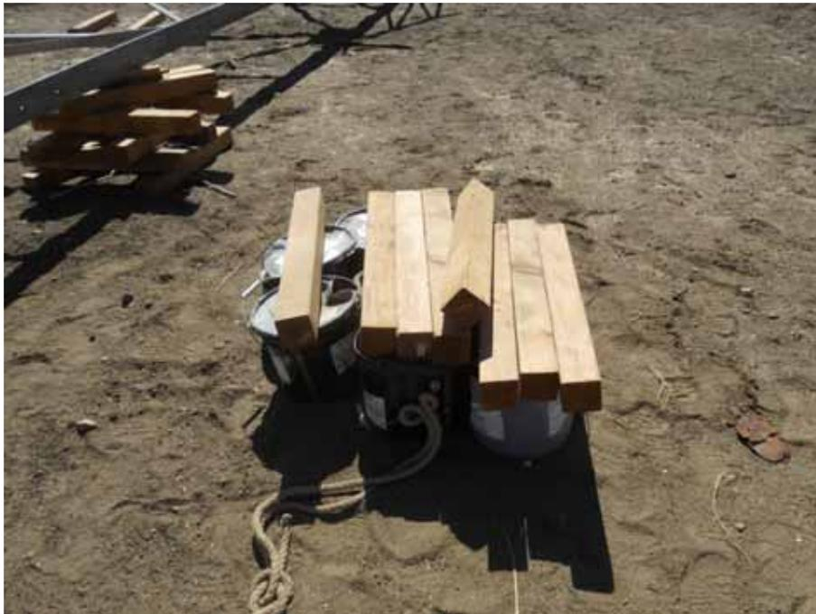
**Figure 2:** Covered bolt buckets at Tower 29, Segment 5.
