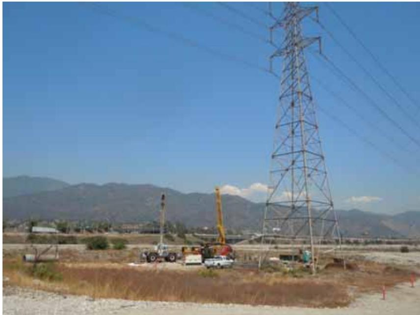
**Figure 6:** A Tri-State crew drills a foundation, Segment 7.
