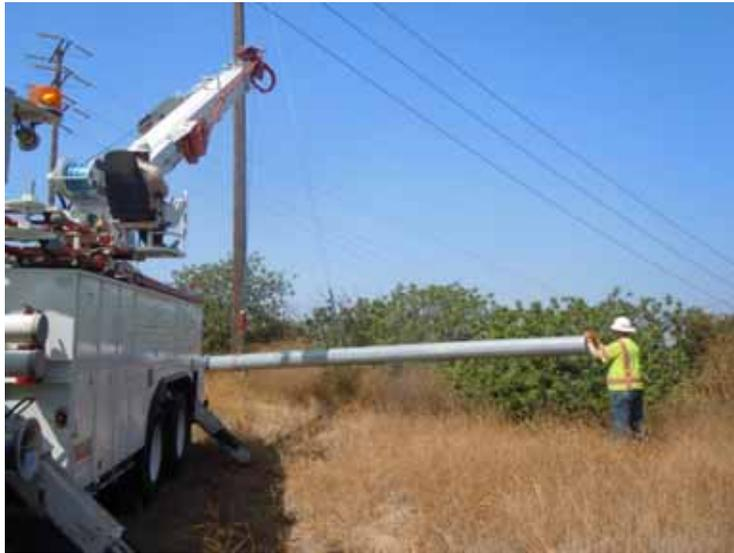
**Figure 5:** An SCE crew erects a lightweight steel pole, Segment 7.
