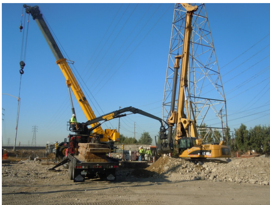
Figure 6: A Tri-State crew drills a foundation, Segment 7.
