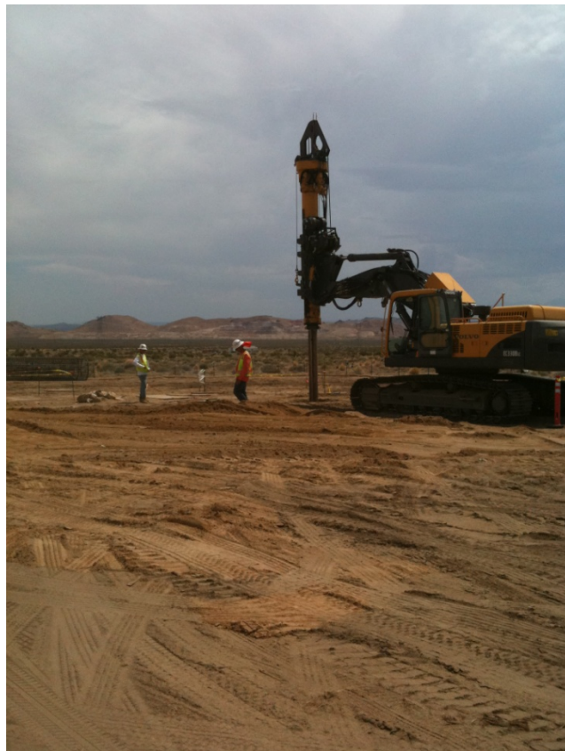
Figure 4: KV Structures drilling Tower 29, Segment 10.
