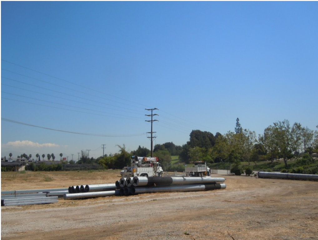
Figure 8: Steel poles and SCE vehicles parked/staged in an unapproved area. A CPUC Project Memorandum was issued on September 7.
