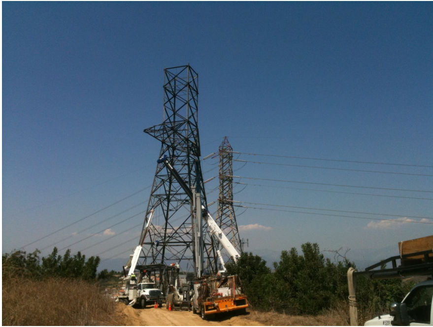
Figure 7: A Wilson crew assembles a tower within Tonner Canyon, Segment 8 Phase 1. Construction vehicles were parked on an access road, obstructing access from the western side of the site.
