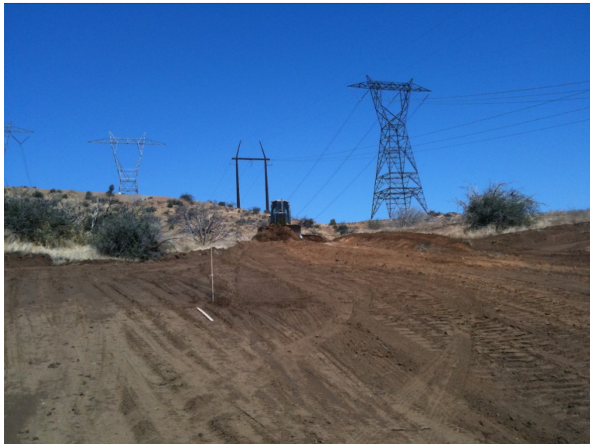
Figure 2: H&H Grading conducted clearing and grading of wire pull site near Tower 57, Segment 5.
