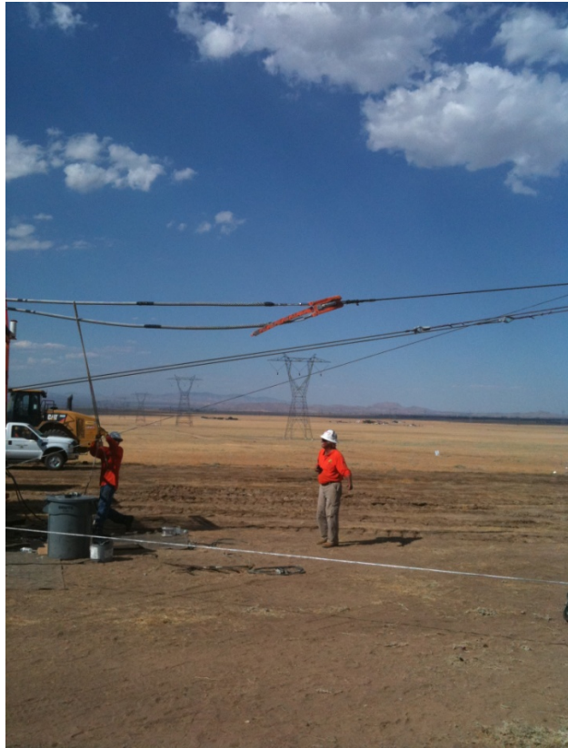
Figure 1: View of gator attached between the hardline and conductor during wire stringing activity, Segment 4.
