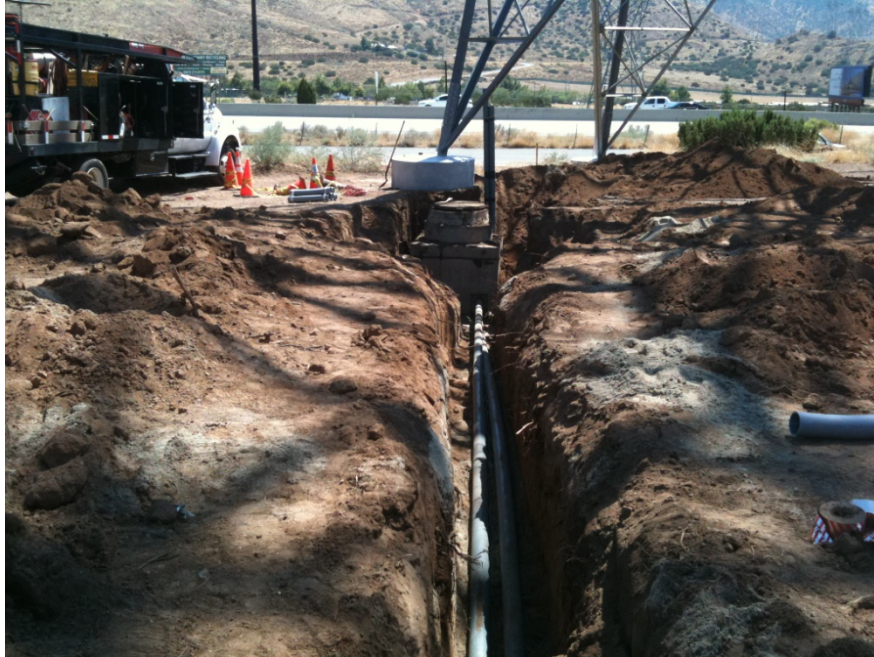
Figure 3: Underground fiber optic cable installation near Towers 63 and 64, Segment 5.
