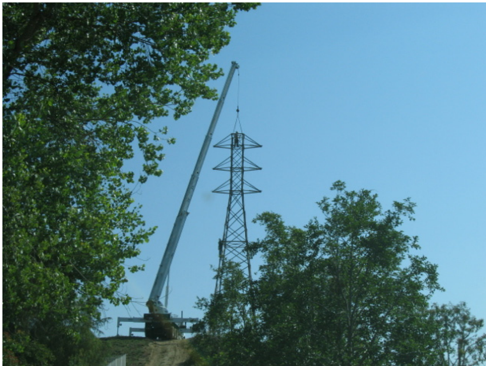
Figure 4: The removal of a 66 kV tower near Seco Canyon. A crane truck removed the tower in sections.
