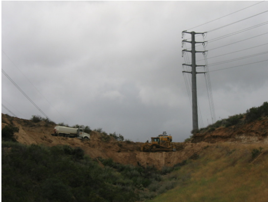
Figure 1: New crane pad construction at NC 9. Once the pad is constructed, the auger truck will be mobilized to drill the new tower foundations.
