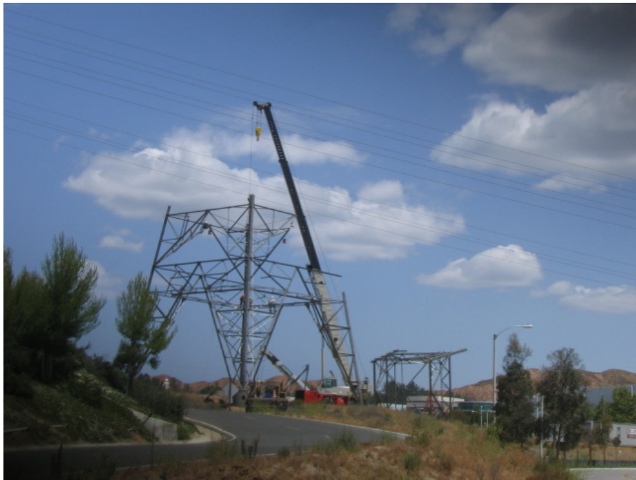
Figure 2: Assembly of 500 kV New Construct tower (NC) 2 outside of the Pardee Substation.
