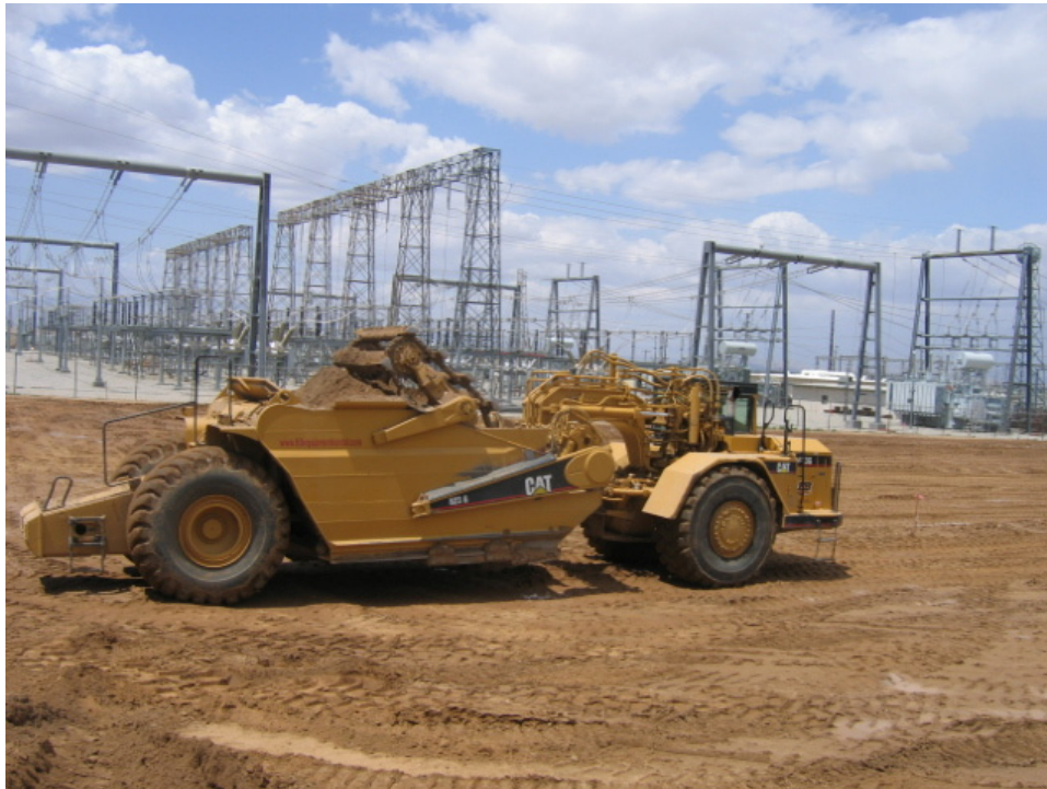
Figure 5: Grading and excavation of the Antelope Substation expansion area. Once the area matches the existing substation grade, rock placement will occur.
