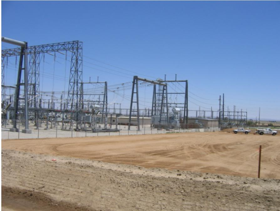
**Figure 2:** Grading of a portion of the Antelope Substation Expansion Area has been completed. Once the copper grounding is installed, rock will be brought in and the area will be fenced.
