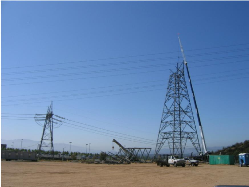
**Figure 1:** New 500 kV double circuit tower (NC2) under construction. This tower is the first one outside of the Pardee Substation, near Wal Mart. The tower in the background (left) will eventually be wrecked out after the new line is energized.
