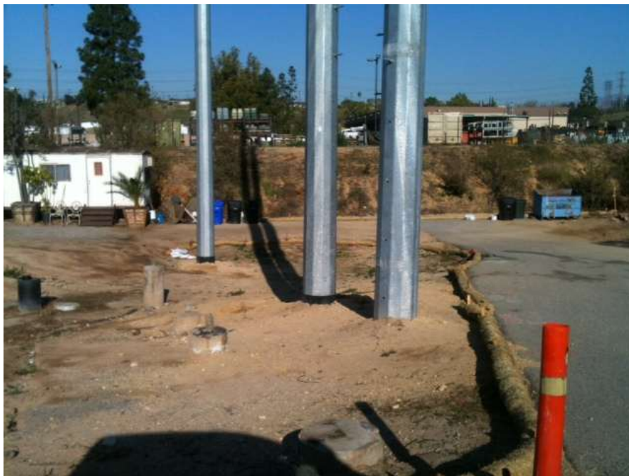
Figure 6: Newly installed fiber rolls, Segment 7.
