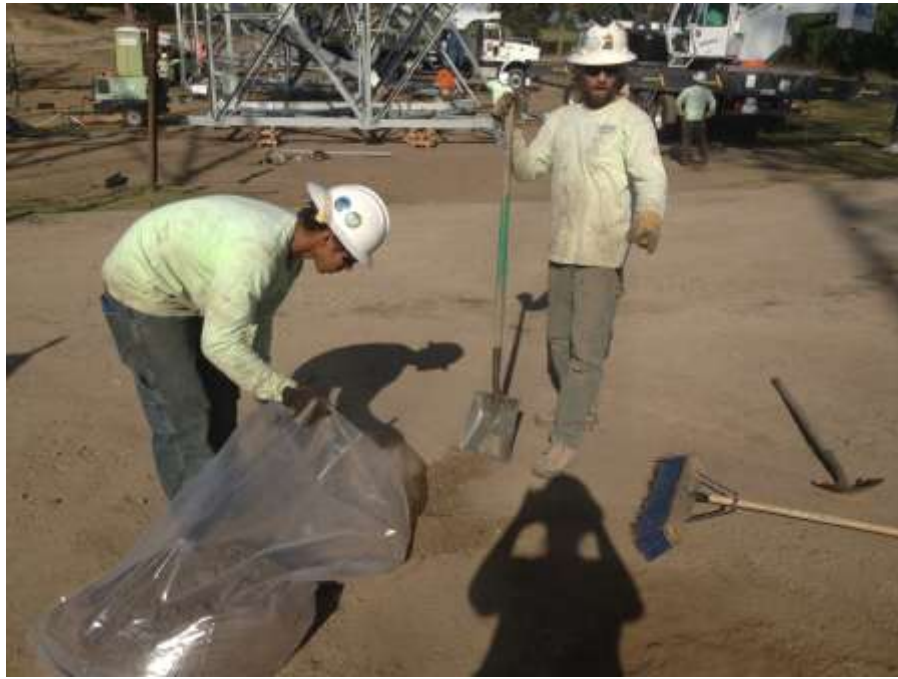
Figure 7: Contaminated soil removal at Tower M42-T3, Segment 7.
