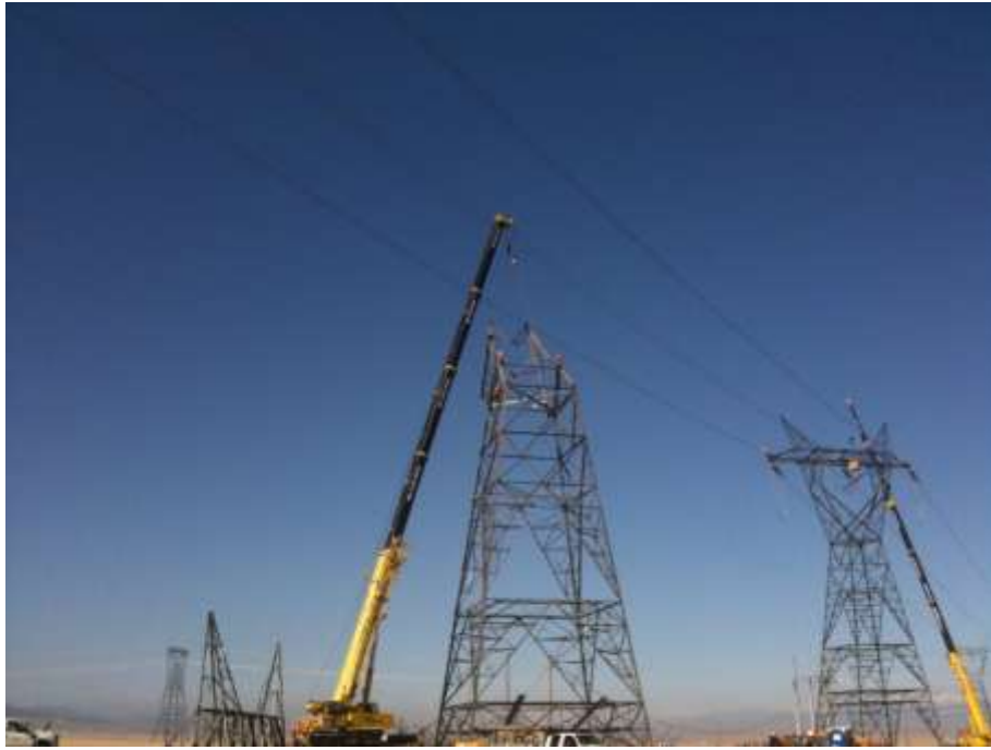
Figure 1: H&M steel crew erecting Tower 56, Segment 5.
