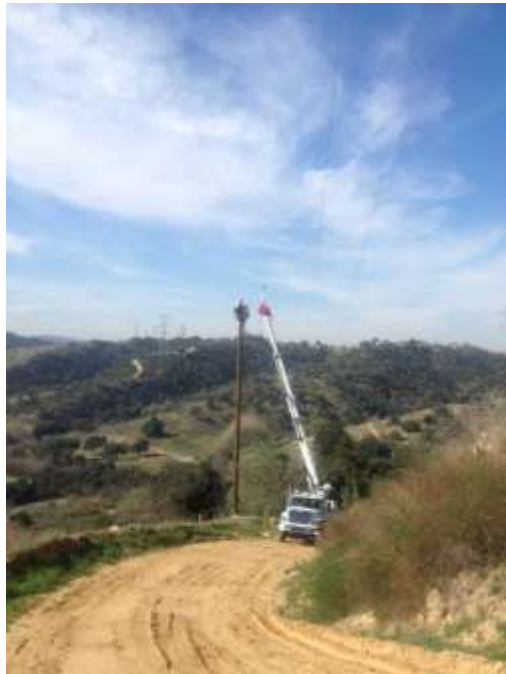
Figure 6: Distribution pole relocation, Segment 8 Phase 1.
