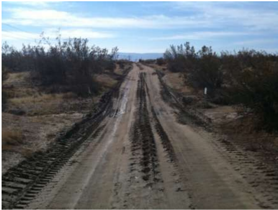
Figure 3: Graded jurisdictional drainage on General Petroleum Road conducted by non-TRTP activity, Segment 10.
