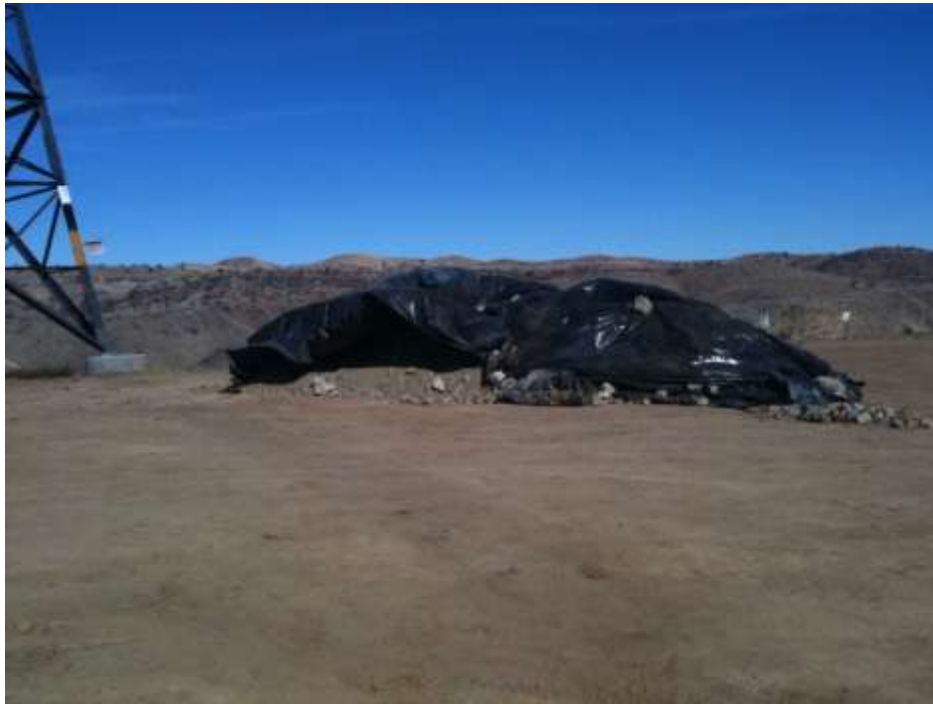
Figure 2: Ineffective stockpile covering at Tower 30, Segment 5.
