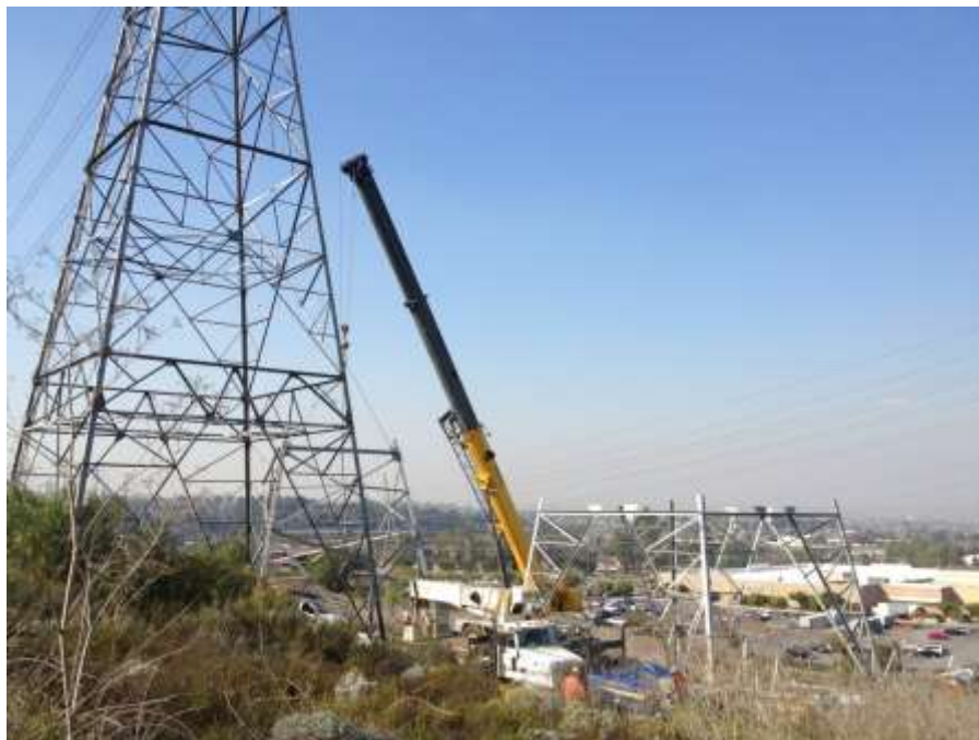
Figure 4: Tower assembly within Montebello Hills, Segment 7.
