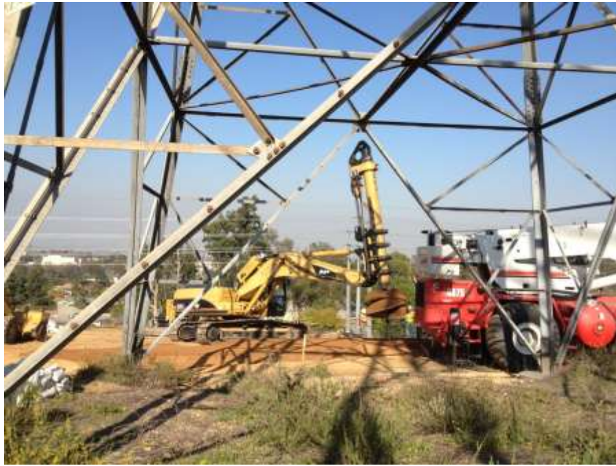
Figure 5: Foundation drilling at Tower M41-T4, Segment 7.
