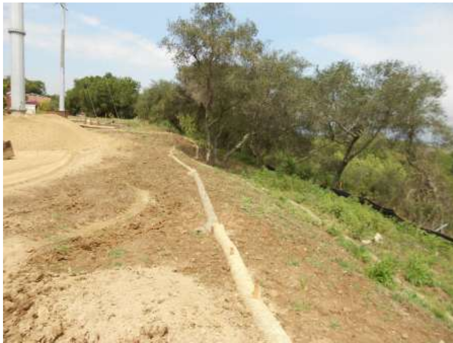
Figure 5: Newly installed fiber roll, Segment 8, Phase 4.
