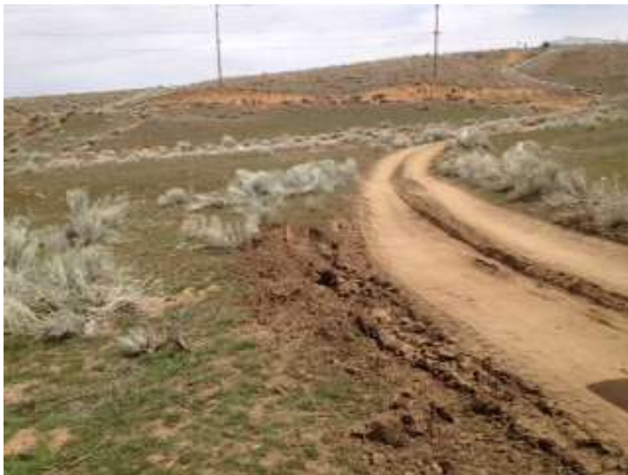
Figure 2: Tire tracks on top of access road berm in close proximity to a cultural site, Segment 3B.
