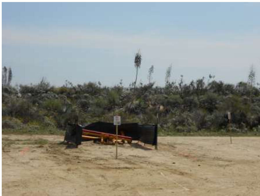
Figure 6: A silt fence for protective screening around a Bewick's wren nest, Segment 7.
