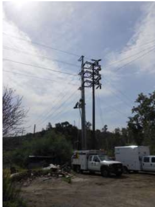
Figure 4: A crew member pulls conduit on a riser pole, Segment 8 66 kV.
