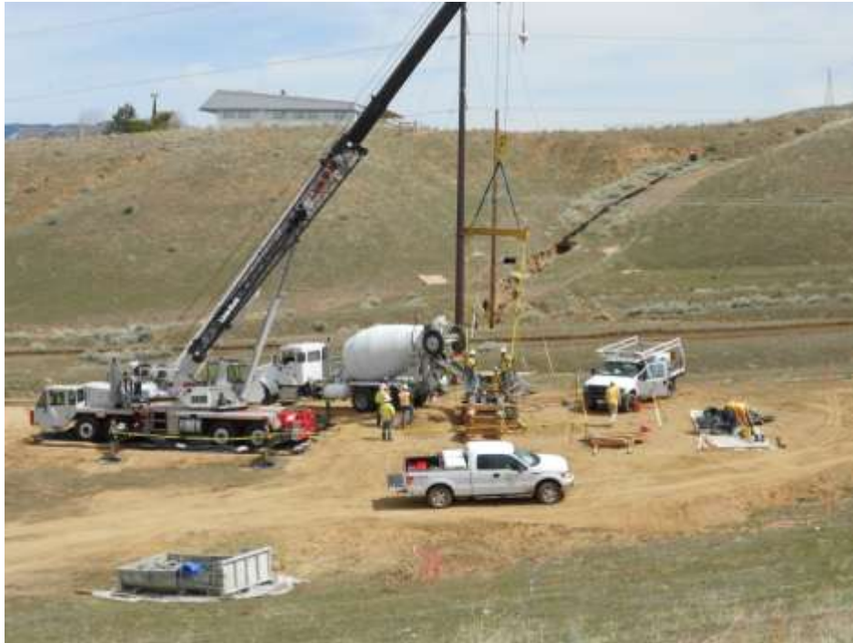
Figure 1: Concrete foundation pour at Construct 9, Segment 3B.
