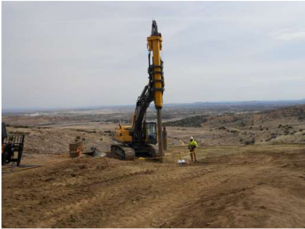
Figure 3: KV Structures drilling Tower 86A, Segment 5.
