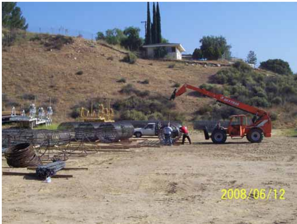
Figure 2: Crews loading steel cages for placement into caissons for concrete pouring.
