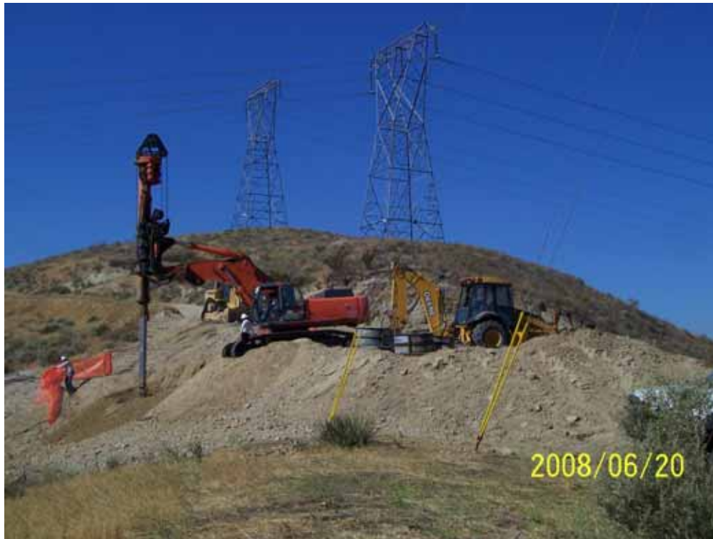
Figure 1: Foundation drilling at NC24.
