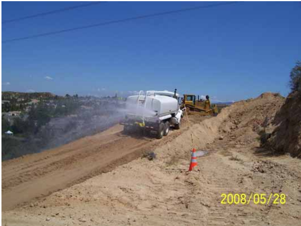
Figure 4: Dust control along access roads near NC 23.
