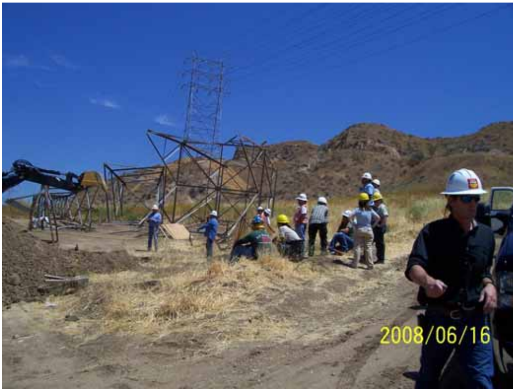
Figure 3: Forest personnel observing excavations of tower footings in order to assess the level of ground disturbance.
