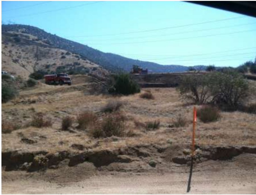
Figure 3: Sagebrush pad construction at Construct 236A.
