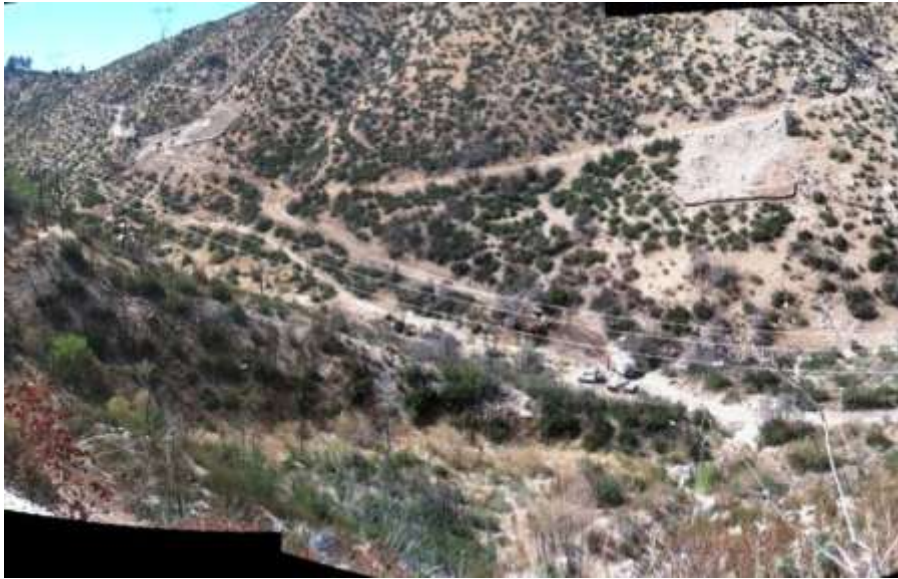
Figure 5: Segment 6 site grading at Constructs 32 and 33.
