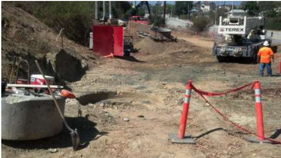
Figure 12: Gas monitoring equipment setup adjacent to footer drilling area at Construct M40-T4, Segment 7.
