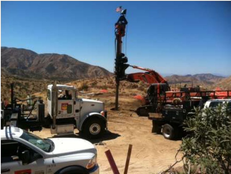
Figure 6: Segment 6 foundation excavation activities at Construct 21.
