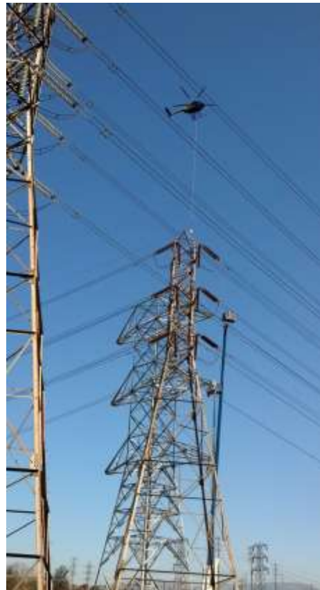
Figure 8: Flying sock line during wire stringing operations on Segment 7.
