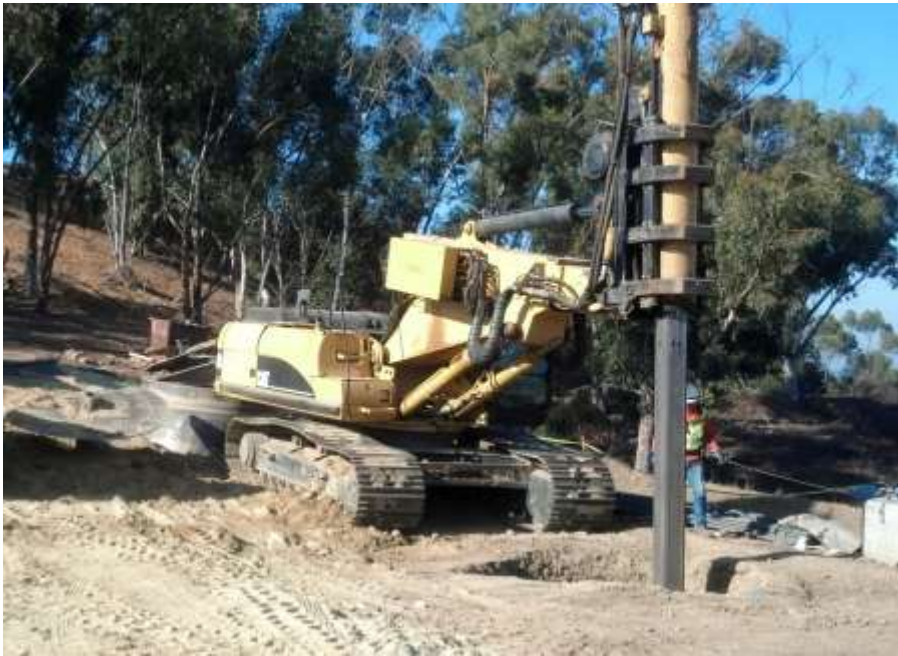
Figure 10: Foundation drilling with worker tied into safety harness at Construct M49-T3, Segment 8, Phase 4.
