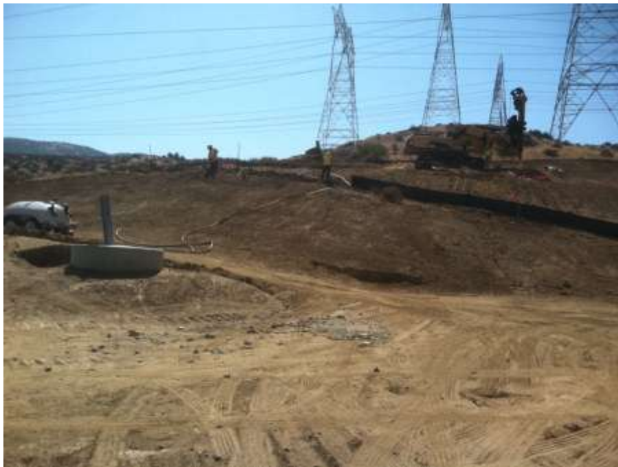
Figure 4: Sagebrush foundation drilling at Construct 235A.
