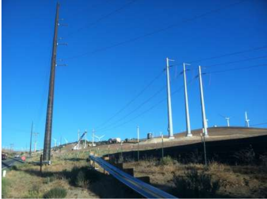
Figure 1: Segment 3B Wire Stringing operations at Construct 34/35.
