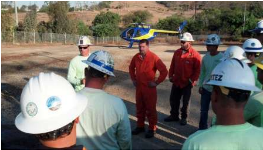
Figure 7: Safety briefing prior to wire stringing operations on Segment 7.
