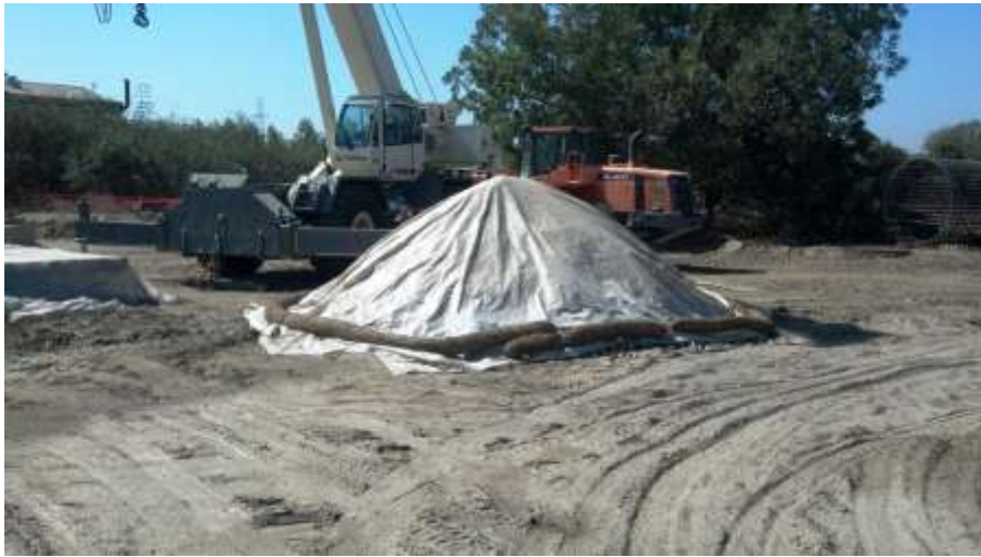
Figure 9: SWPPP installation on and around a soil pile.
