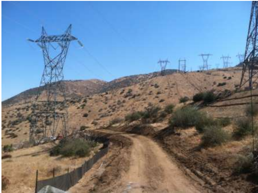
Figure 2: Sagebrush road grading to Construct 236A.
