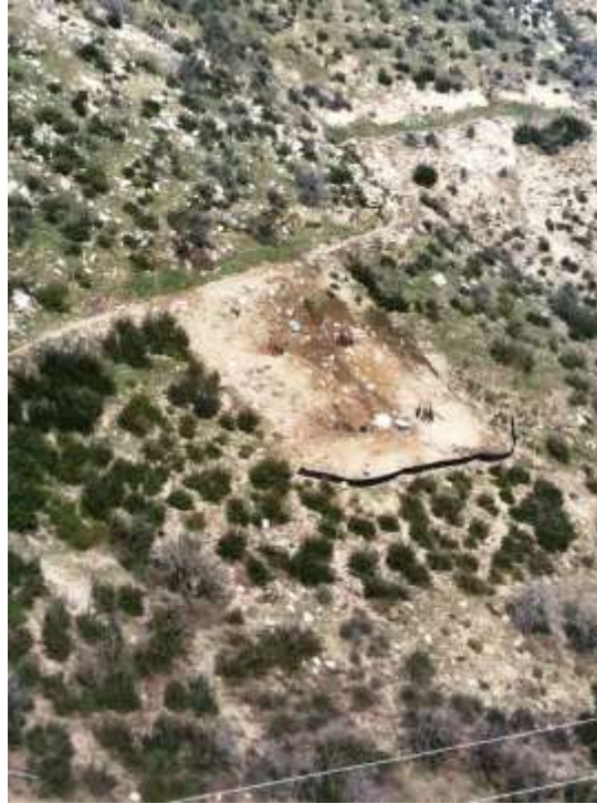
Figure 1: Foundation activities at Construct 32 on Segment 6A.
