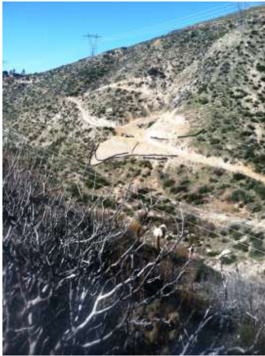
Figure 3: BMP installation at Construct 33 on Segment 6A.
