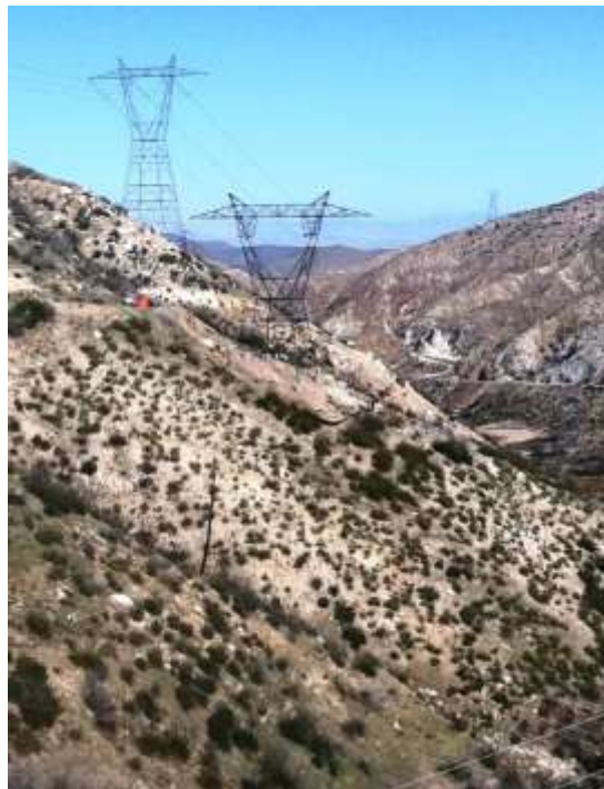
Figure 2: Structure erection at Construct 31 on Segment 6A.
