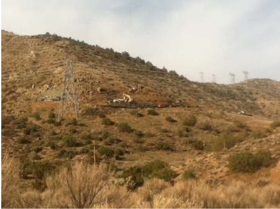
Figure 1: Grading activities at Construct 8.
