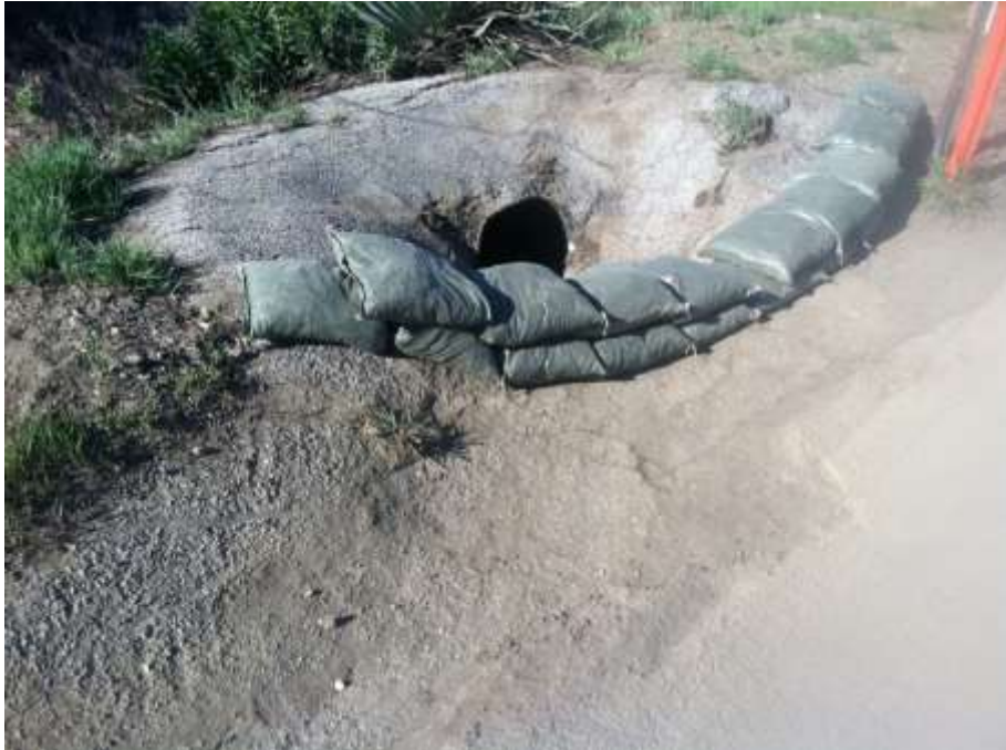
Figure 2: BMP installation on Angeles Crest Highway.
