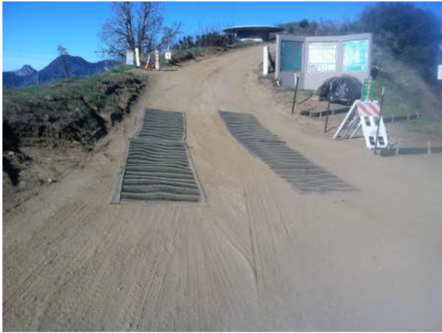
Figure 3: Trackout mats installed at the entry to Loop Road L in response to PM #9.
