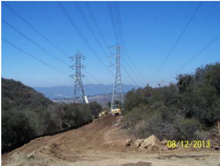
Figure 3: Grading activities at Pull Site between Constructs M1-T4 and M2-T1 on Segment 11B.
