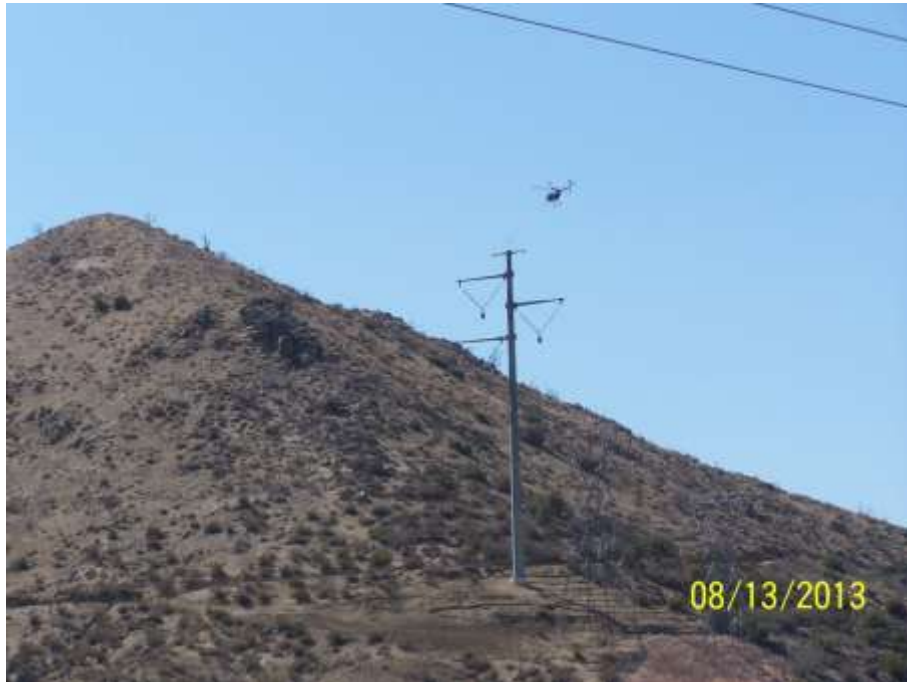
Figure 2: Wire stringing activities occurred between Constructs 2 and 11 on Segment 6A.
