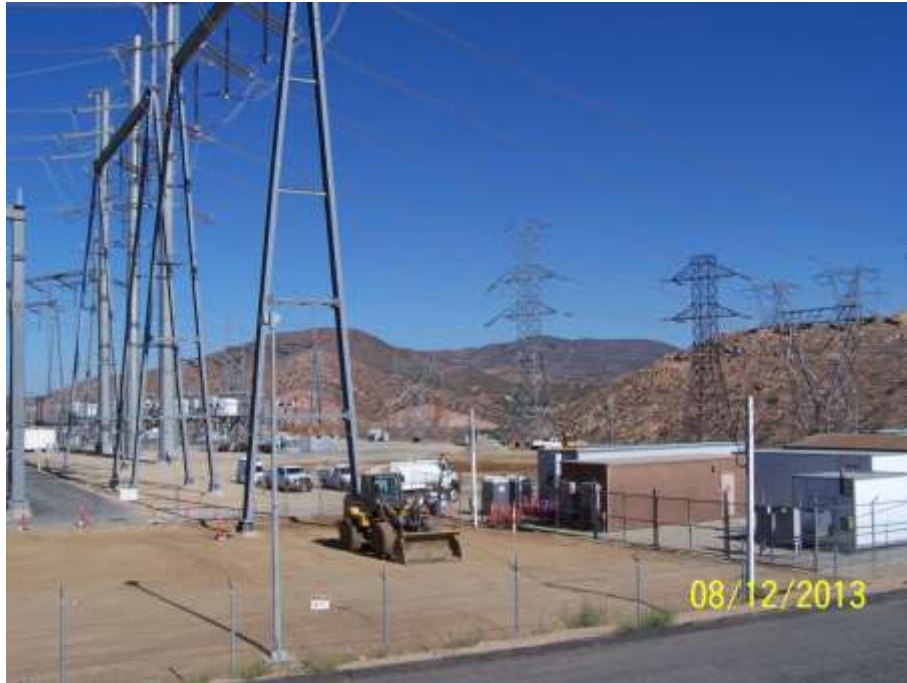
Figure 1: Vincent Substation grading activities.
