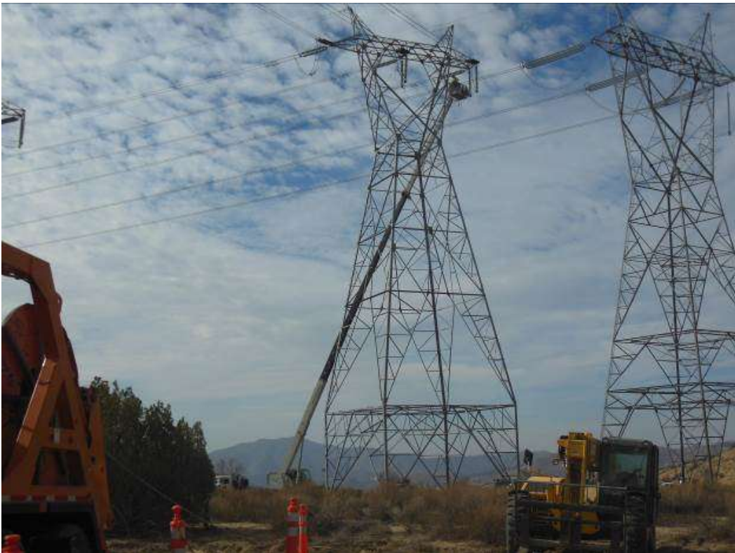
Figure 4: Removing jumpers from existing Tower M32-T3, Segment 11C.
