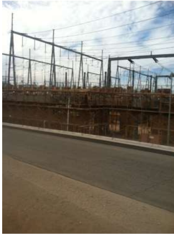
Figure 1: Vincent Control Building construction on Segment 9.
