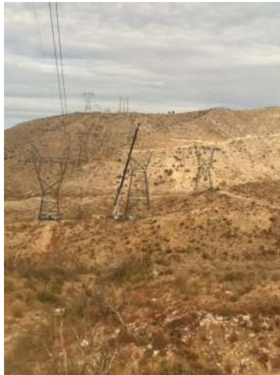
Figure 2: Structure assembly occurring at Construct 21 on Segment 6.
