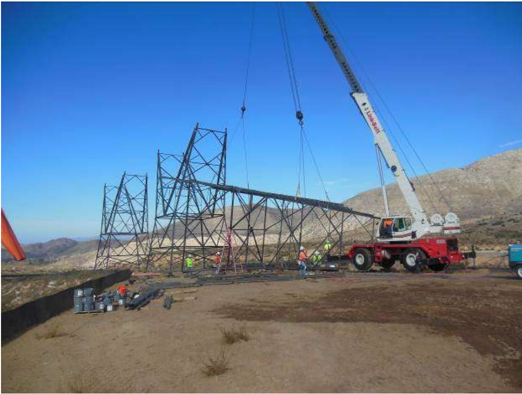
Figure 3: Assembly of towers for Segment 11C occurring at Aliso HAY.
