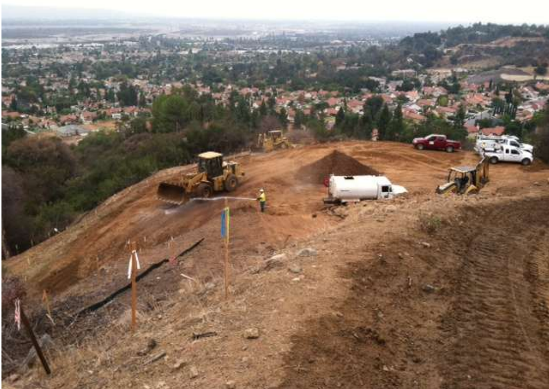
Figure 6: Grading access road to Segment 7 Tower M27-T3 in Duarte.
