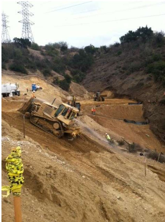
Figure 7: Grading access road to Segment 8 Tower M57-T1 in Tonner Canyon.
