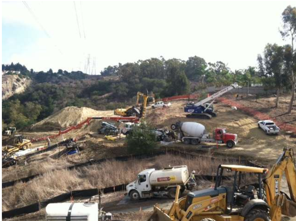
Figure 8: Foundation pouring at Segment 8 Tower M49-T1 near Puente Hills.
