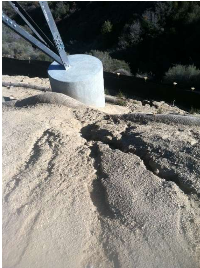
Figure 4: Rilling observed at Construct 58 on Segment 6.
