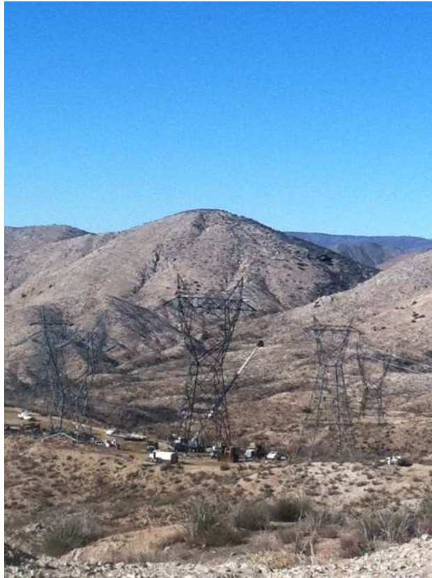
Figure 1: Construct 22 wire stringing activities, Segment 6.
