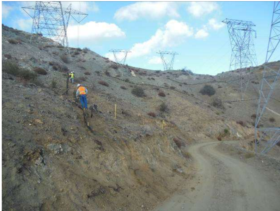
Figure 2: BMP installation at Construct 8 on Segment 11.
