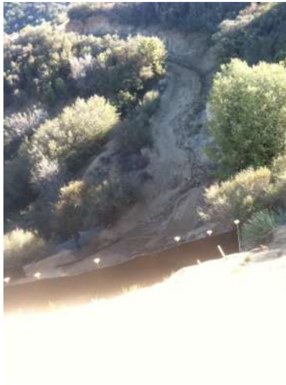
Figure 5: Sediment flow that can be seen going towards Waters of the US at Construct 58 on Segment 6.
