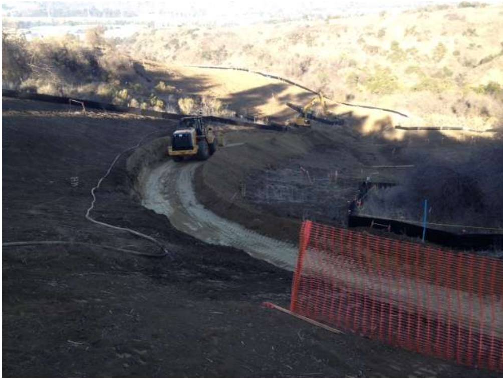
Figure 9: Patriot crews grading access road at Tower M43-T3 in Segment 8, Phase 4.
