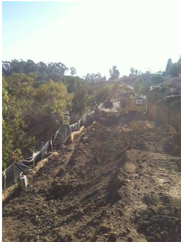
Figure 10: Patriot crews grading access road at Tower M49-T1 in Segment 8, Phase 4.
