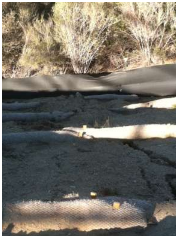
Figure 6: Sediment flow over installed BMPs at Construct 58 on Segment 6.
