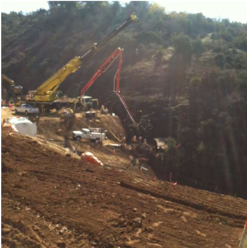
Figure 8: Union Engineering excavating and pouring foundations at Segment 8, Tower M57-T1.
