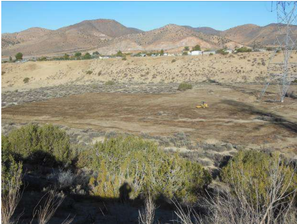
Figure 3: Grading at Wire Site associated with Construct 1 along Segment 11.
