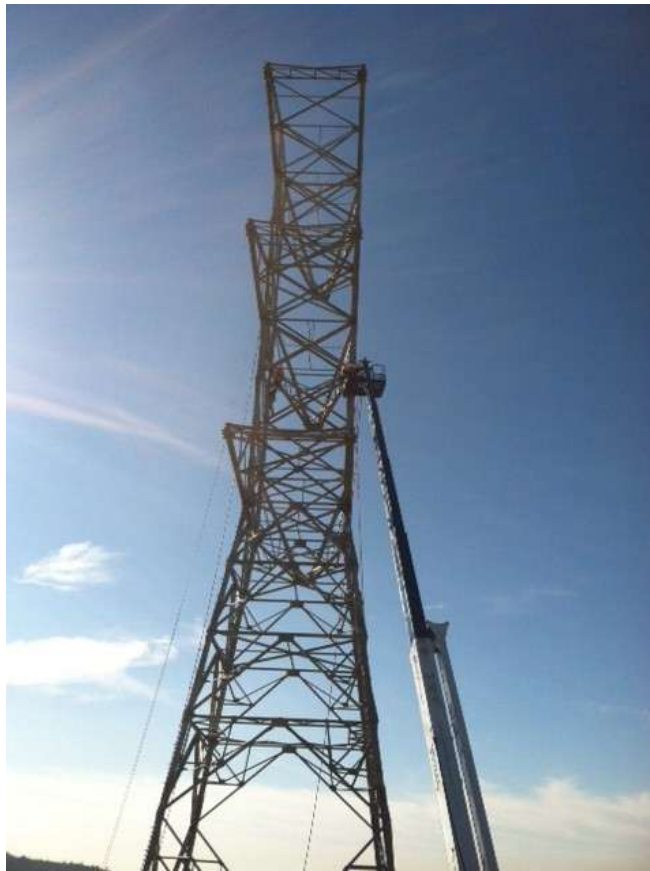
Figure 11: ASB crews assembling Tower M44-T3 in Segment 8, Phase 4.
