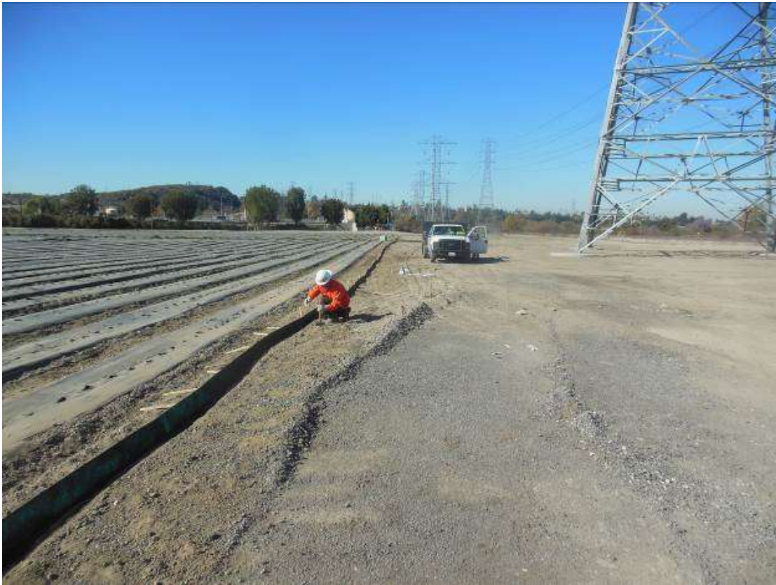
Figure 3: Installation of erosion control BMPs at Tower M41-T2, Segment 8.
