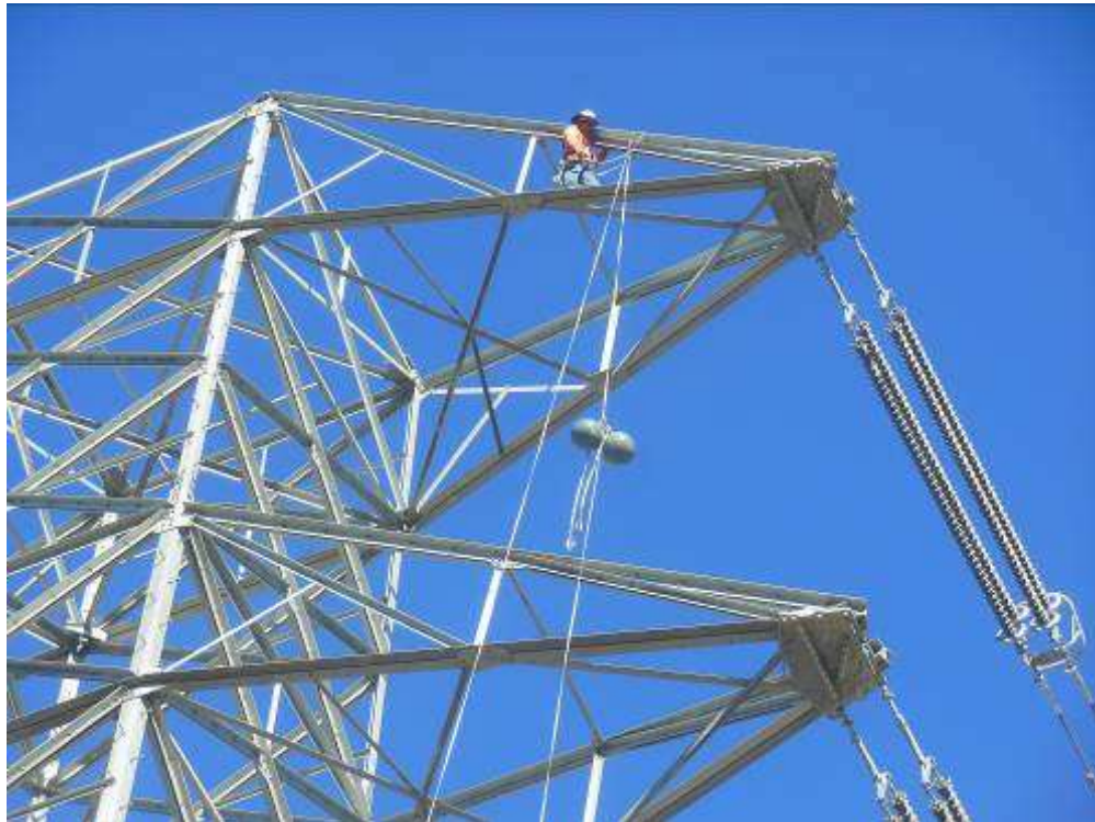
Figure 2: Bird deterrent buoys being installed at Tower M34-T1, Segment 7.
