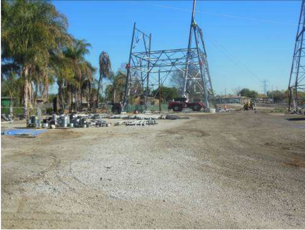
Figure 1: Assembly of tower sections onsite at Tower M37-T4, Segment 7.
