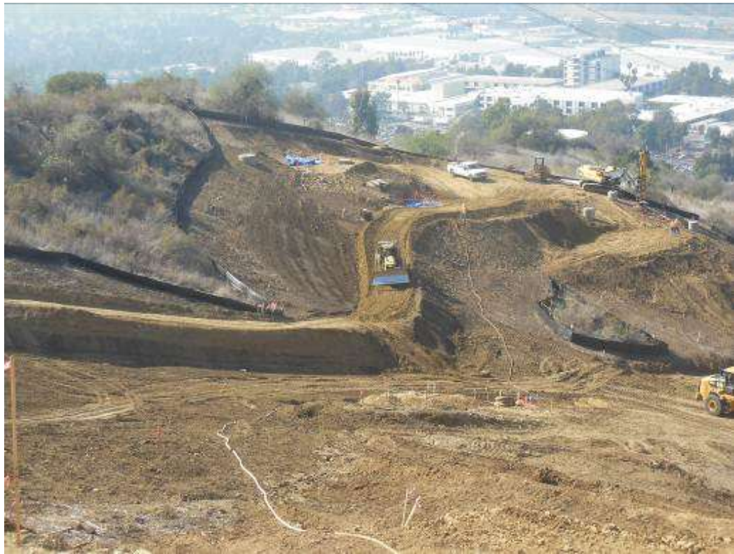
Figure 4: Patriot crews performing grading activities at Tower M43-T3, Segment 8, Phase 4.
