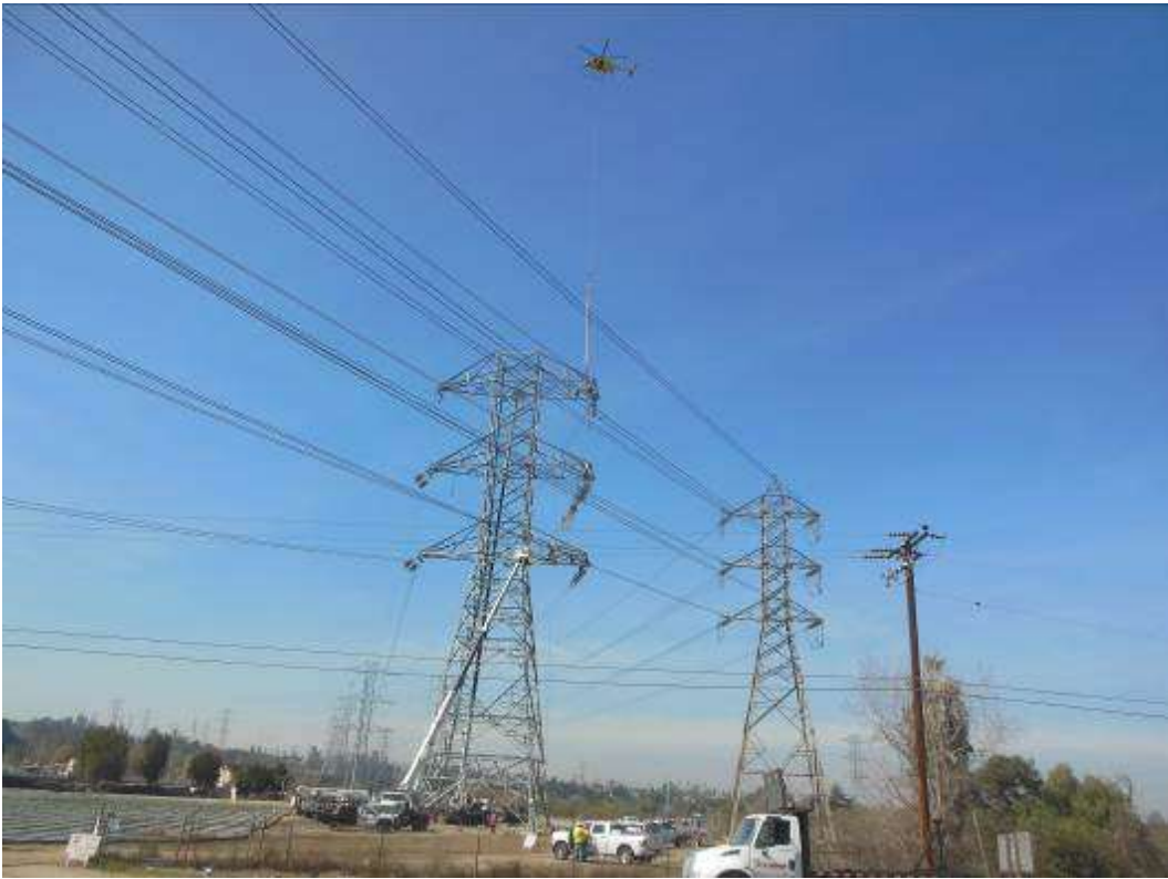
Figure 5: Wire stringing occurring between Towers M40-T4 and M42-T3, Segment 8, Phase 4.
