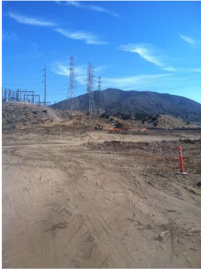
Figure 1: Ground disturbance at Construct M0-T1, Segment 11C.
