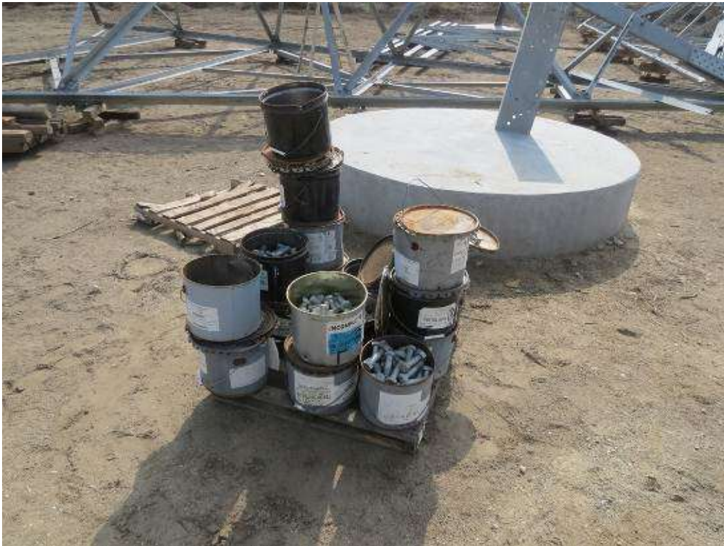
Figure 6: Uncovered bolt buckets identified by SCE Monitor at Tower M42-T5, Segment 8, Phase 4 (photo courtesy of FRED).
