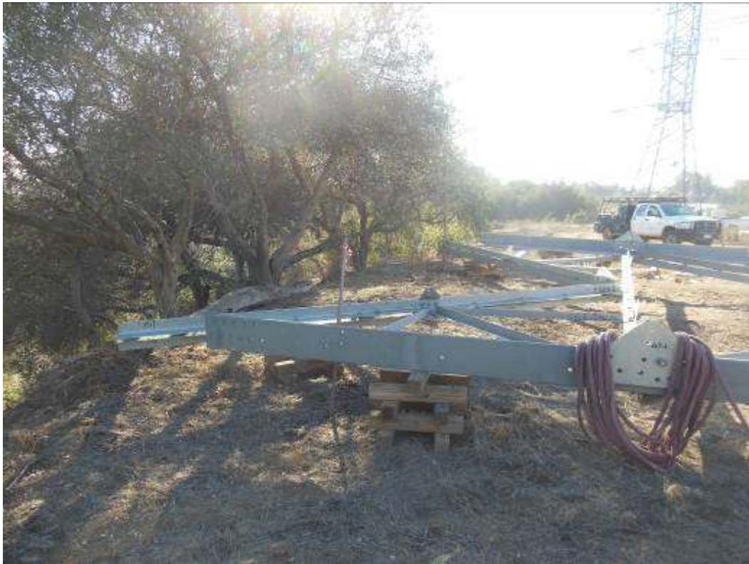
Figure 7: Assemble pieces of tower encroaching ESA for bat habitat at Tower M40-T3, Segment 7. Note red/white ESA staking in center.
