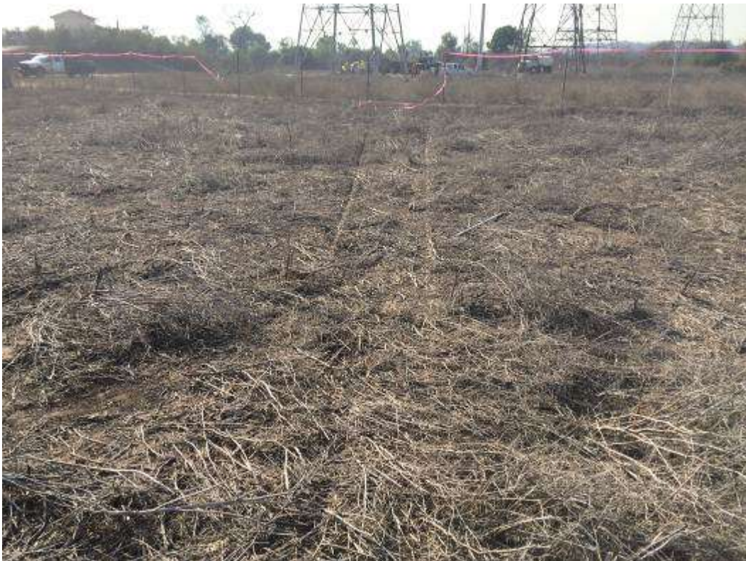
Figure 8: Visible markings within the vegetation from dropped wire between Tower M42-3 and WSS 8-4.12, Segment 8, Phase 4 (photo courtesy of FRED).
