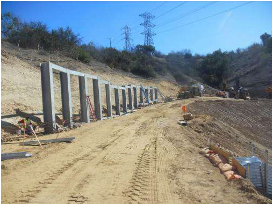
Figure 3: Construction of retaining wall at Tower M57-T1, Segment 8, Phase 1.
