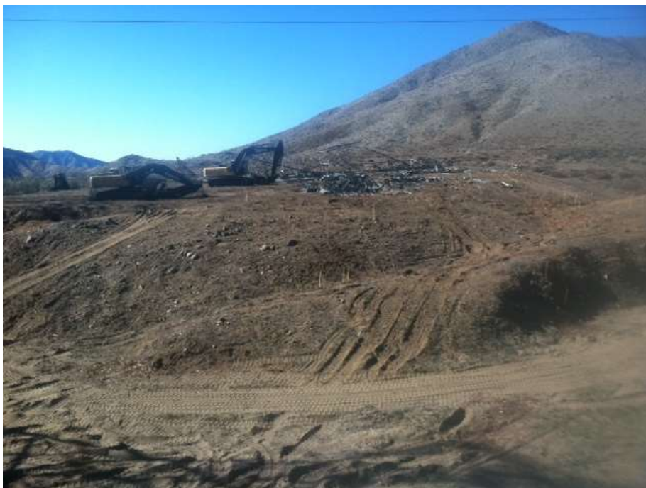
Figure 2: Wreck-out structures stored at Construct 11, Segment 11C.
