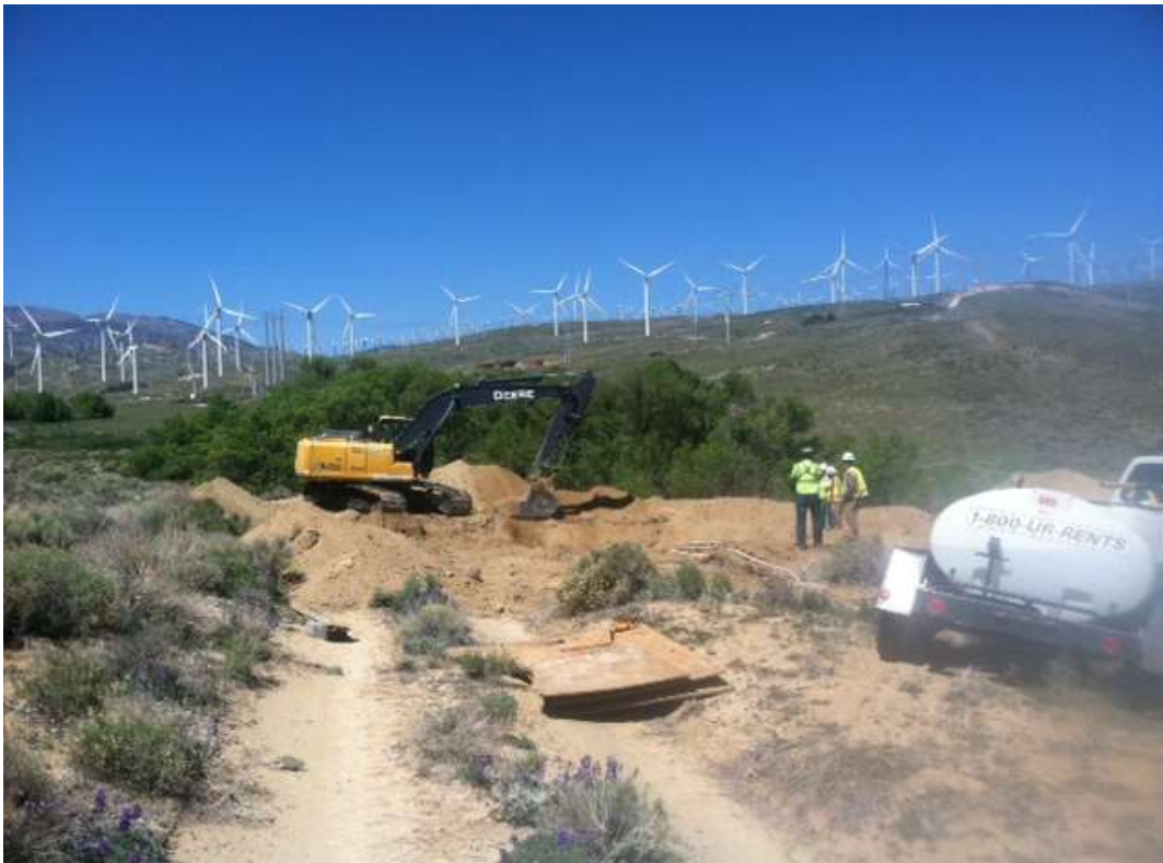
Figure 2: AC mitigation activities on Segment 3B.
