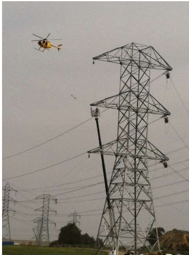
Figure 7: Wire stringing activities on Segment 8, Phase 4, at Rose Hills.
