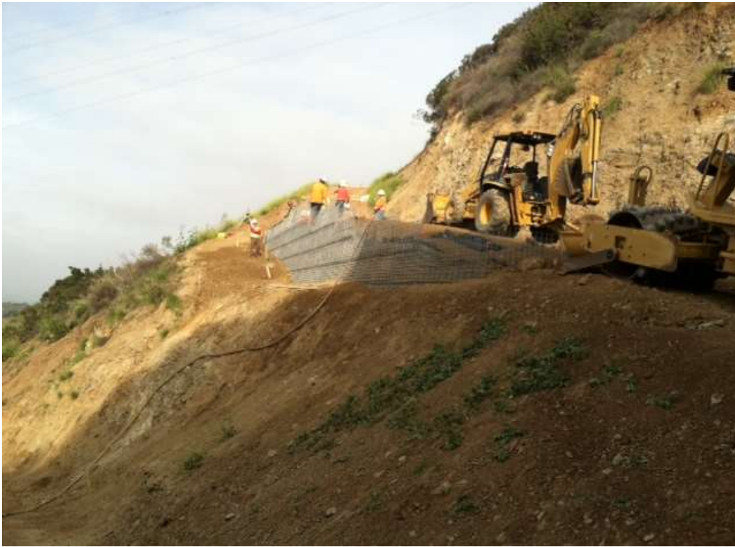
Figure 5: Wall construction along the access road to Tower M27-T3 in the City of Duarte, Segment 7.
