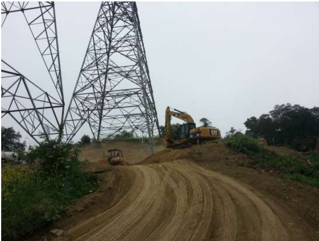
Figure 6: Road grading to Tower M50-T4, Segment 8, Phase 4 (photo courtesy of FRED).
