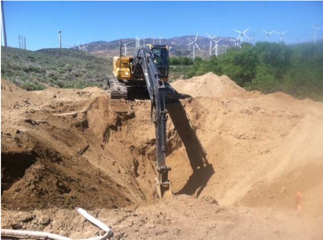
Figure 1: AC mitigation activities on Segment 3B.
