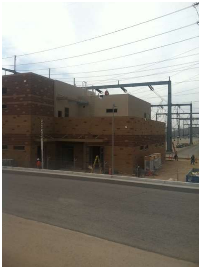
Figure 3: Vincent Control Building construction activities.
