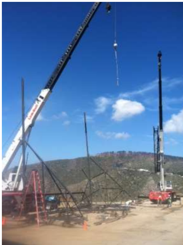
Figure 4: Erection activities occurring at Construct 5, Segment 11C.
