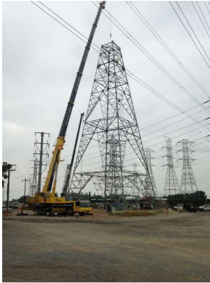
Figure 9: Tower assembly at Tower M42-,T2, Segment 8 Phase 4.
