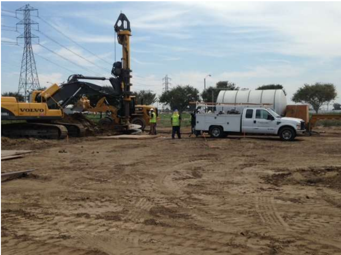
Figure 6: Foundation drilling in Segment 8, Phase 3.
