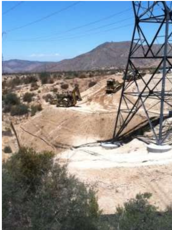
Figure 2: Grading activities at Construct 17, Segment 6A.
