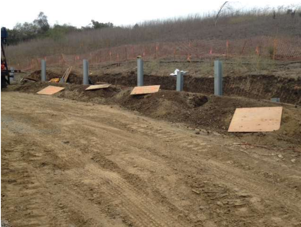
Figure 7: Wall construction along the access road to Tower M49-T1, Segment 8, Phase 4.
