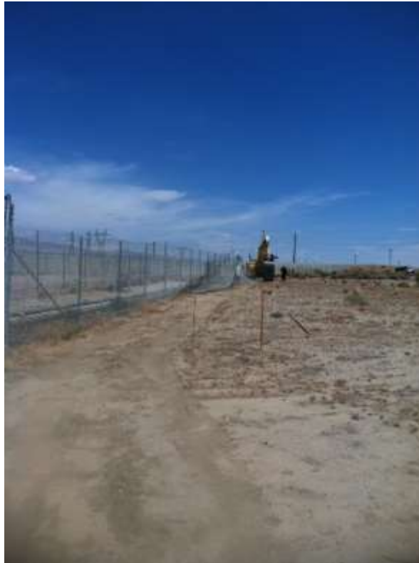
Figure 1: Fence removal at Whirlwind Substation.
