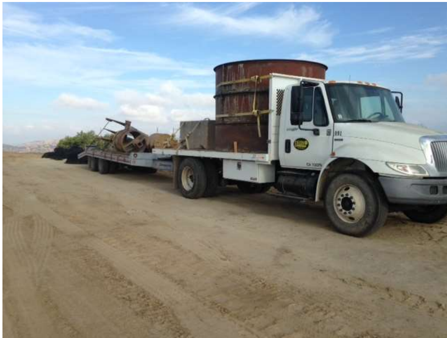
Figure 10: TRTP equipment and materials staged outside of approved work limits in Tonner Canyon, Segment 8, Phase 1.
