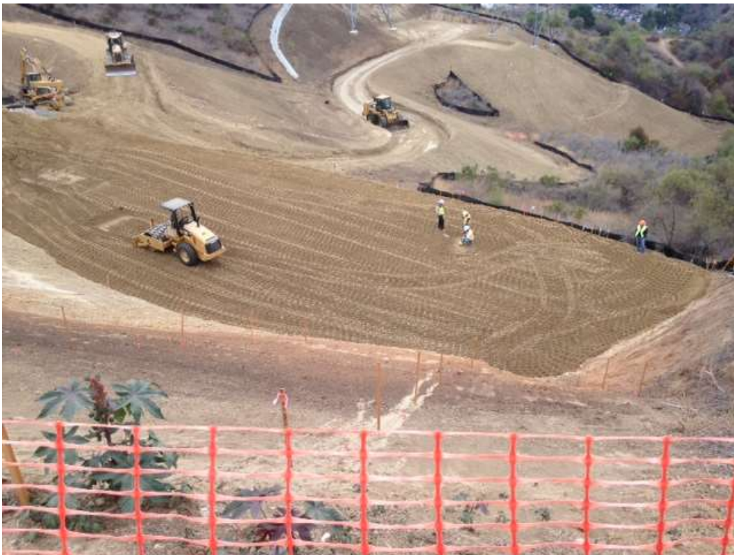
Figure 8: Grading at Tower M43-T3 in the landslide area, Segment 4, Phase 4.
