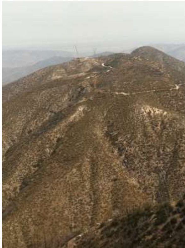
Figure 3: Micropile and conventional foundation activities at Constructs 28 and 29, Segment 11C.
