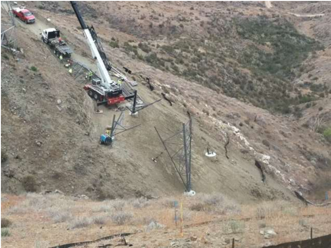
Figure 5: Erection activities occurring at Construct 9, Segment 11C.
