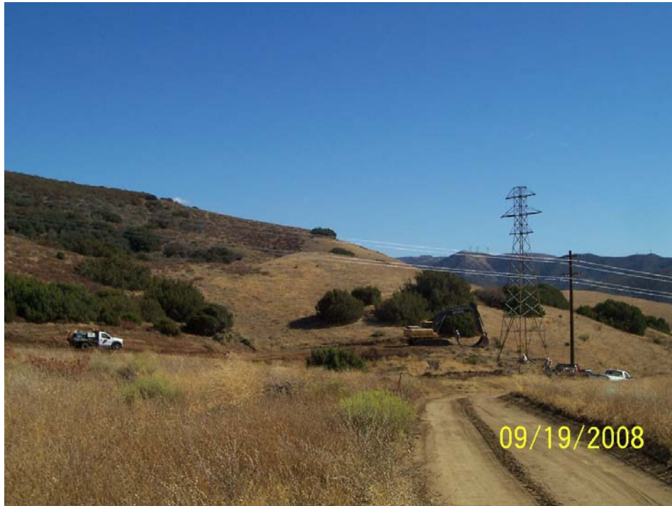
Figure 1: New temporary road construction to NC 97 in Section 3, completed after Variance was approved by the CPUC for change in access method.
