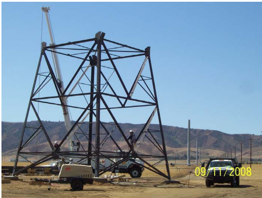
Figure 2: A combination of lattice towers and TSPs are being constructed to support the new 500 kV lines near the Antelope Substation.
