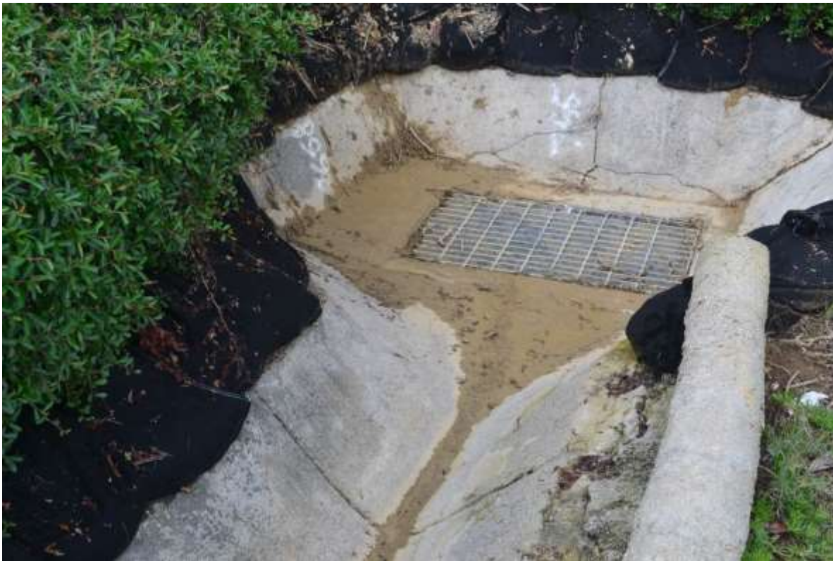
Figure 3: An unprotected storm drain with accumulated sedimentation from nearby project graded areas, Vault Cluster #11, 500 kV Underground.
