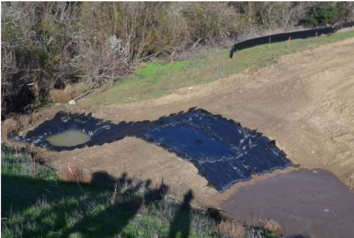
Figure 5: Settling ponds at the WTS used to collect and settle turbid water before it runs offsite. These pools were the subject of a safety concern for the public and were eventually fenced.
