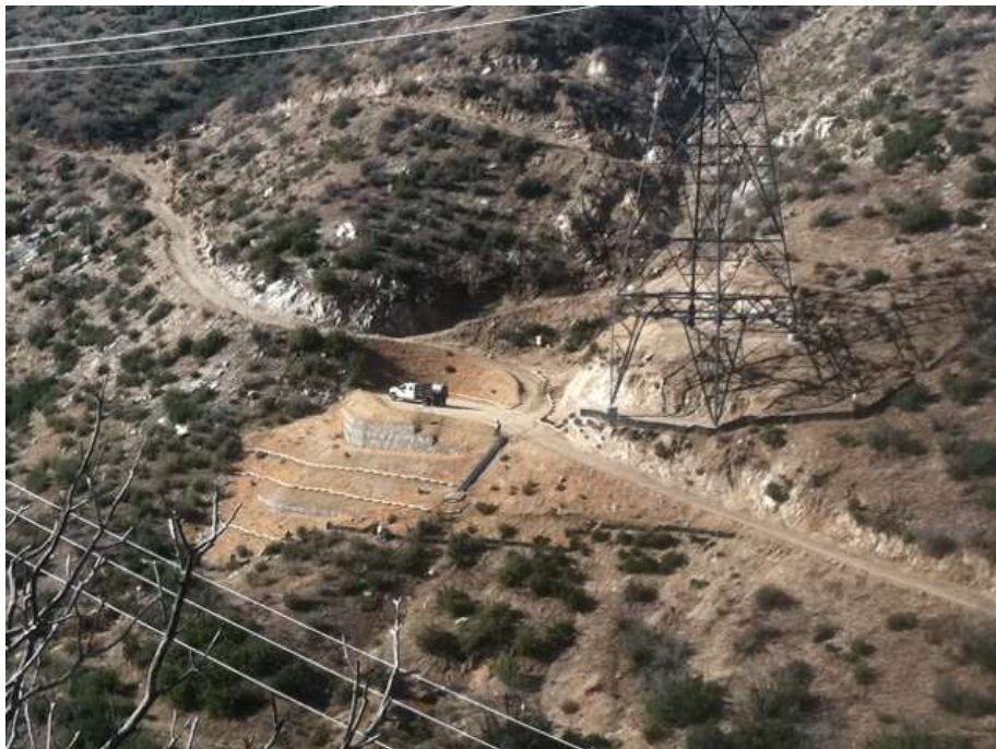
Figure 2: BMP maintenance at Construct 33, Segment 6A.
