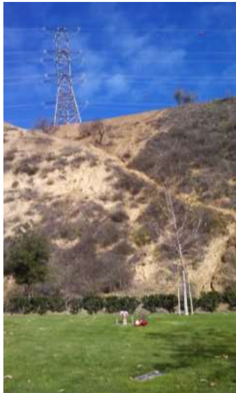
Figure 6: Erosion gully evident at Tower M44-T2 adjacent to Rose Hills Cemetery. Offsite sedimentation was documented by SCE's monitors.
