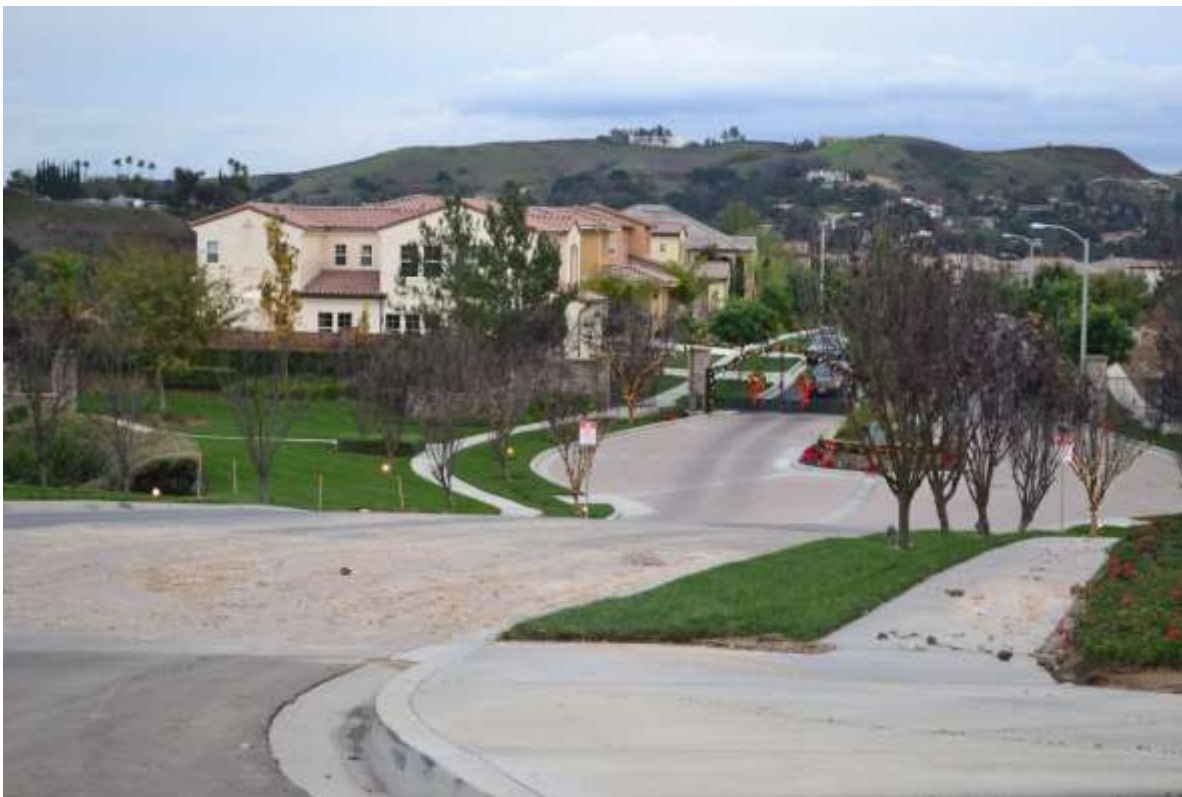
Figure 4: Offsite sedimentation onto Canon Lane in Chino Hills after the rain event on December 17. Construction street sweepers removed the sediment the following day.
