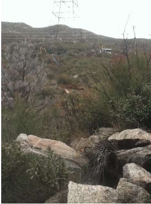
Figure 1: Road grading activities on Loop Road H, Segment 6B.
