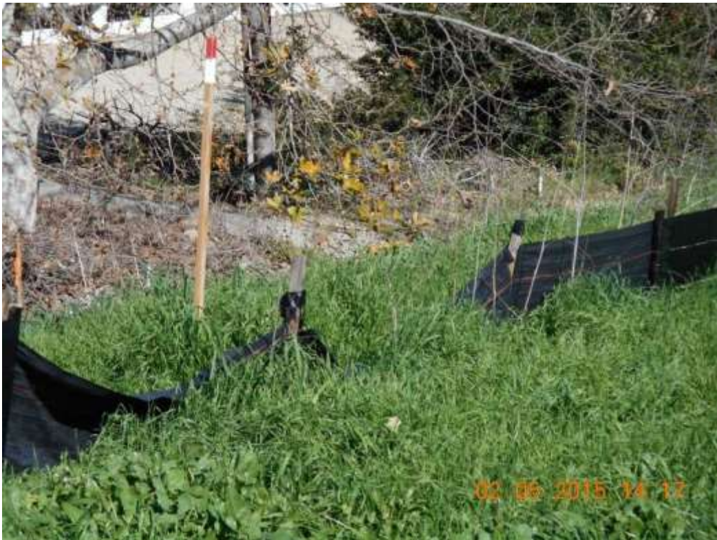
Figure 11: Damaged silt fencing at VC #8 recorded as a SWPPP maintenance action by SCE SWPPP inspectors (photo courtesy of SCE FRED).
