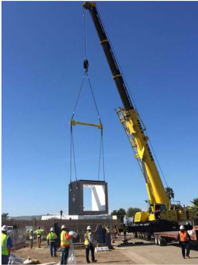
Figure 9: Vault Installation at VC #14 near Pipeline Avenue, Chino Hills.
