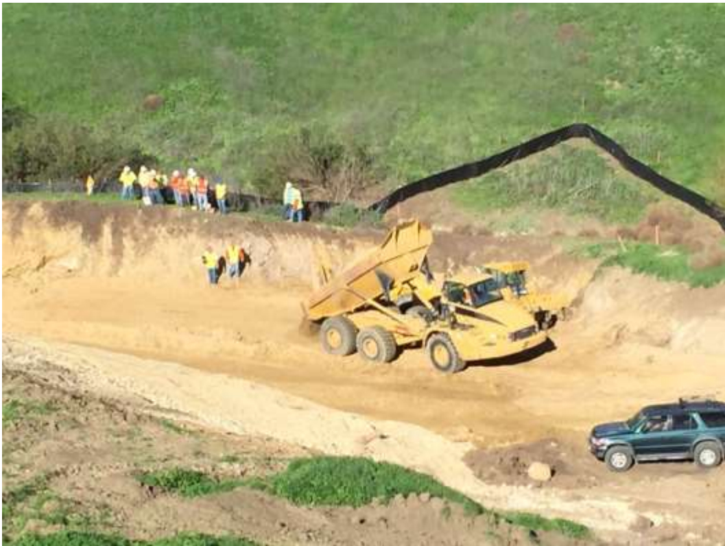
Figure 6: Importing soil and filling the keyway at the Western Transition Station, 500 kV Underground.
