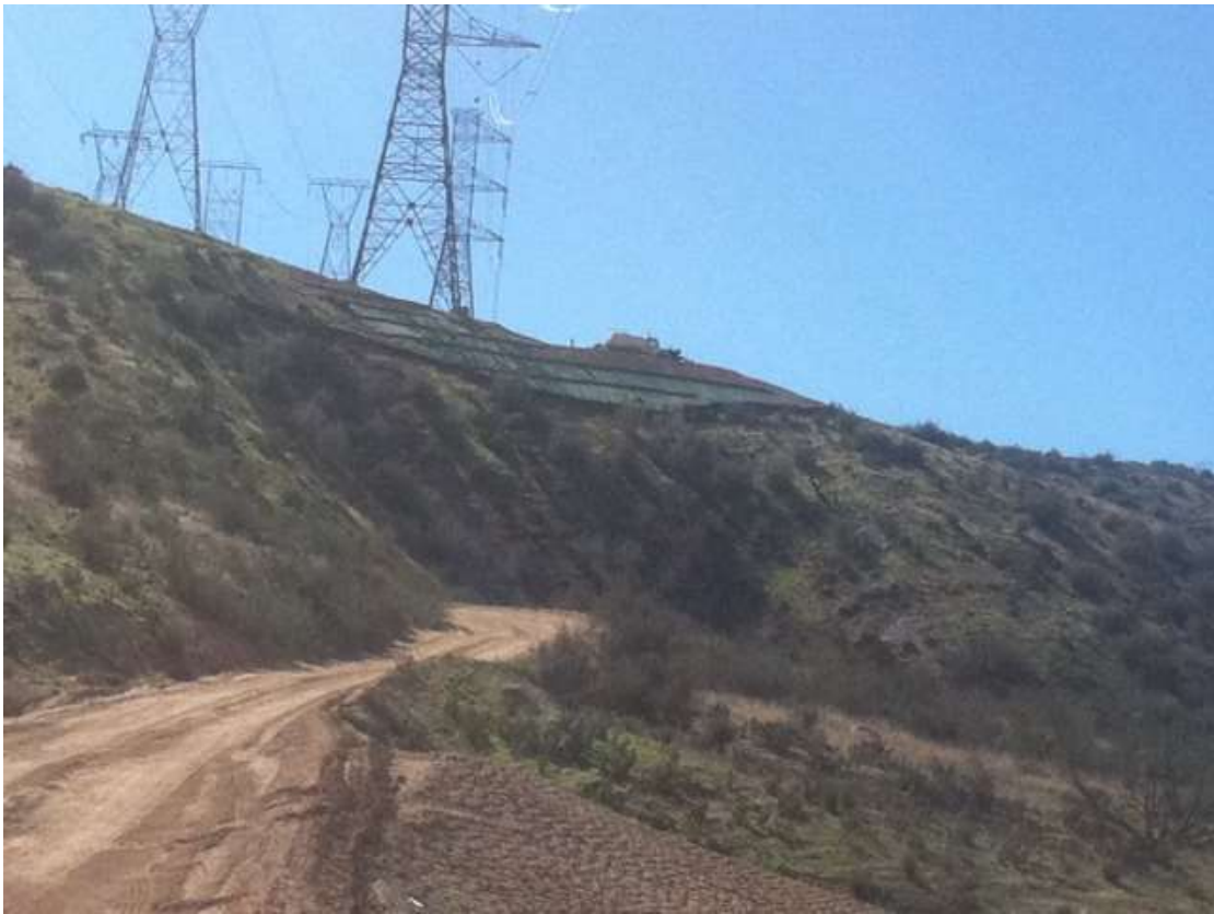
Figure 3: Hydromulch application as a BMP and site stabilizer at Construct 12, Segment 11C.
