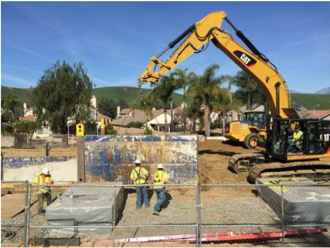
Figure 8: Setting shoring walls at VC #5, 500 kV Underground.
