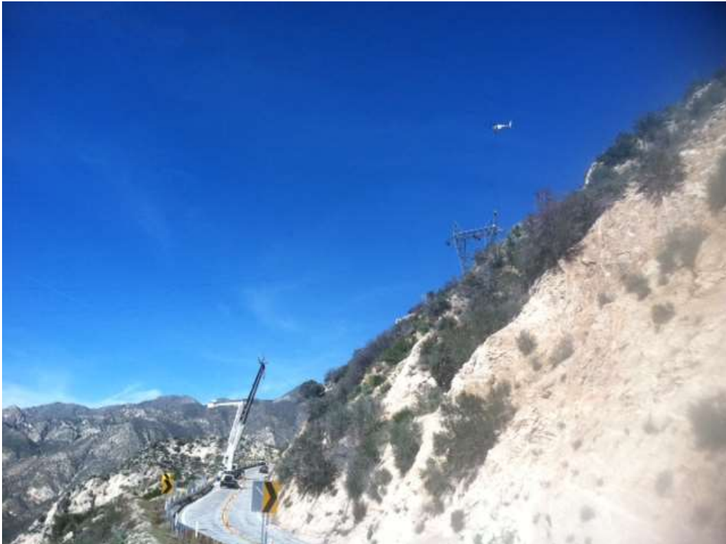
Figure 2: Wire stringing operations at Construct 57, Segment 11C.
