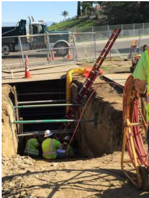
Figure 5: Conduit installation at the Cabrillo Street crossing, 500 kV Underground.
