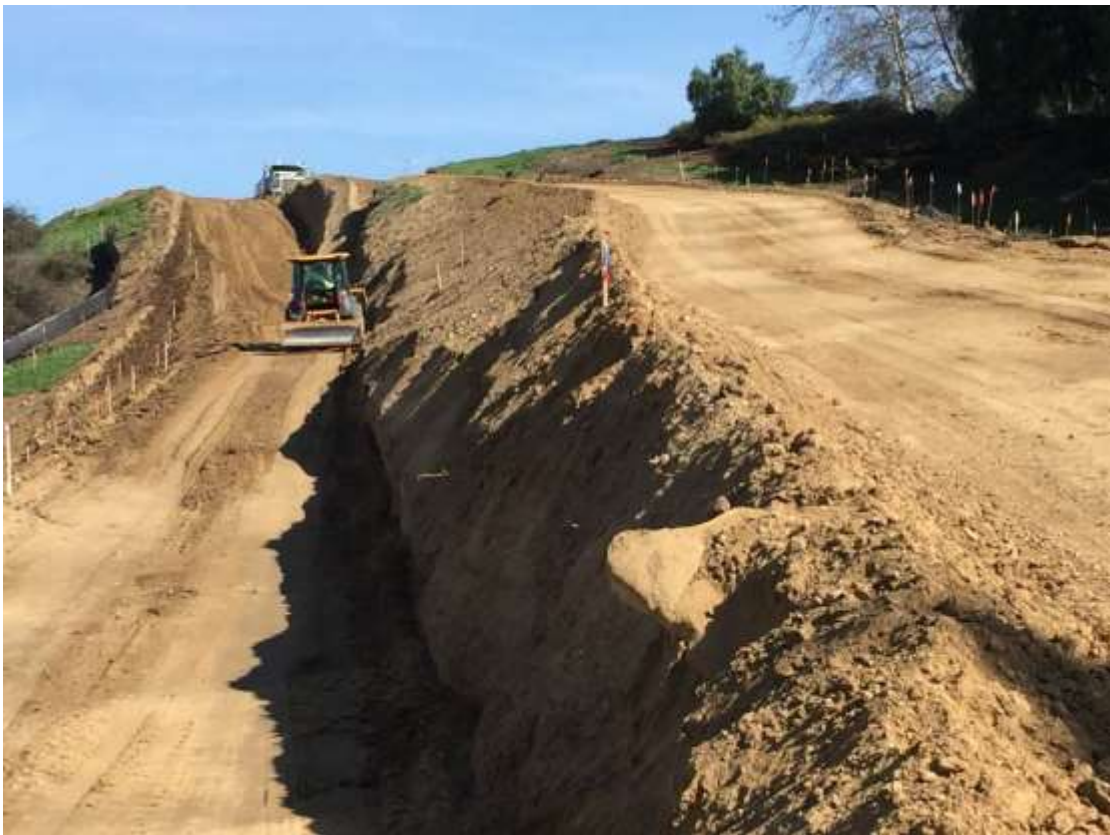
Figure 7: Access road grading between VCs #9 and #10, 500 kV Underground.
