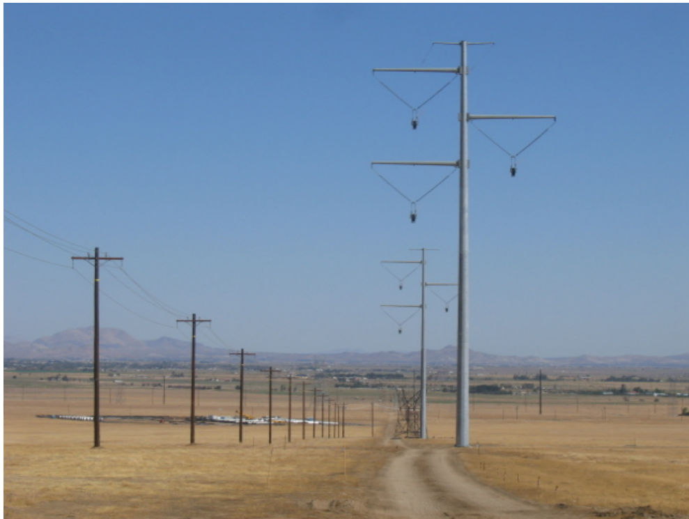
Figure 3: Tubular Steel Poles (TSPs) and Lattice towers will support the new 500 kV line in Section 3. The wood poles on the left are the newly installed Hughes Lake 12 kV relocated line.
