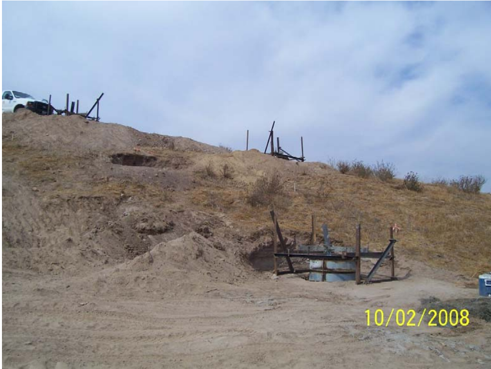
Figure 1: Foundations for NC 28 ready to be poured.
