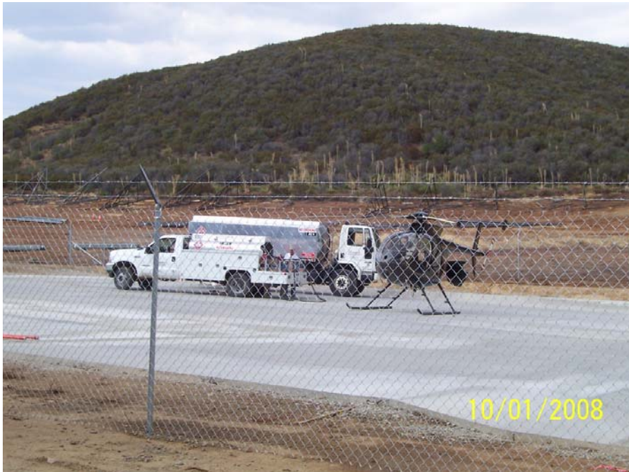
Figure 2: Conductor removal in Phase 2 ANF was carried out using the Hydrant Yard helicopter landing and refueling pad.
