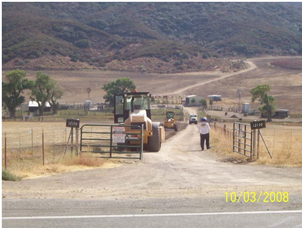
Figure 4: Road improvement at the Reitano Ranch, Section 3.
