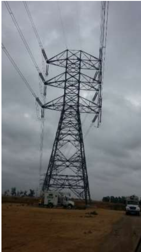
Figure 5: OPGW splicing at Tower M70-T4 (Segment 8, Phase 3) (photo courtesy of SCE).
