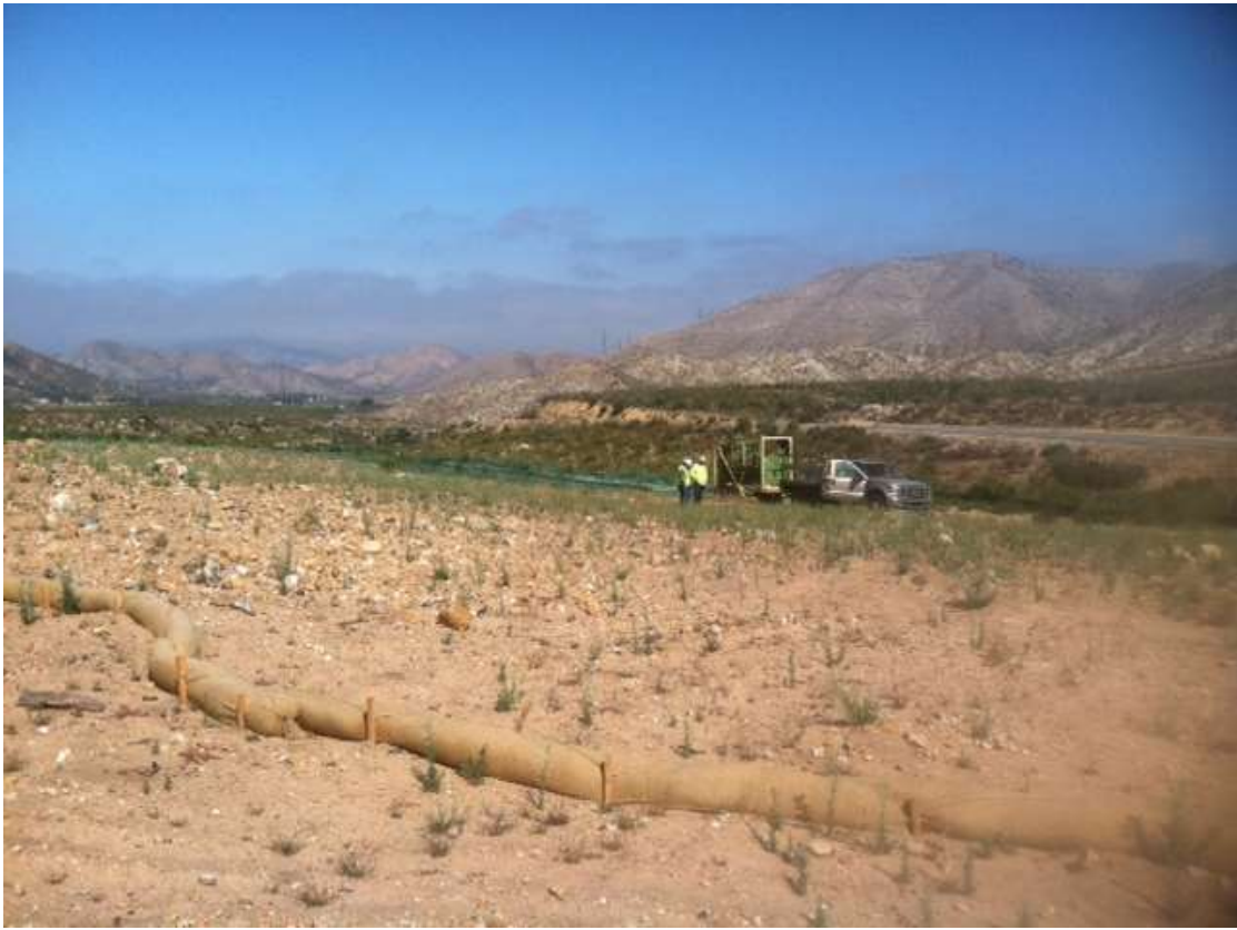
.Figure 3: Hydromulch (BMP) application at Aliso Canyon HAY for final stabilization.
