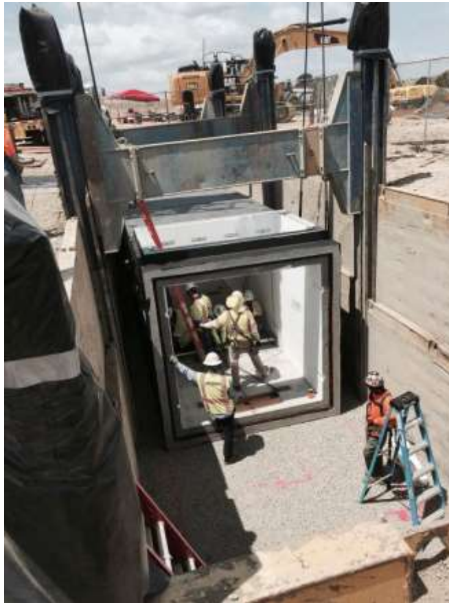
Figure 7: Installing the third splice vault at Vault Cluster #1.
