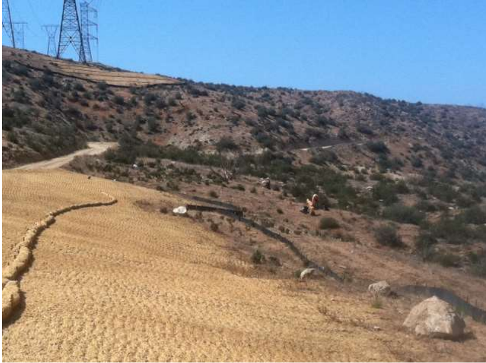
Figure 1: Hand pulling weed abatement occurring at Construct 11AXXX, Segment 11C.
