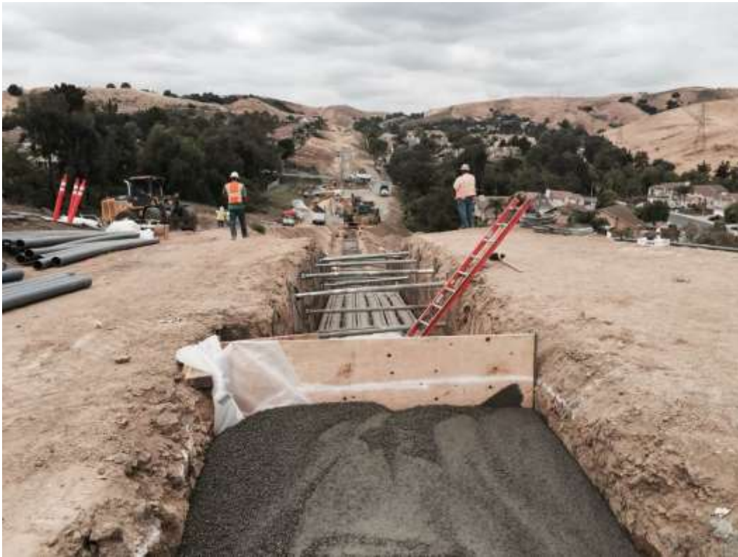
Figure 8: Conduit installation and concrete backfilling between Vault Clusters #7 and #8.
