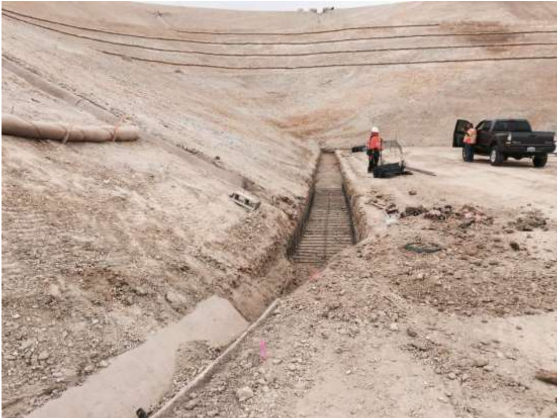
Figure 9: Terrace drain construction along the toe of the upper slope at Western Transition Station.
