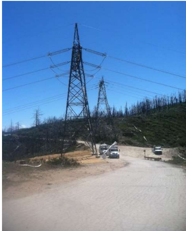
Figure 2: Wire splicing activities at Construct 33, Segment 11C.
