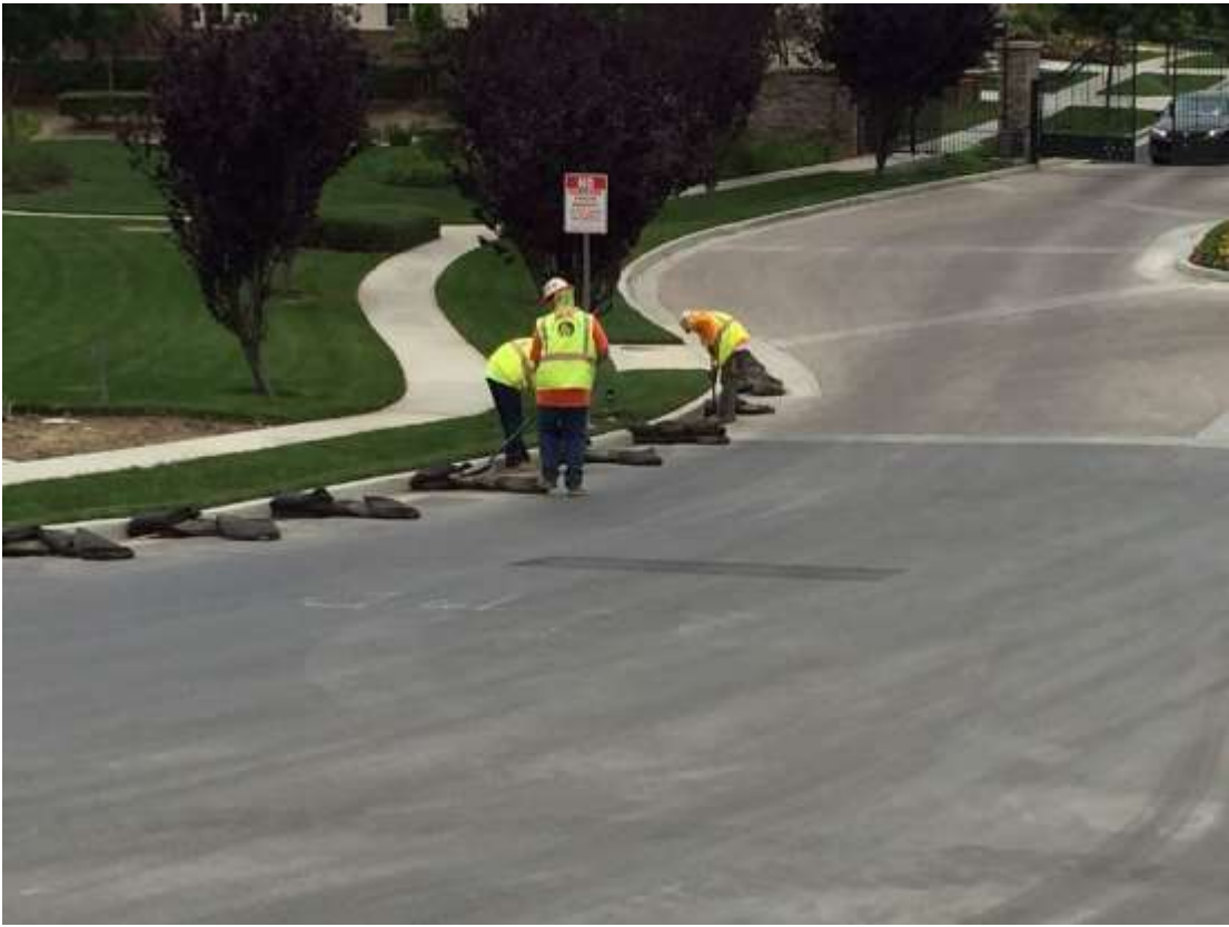
Figure 10: Crew repairing BMPs along Canon Drive.
