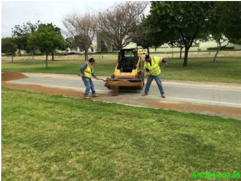
Figure 6: Installing decomposed granite along pedestrian walkway in Ayala Park (Segment 8, Phase 3) (photo courtesy of SCE).
