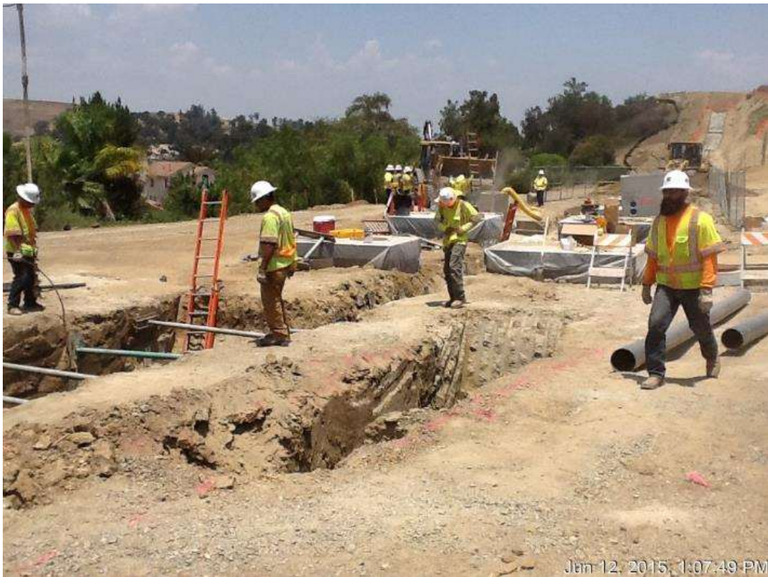
Figure 4: In and out trenching activities at VC #7, 500 kV Underground.
