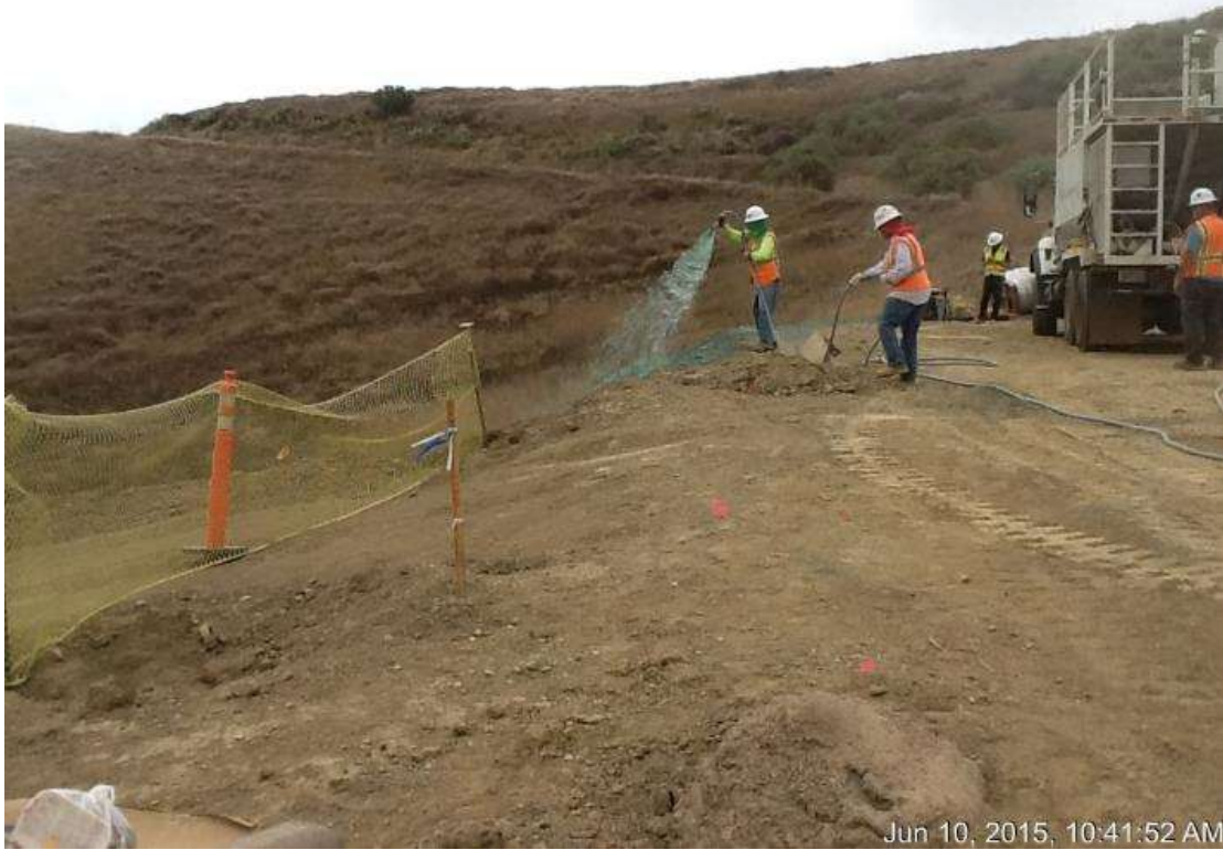
Figure 7: Hydromulch (BMP) installation at slopes at the WTS entrance and VC #1, 500 kV Underground.
