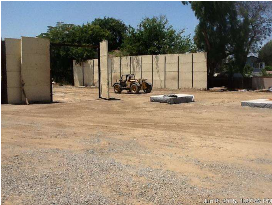
Figure 9: Relocation activities of HDD drill at VC#12, 500 kV Underground.
