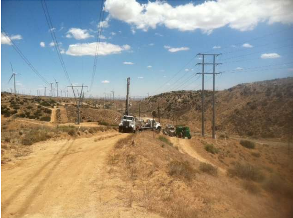
Figure 1: GR #13 excavation for cathodic protection activities, Segment 3B.
