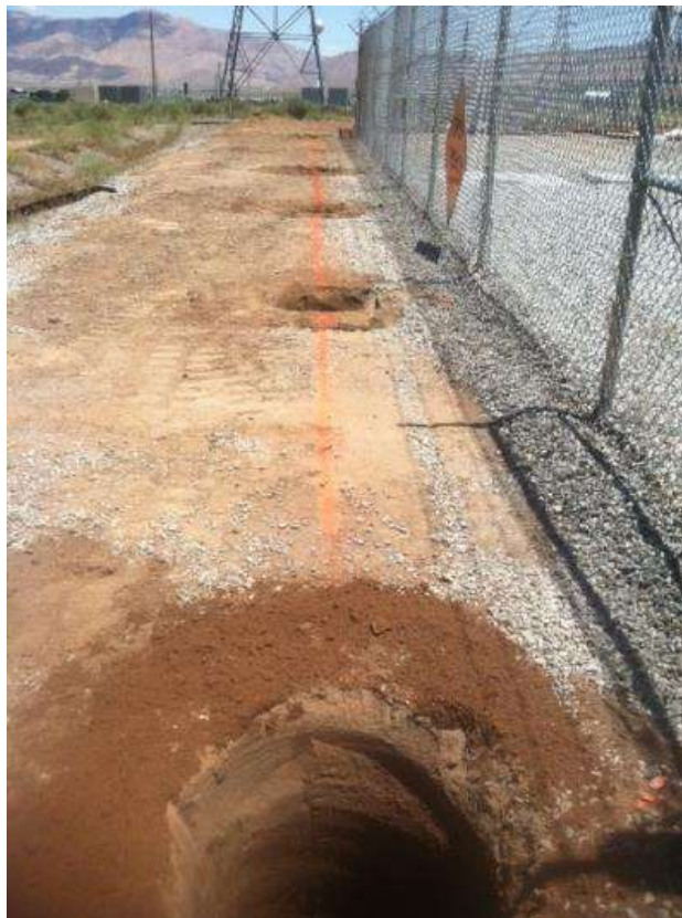
Figure 2: Excavation holes for fence posts at Highwind Substation wall.
