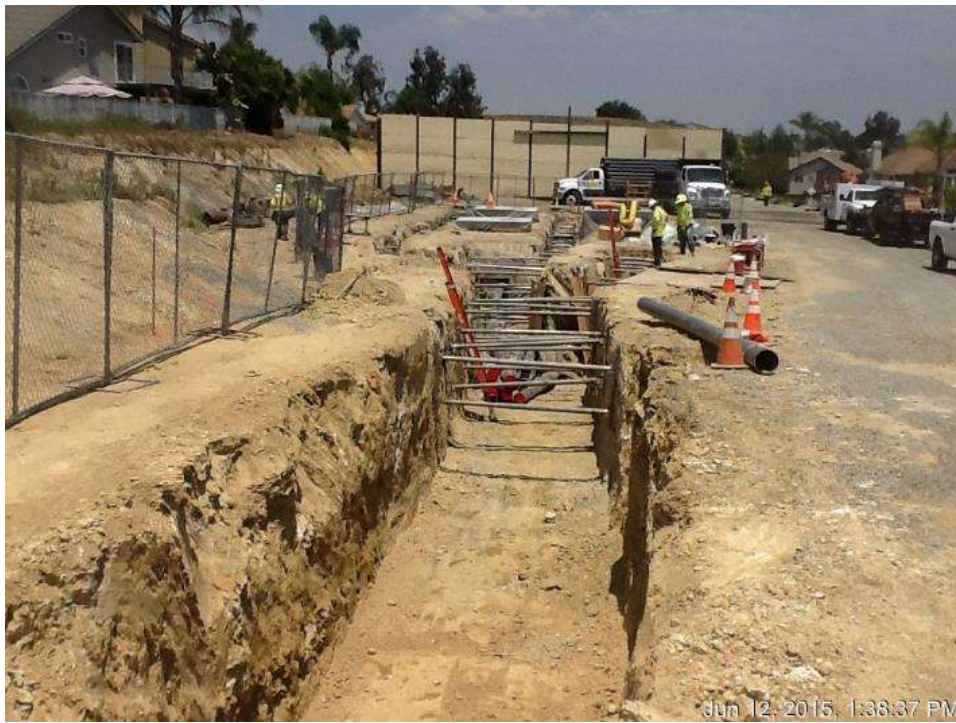
Figure 5: Trenching and conduit installation at VC #11, 500 kV Underground.
