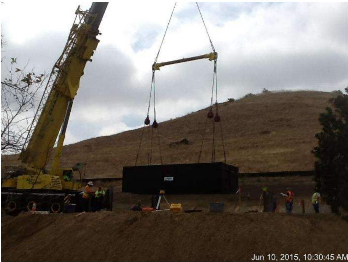
Figure 3: Installation of RV #4, 500 kV Underground.
