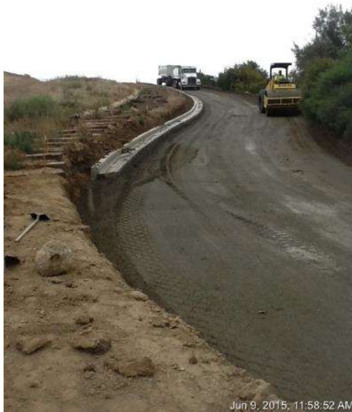
Figure 6: Class II Base installation at the WTS entrance, 500 kV underground.
