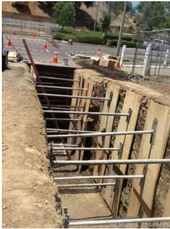
Figure 5: Trenched area between Chino Hills Parkway and VC #9 awaiting conduit placement, 500 kV Underground.
