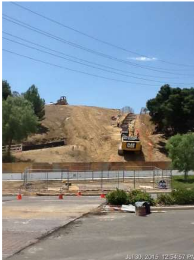
Figure 4: Trenching activities between VC #8 and Chino Hills Parkway, 500 kV Underground.
