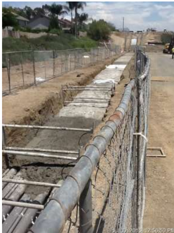
Figure 6: Conduit and concrete fill for the trenchline near Little Bend up to VC #9, 500 kV Underground.
