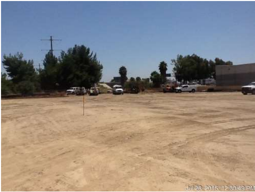
Figure 3: Site preparation for foundations at the WTS, 500 kV Underground.
