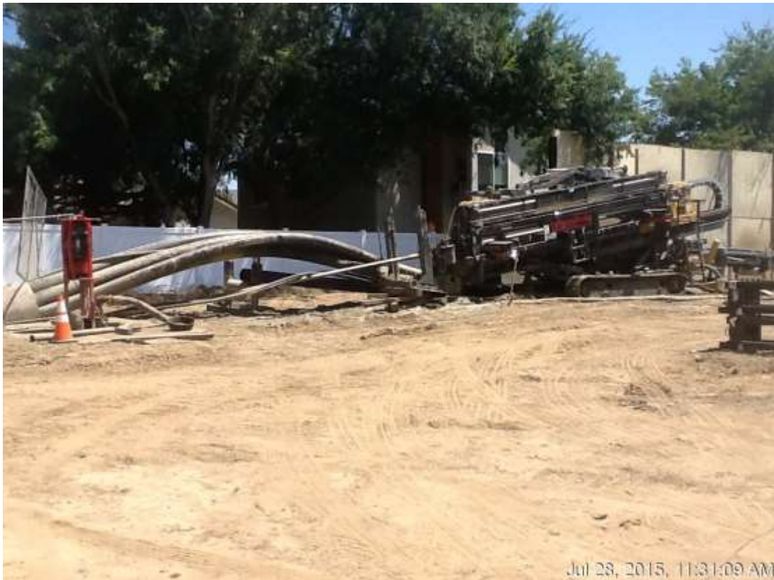
Figure 7: Conduit recovery at VC #12, 500 kV Underground.
