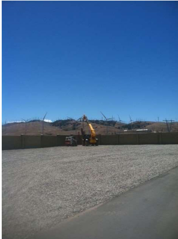
Figure 2: Wall panel capping activities occurring at Highwind Substation.
