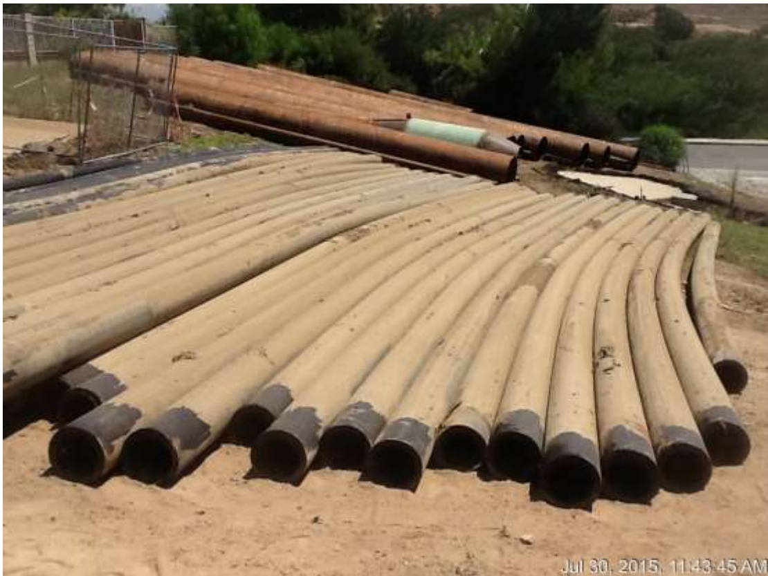
Figure 8: Conduit cut into 40-foot lengths and casing at VC #11, 500 kV Underground.
