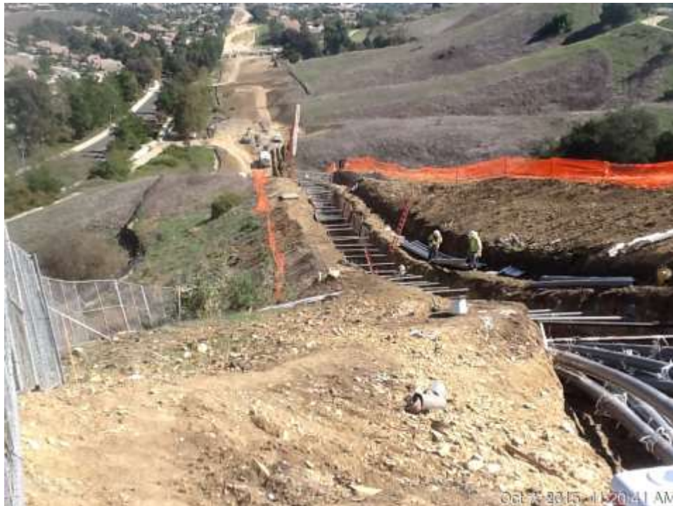
Figure 6: Conduit installation between V #3 and VC #4, 500 kV Underground.
