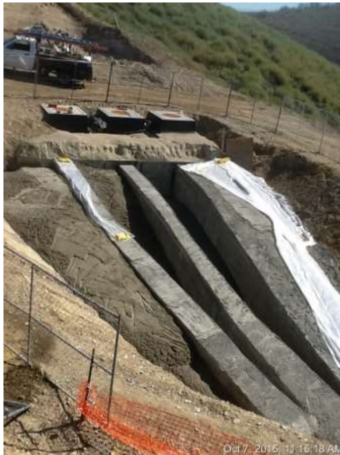
Figure 5: RV #2 in/out concrete placement activities, 500 kV Underground.
