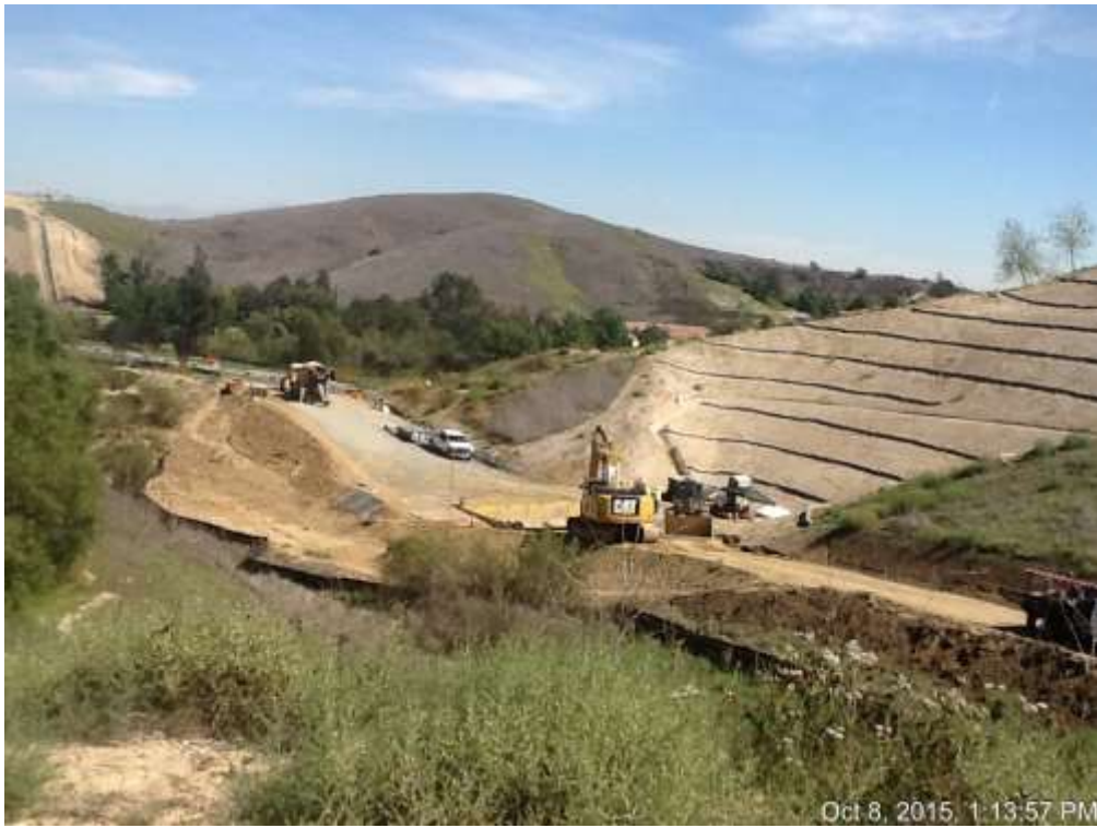
Figure 3: Vault installation at RV #1, 500 kV Underground.
