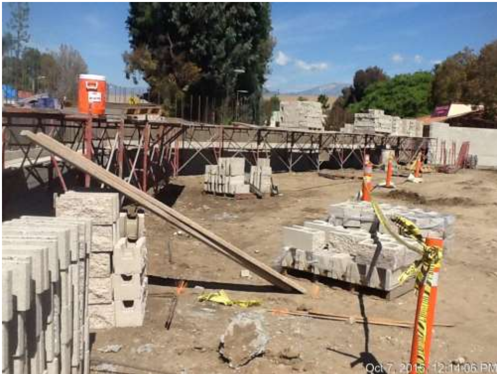
Figure 2: ETS wall construction, 500 kV Underground.
