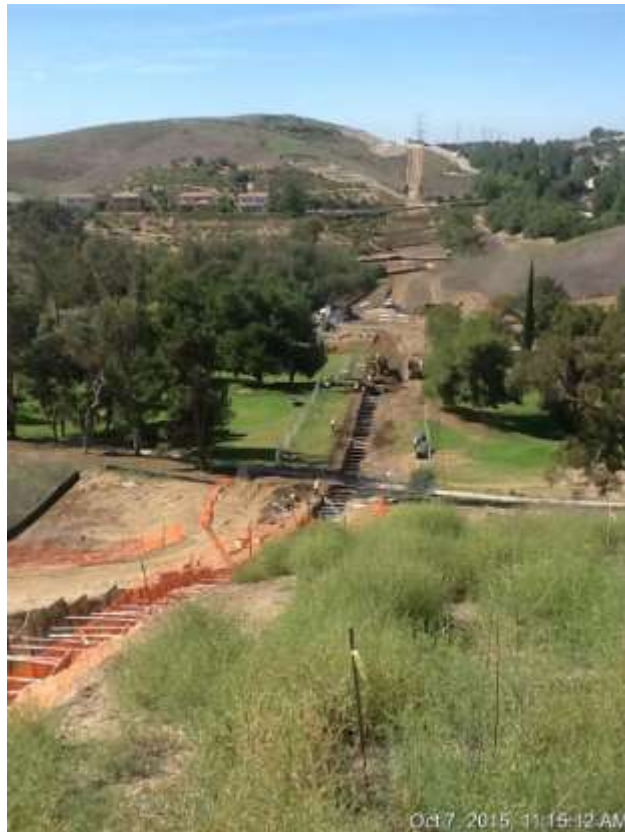
Figure 4: Conduit installation activities RV #2 towards VC #2 through the golf course area within the 500 kV Underground.
