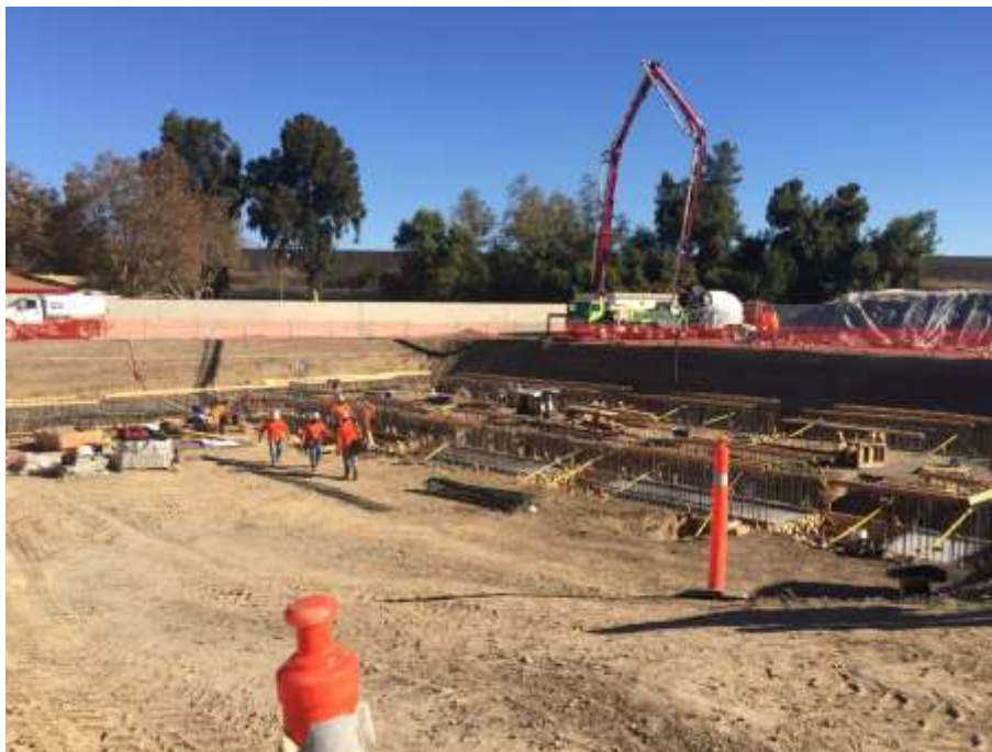
Figure 4: Foundation work at the ETS, 500 kV Underground.
