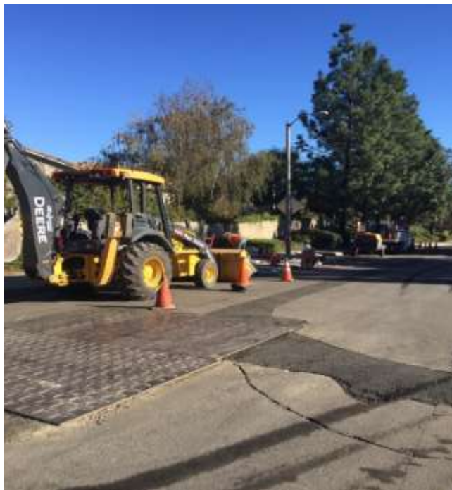
Figure 2: Telecom installation along Eucalyptus Avenue, Chino Hills, 500 kV Underground.
