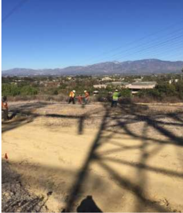
Figure 1: Installation of irrigation system at Tower M41-T4, in preparation for container plant installation on Segment 7.
