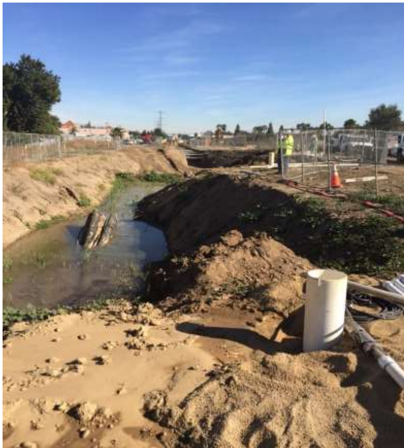
Figure 3: Well installation near the VC #14 tie-in. Six wells were installed in order to dewater the trench and allow crews to complete the tie-in between the HDD conduit and VC #14, 500 kV Underground.
