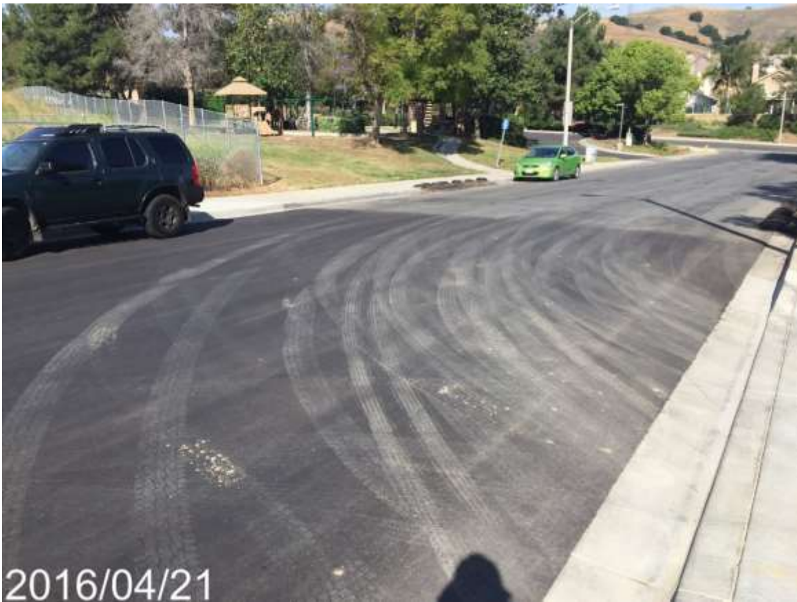
Figure 3: Trackout was reported in several locations along the 500 kV Underground right-of-way. Photo courtesy of SCE.
