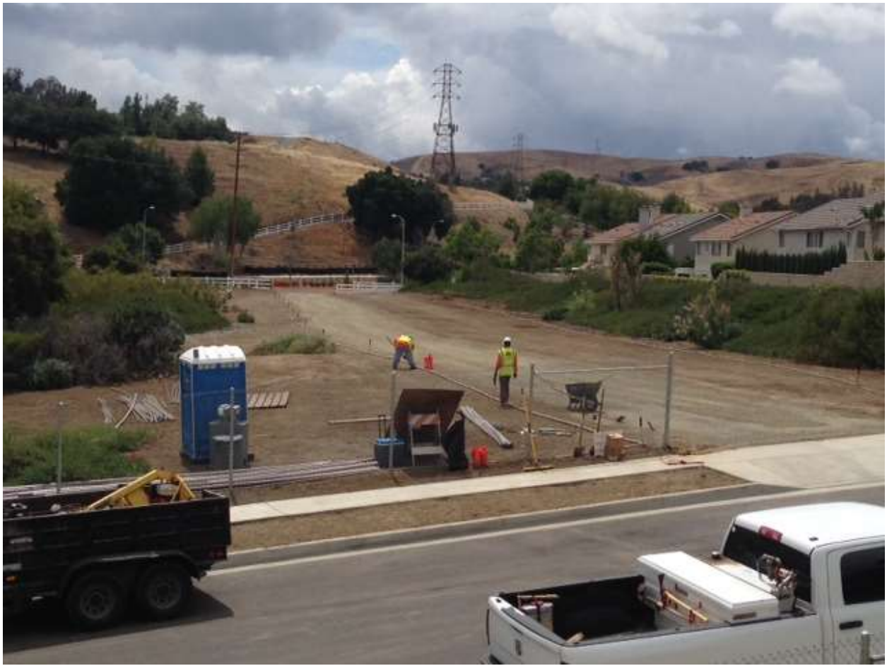
Figure 3: Landscaping crews conducted irrigation repair near VC #9. Photo courtesy of SCE.
