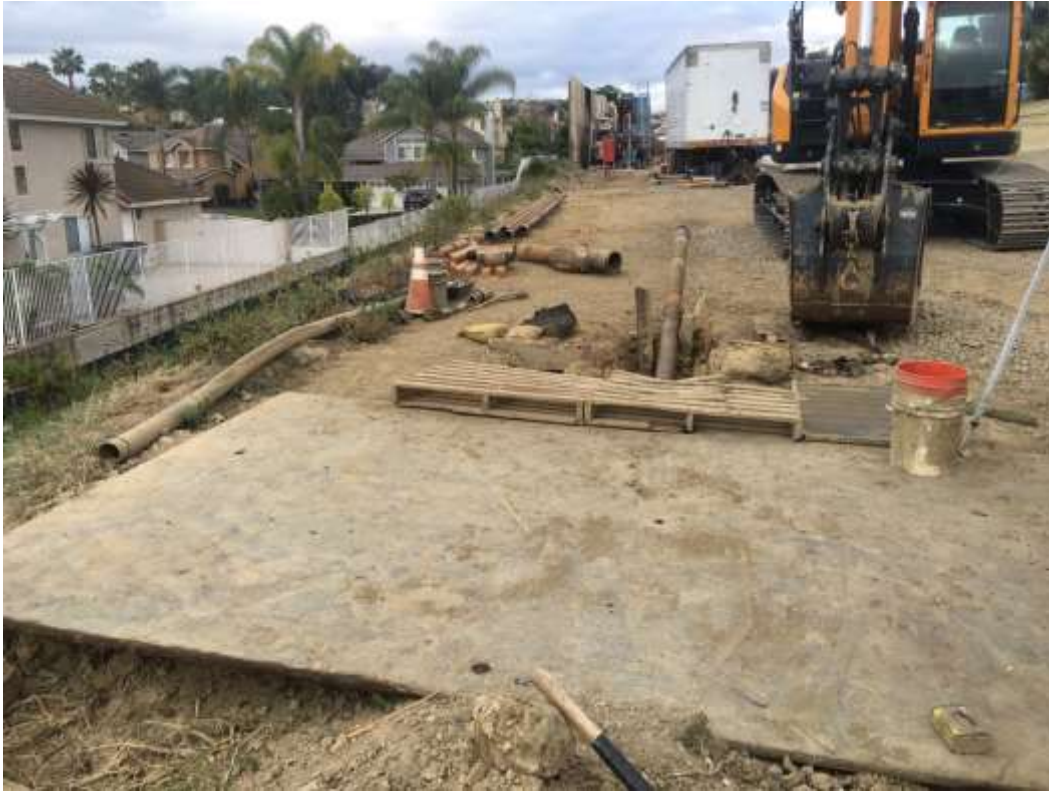
Figure 1: The pilot drill at the 6th and final HDD long-bore site was completed during the subject week. Photo courtesy of SCE.
