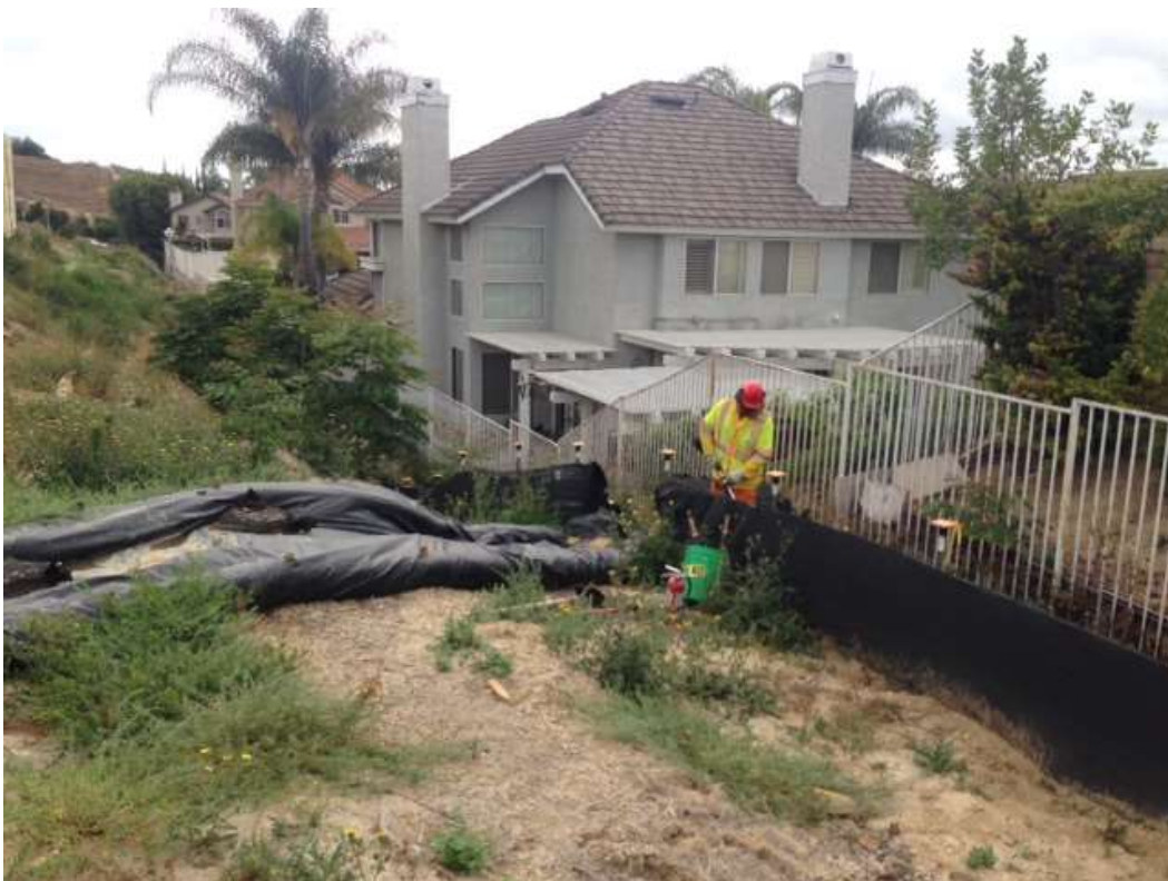
Figure 2: Vegetation removal near VC #7. Photo courtesy of SCE.
