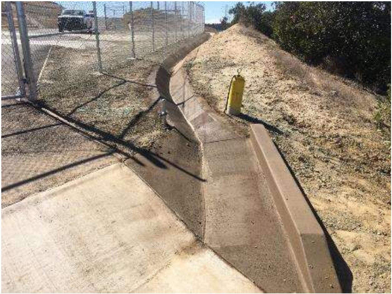
Figure 5: Concrete v-ditch placement near VC #1, 500 kV Underground. (Photo courtesy of SCE.)
