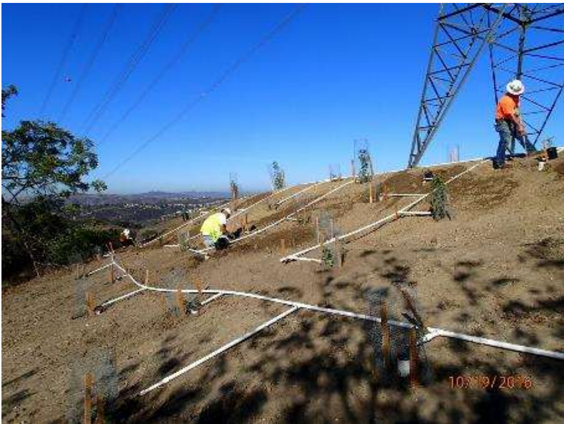
Figure 4: Container planting at Restoration Site 21, Segment 8. (Photo courtesy of SCE.)
