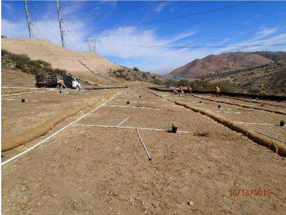
Figure 1: Irrigation installation and testing at Restoration Site 21, Segment 11. (Photo courtesy of SCE.)
