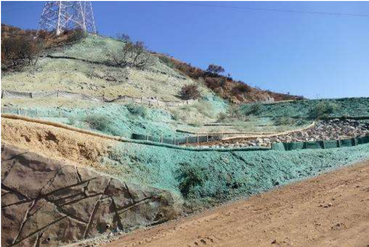
Figure 3: Hydroseeding after BMP repairs at Tower M27-T3 near Duarte, Segment 7. (Photo courtesy of SCE.)
