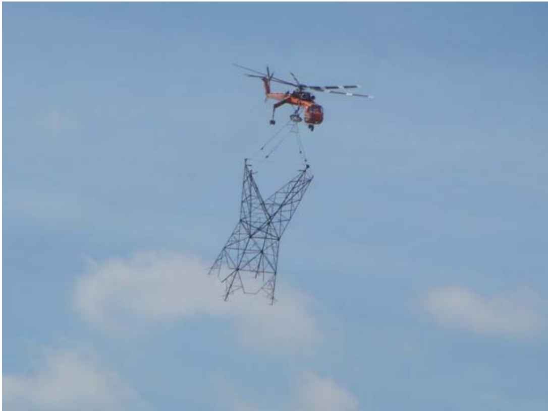
Figure 2: Skycrane lifting tower sections into place on the ANF.
