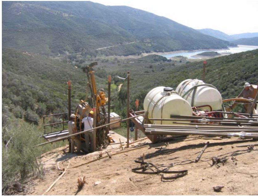
Figure 1: Micropiling operations at Tower 77 on the ANF.
