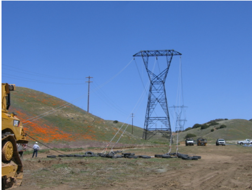
Figure 4: Stringing activity in Section 3, Segment 1.
