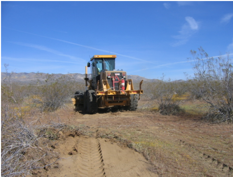
Figure 6: Crush clearing at Tower 24 in Segment 3A.
