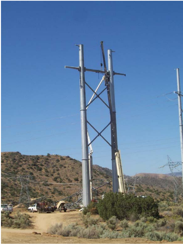
Figure 2: Sagebrush Transmission Line Modification, Segment 2, by the Vincent Substation.
