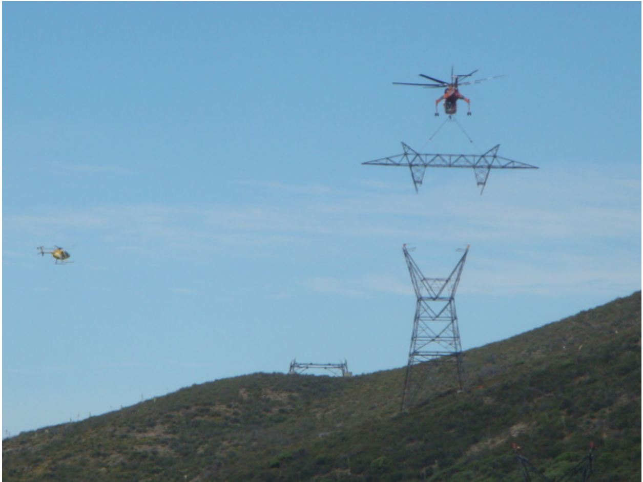
Figure 1: Tower assembly on the ANF using the Ericsson Sky Crane, Segment 1, Section 2.
