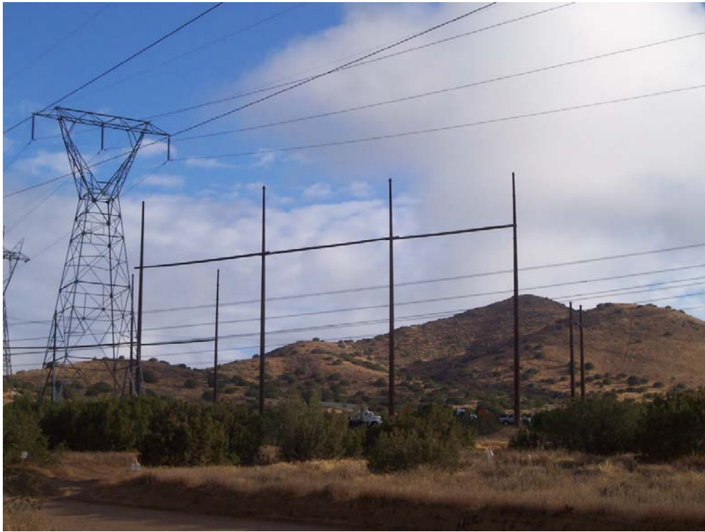
Figure 3: Guard pole structure between Towers 106 and 107, Segment 2.
