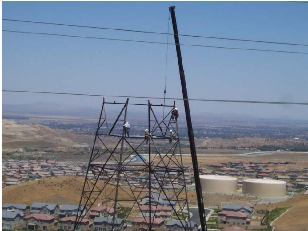
**Figure 2:** Assembly of lattice steel tower at Structure 80, Segment 2.
