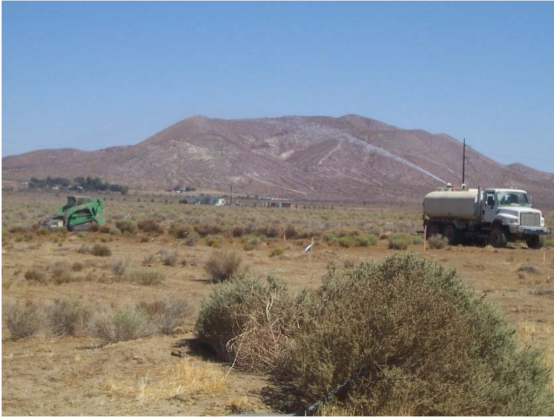
Figure 3: Vegetation removal Tower 52 Segment 3A.
