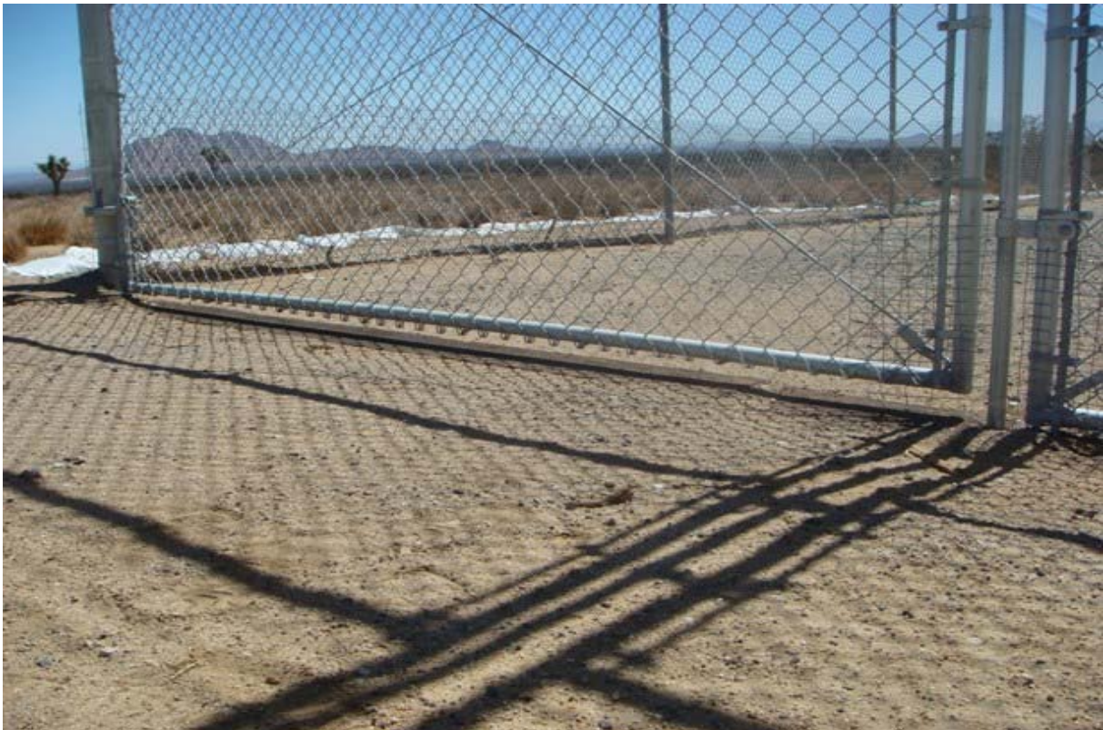
Figure 4: Gap under the fence on the east side of the Windhub Substation.
