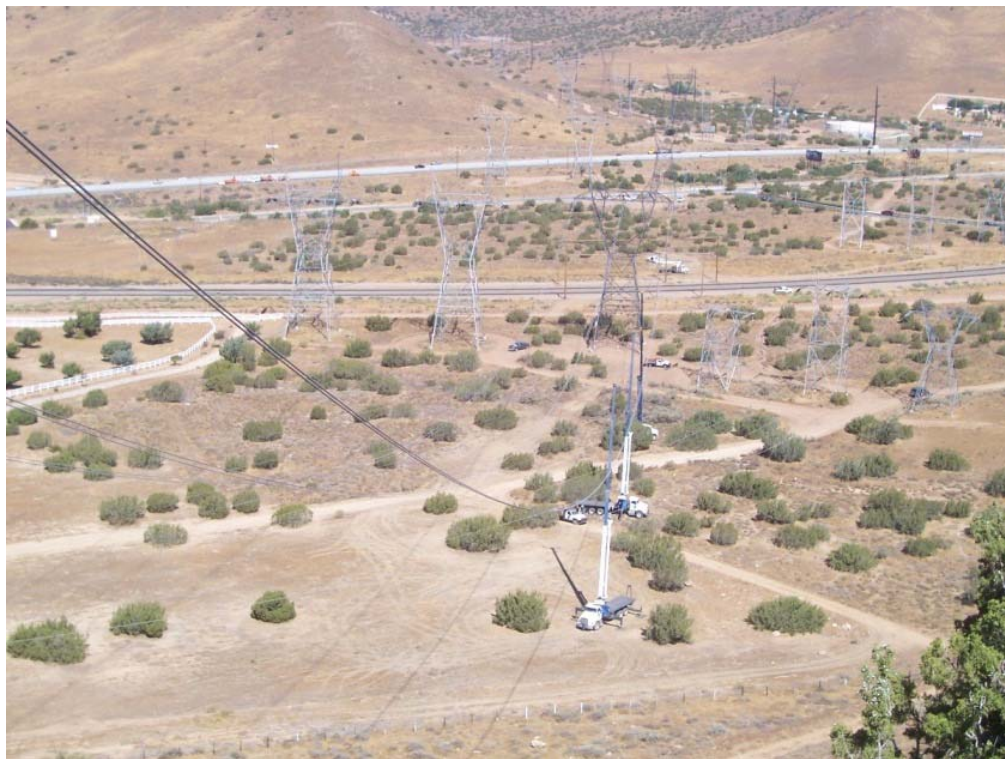
Figure 2: Wire stringing between Towers 113-115 Segment 2.
