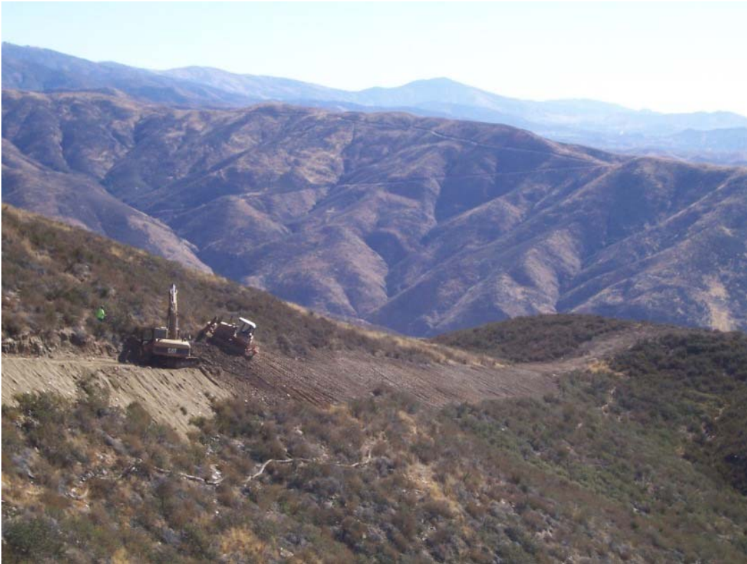
Figure 1: Road SR41 restoration on the ANF.
