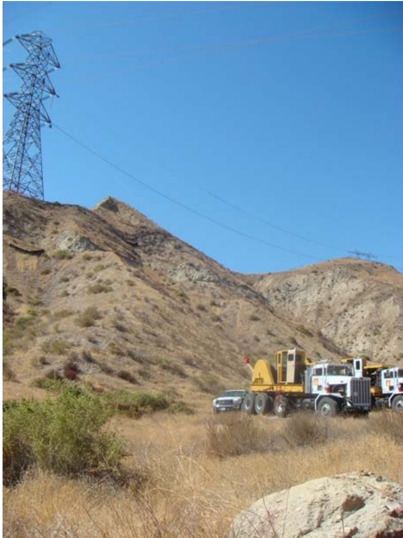
Figure 1: Stringing operations in Segment 1, between Towers 25 and 26C.
