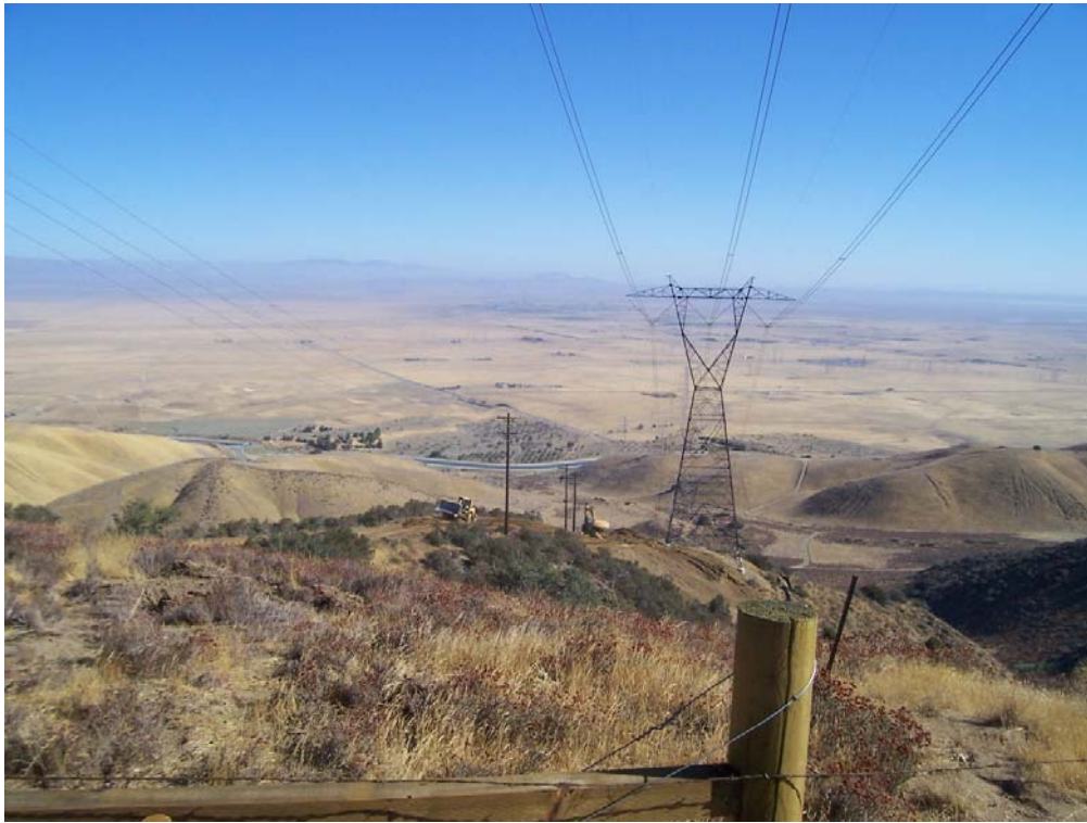
Figure 2: Access road and pad restoration Segment 1, Section 3, Tower 99.
