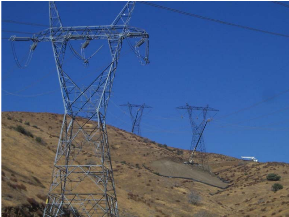
Figure 3: Segment 2 wire stringing at Tower 76.
