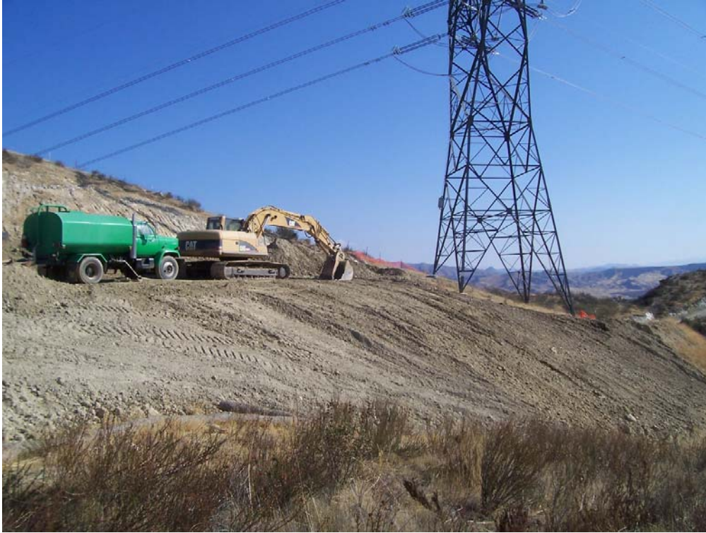
Figure 1: Final road recontouring at Towers 26 A-C, Section 1.
