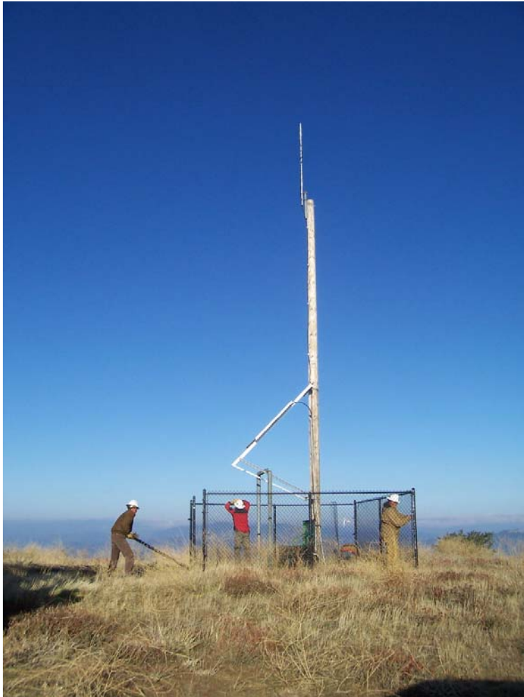
Figure 2: Removal of the Sierra Pelona radio repeater on the ANF.
