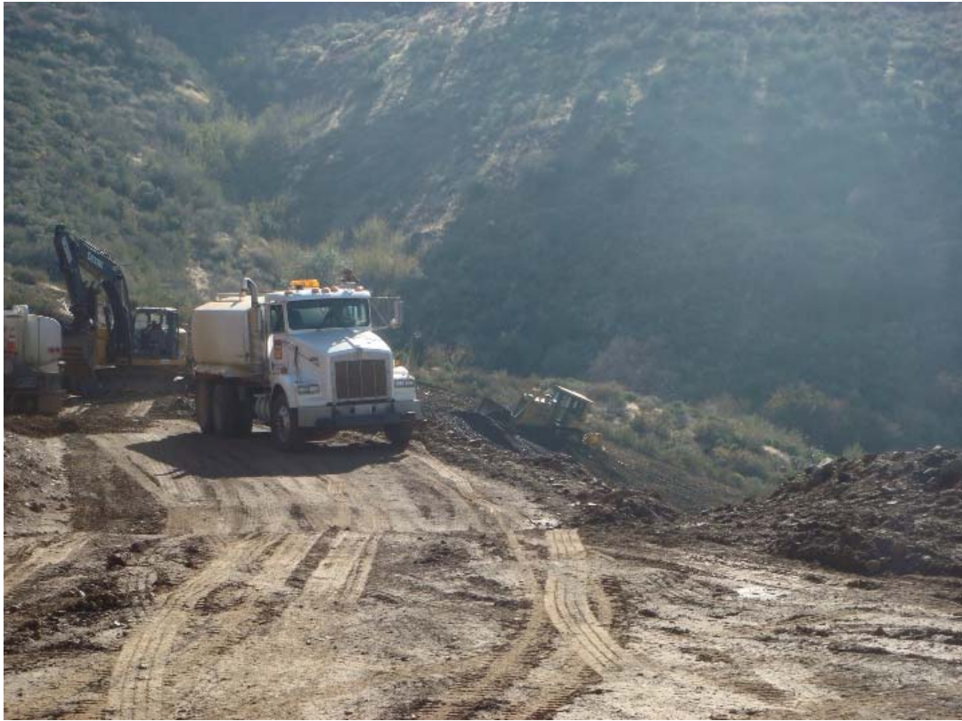
Figure 3: Road recontouring near Tower 43, Segment 2.
