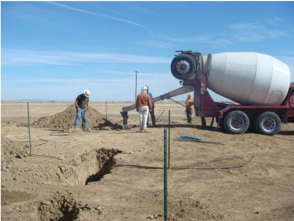
Figure 4: Installation of concrete snubs for wire stringing near Tower 71, Segment 3A.
