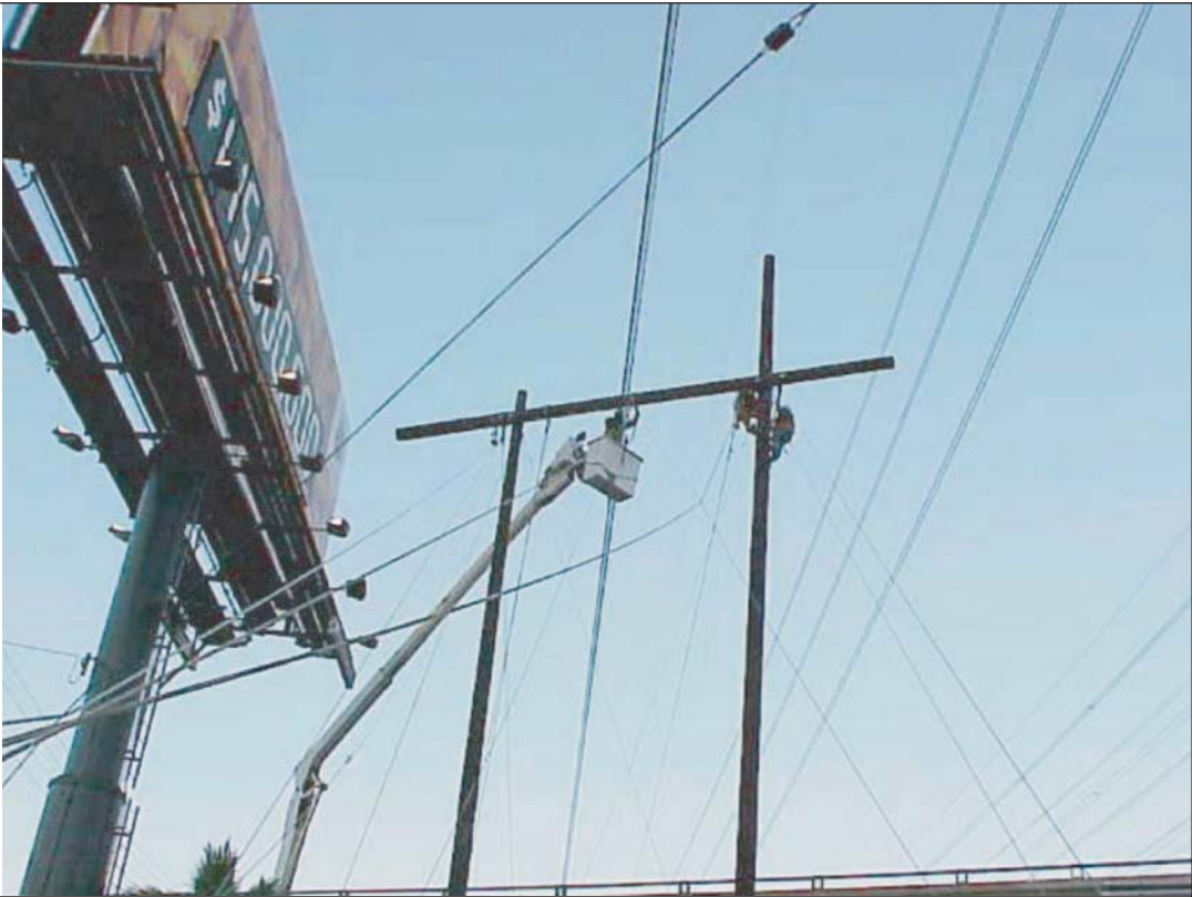
Low Voltage or Street Under-Crossing (H-Frame Configuration)
