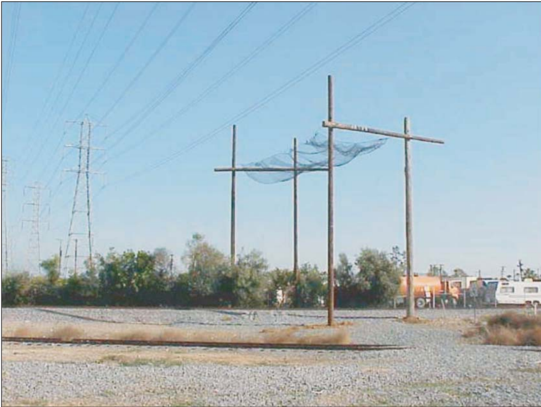
Railroad Under-Crossing (H-Frame Configuration with Net)
