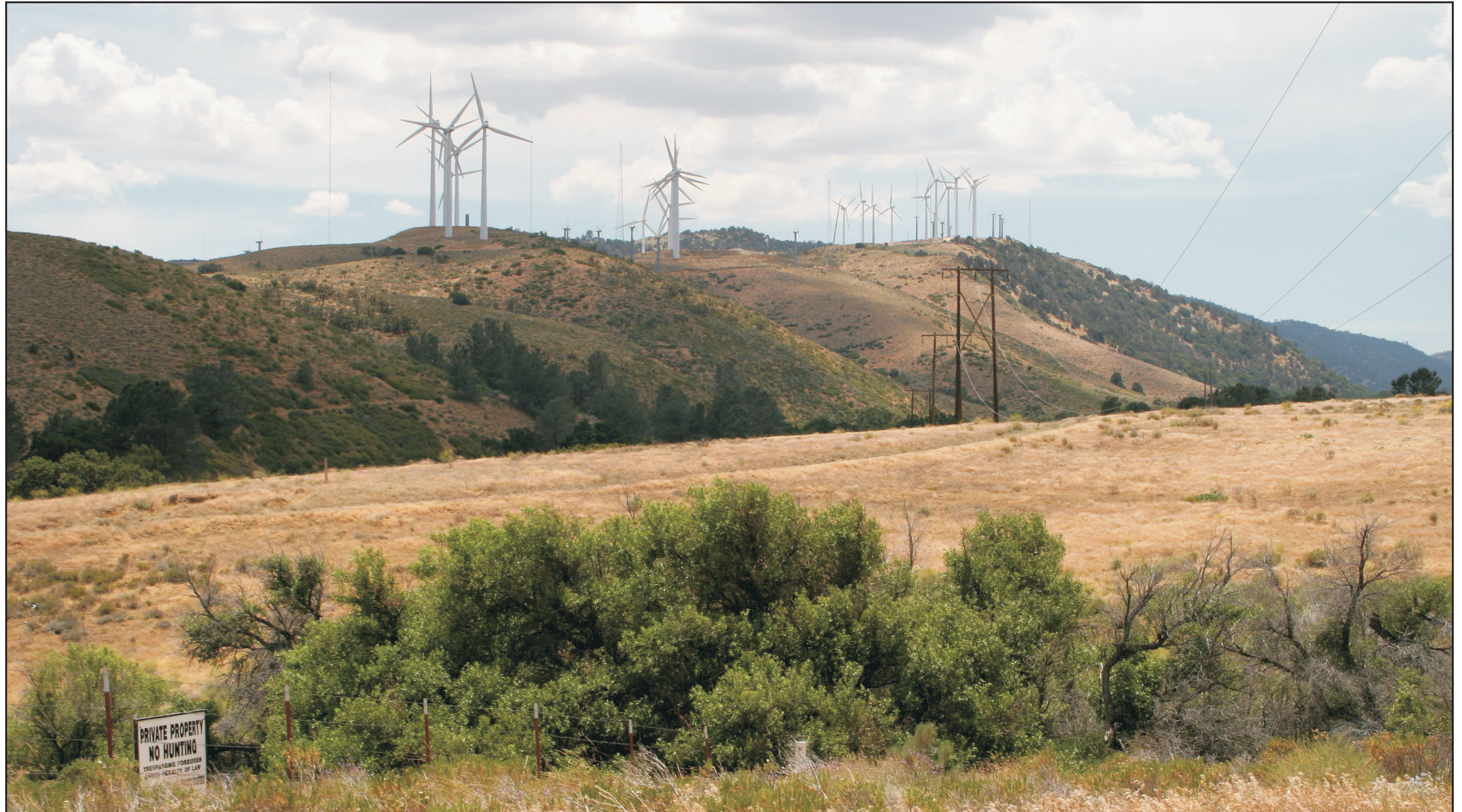
Figure C.11-3A Existing Visual Condition as seen from KOP 2
