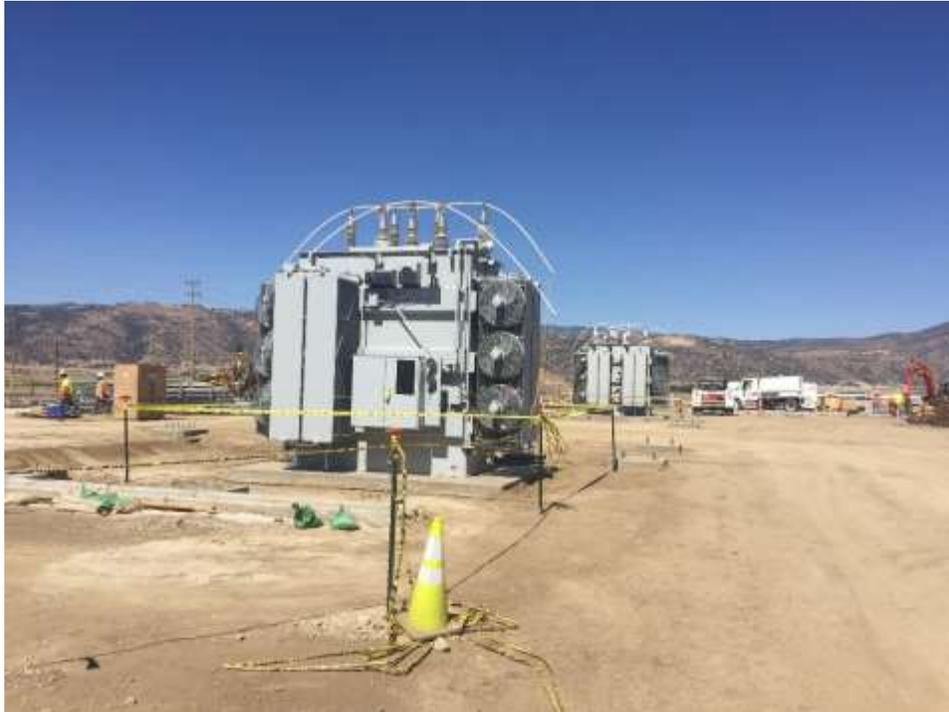
Figure 1 – Construction crews delivered and installed two transformers to the Banducci Substation site.
