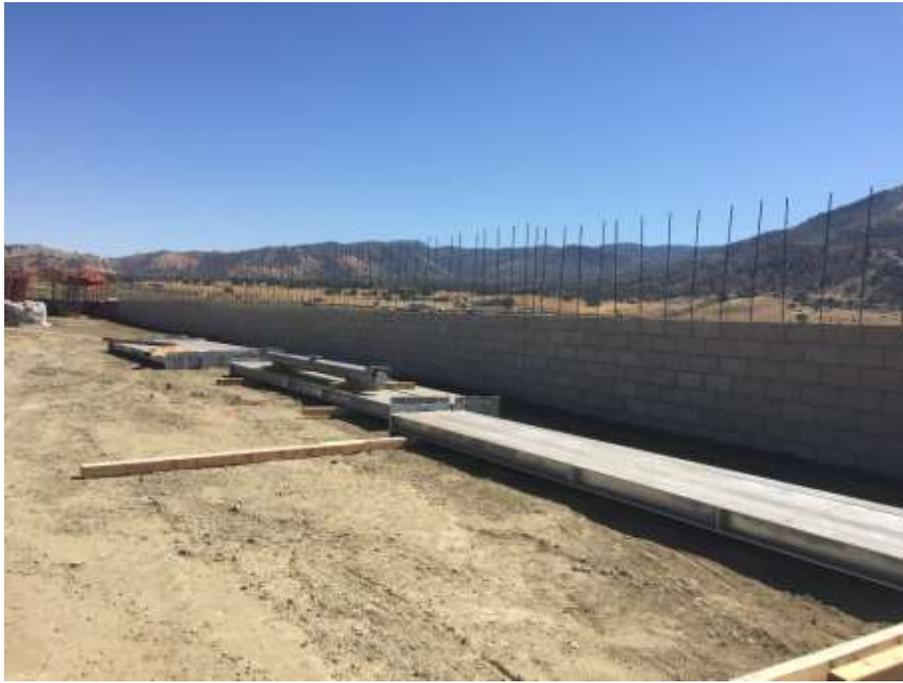
Figure 3 – Block wall installation surrounding the Banducci Substation.
