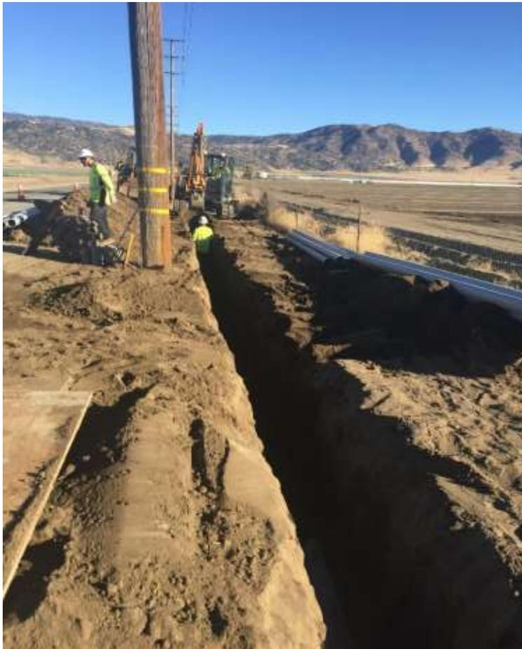
Figure 4 – Conduit installation along Pellisier Road outside of the Banducci Substation.
