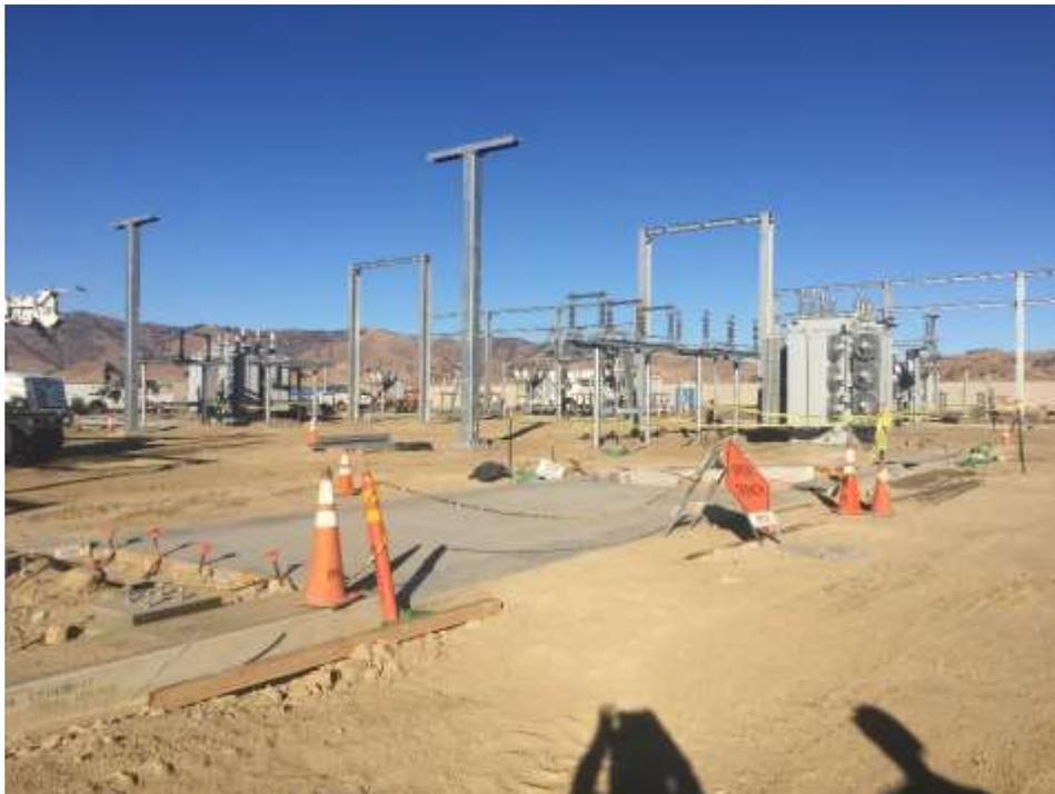
Figure 2 – Vertical steel infrastructure was erected at the Banducci Substation once foundations were completed.
