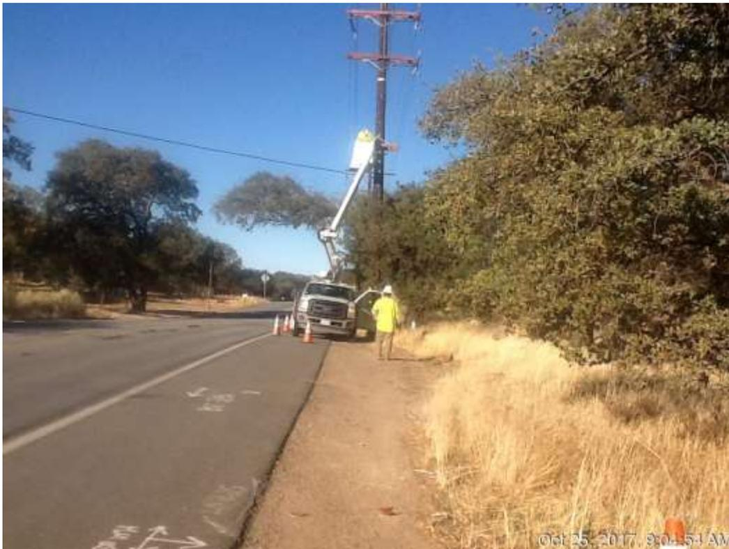
Figure 5 – Telecom installation on existing overhead wood poles took place along Highline Road near the Cummings Substation.
